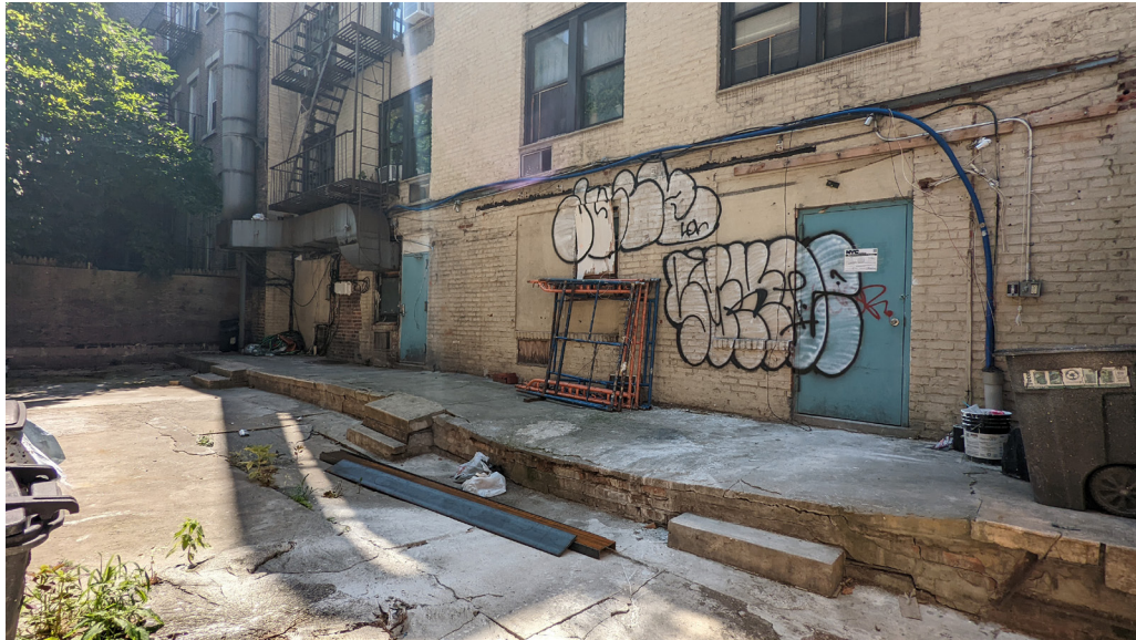
EXISTING LOOKING WEST
