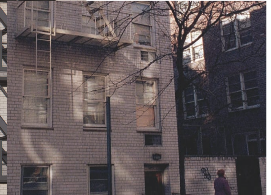
OLD SIDE YARD FACADE WITH 1-STORY BRICK WALL
