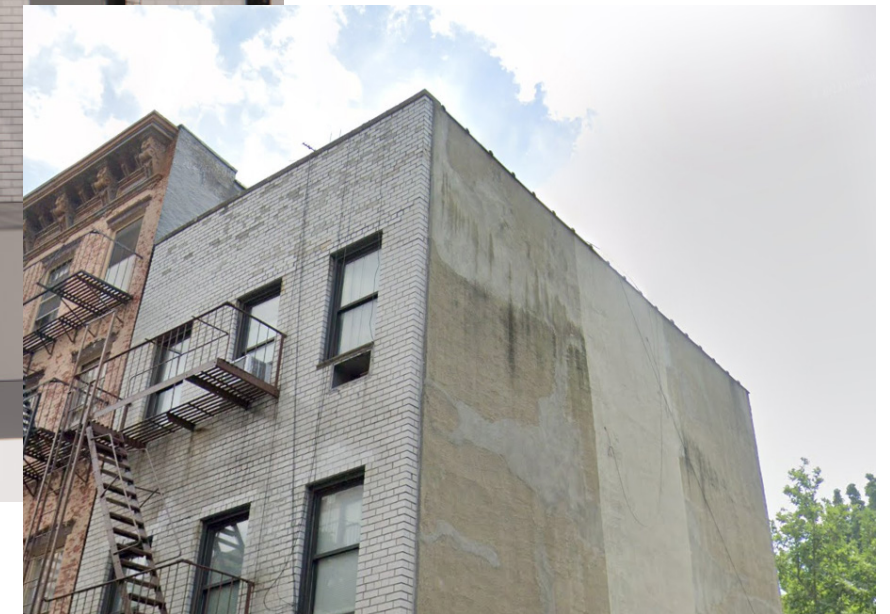
EXISTING FACADE WITH STONE CAP
