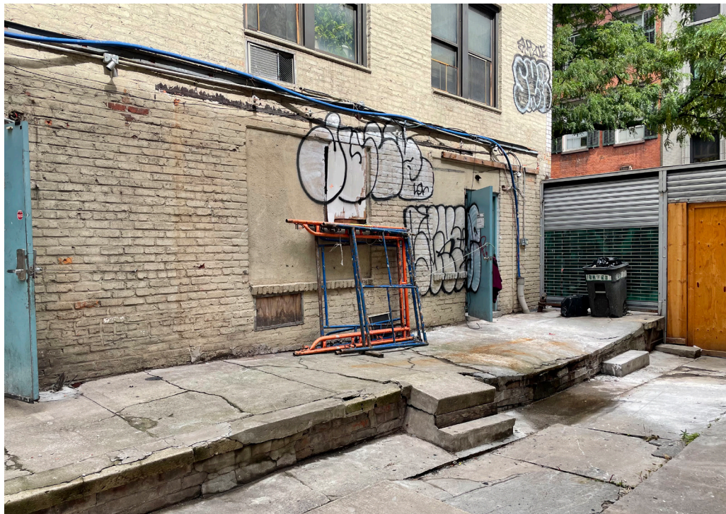
EXISTING LOOKING WEST
