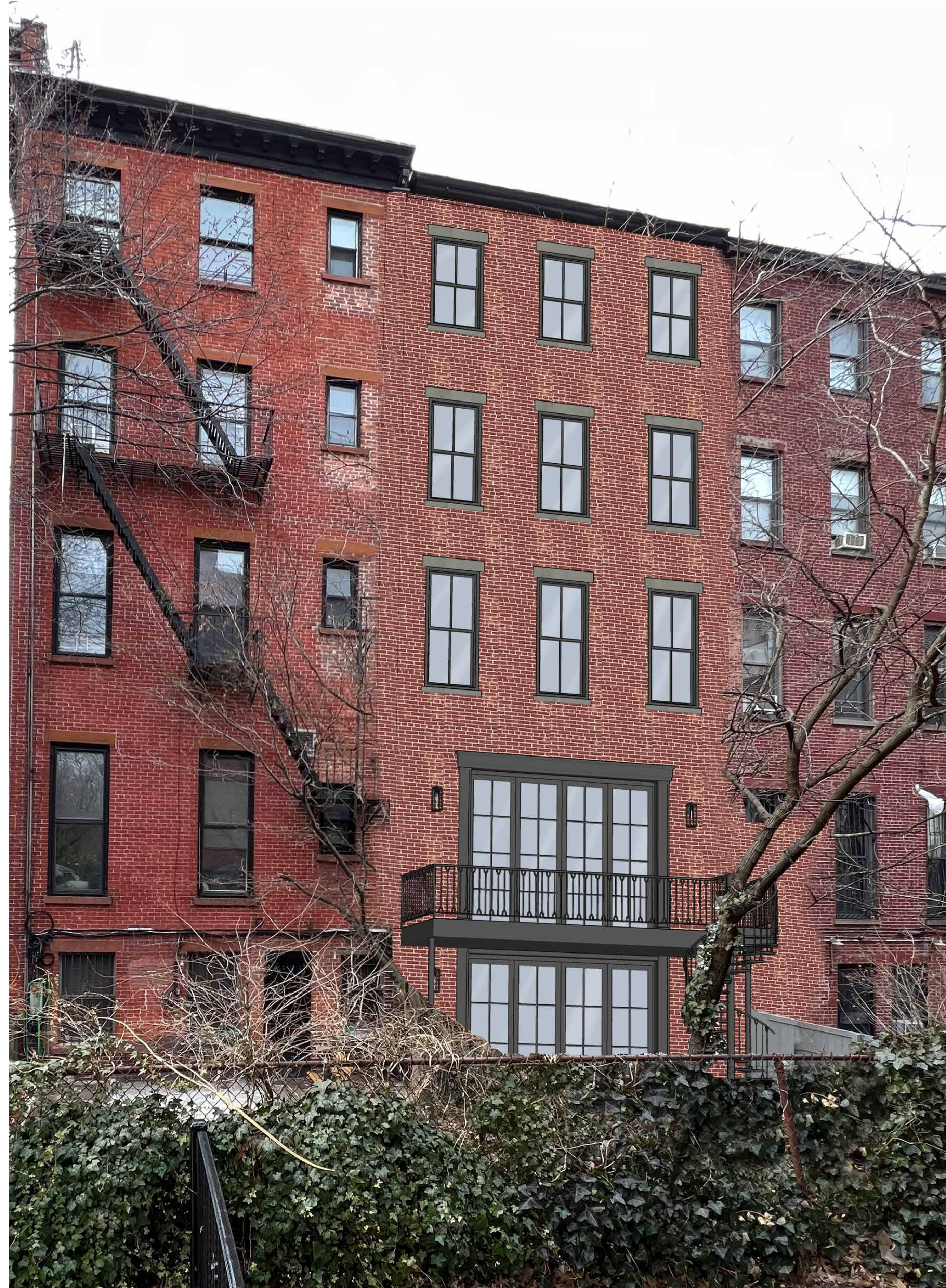
2 VIEW FROM PRIVATE DRIVEWAY - LOOKING WEST
