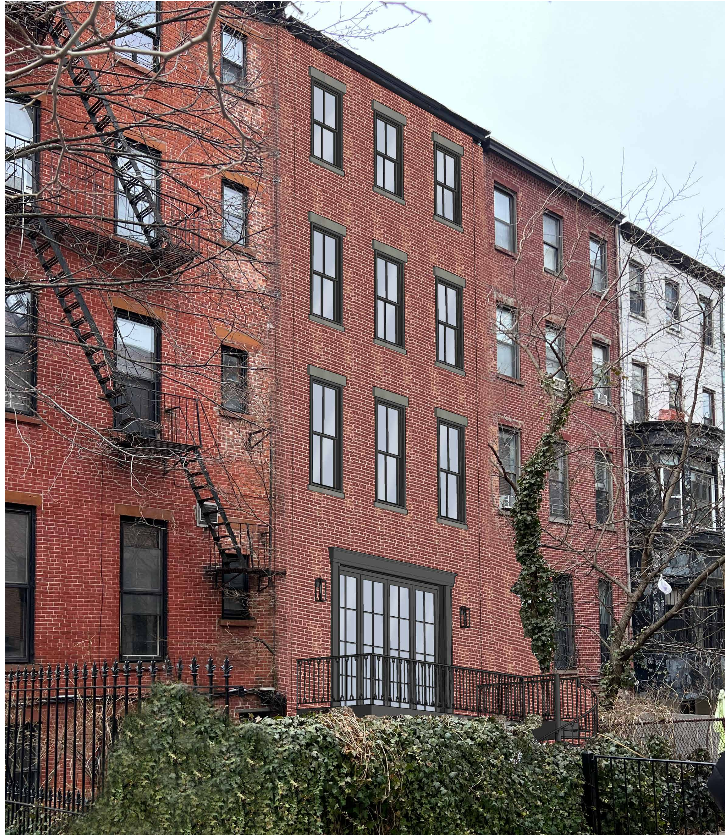
1 VIEW FROM PUBLIC SIDEWALK - LOOKING NORTHWEST
