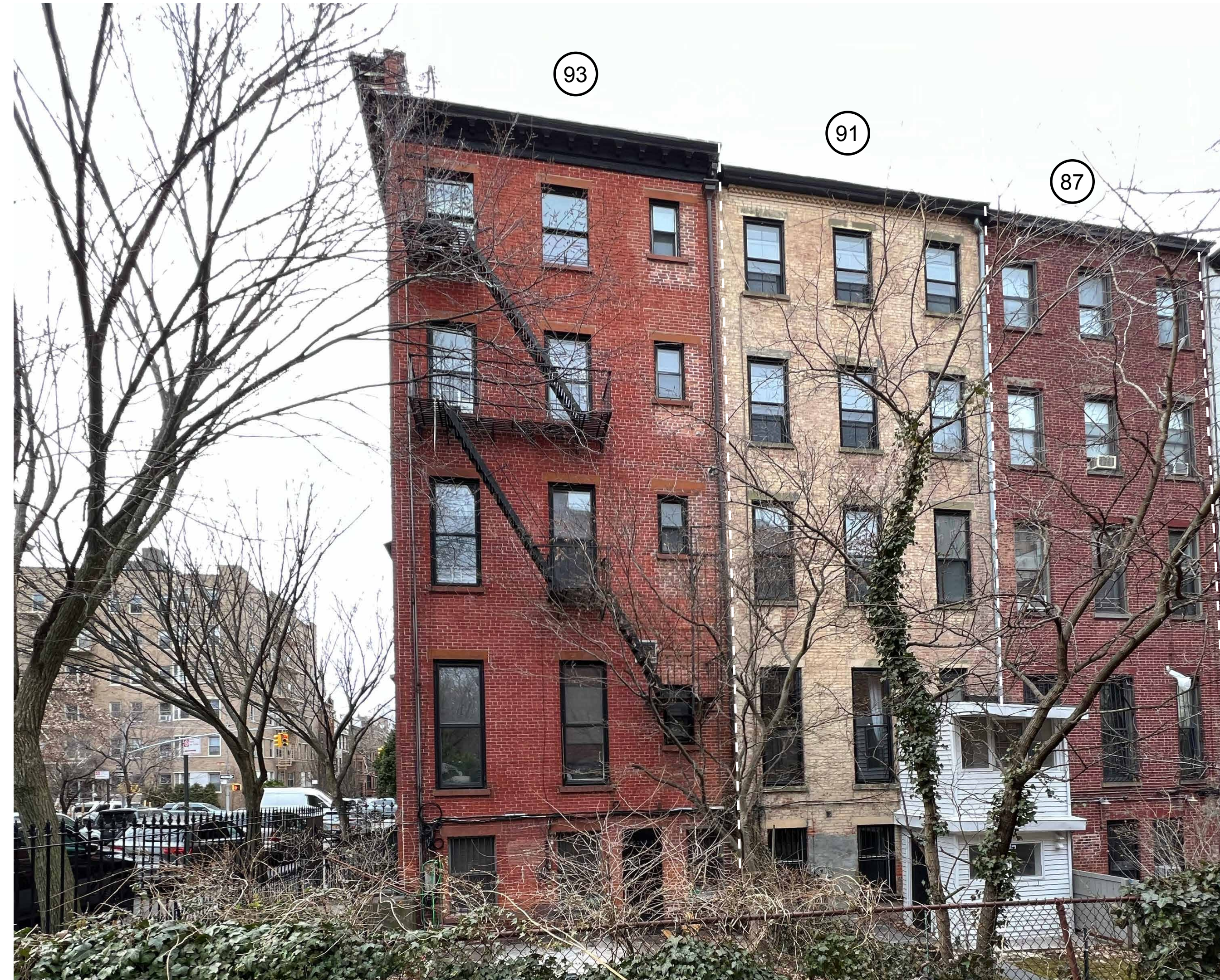
D ALLEY VIEW FROM PRESIDENT STREET ALLEY -- LOOKING NORTH
