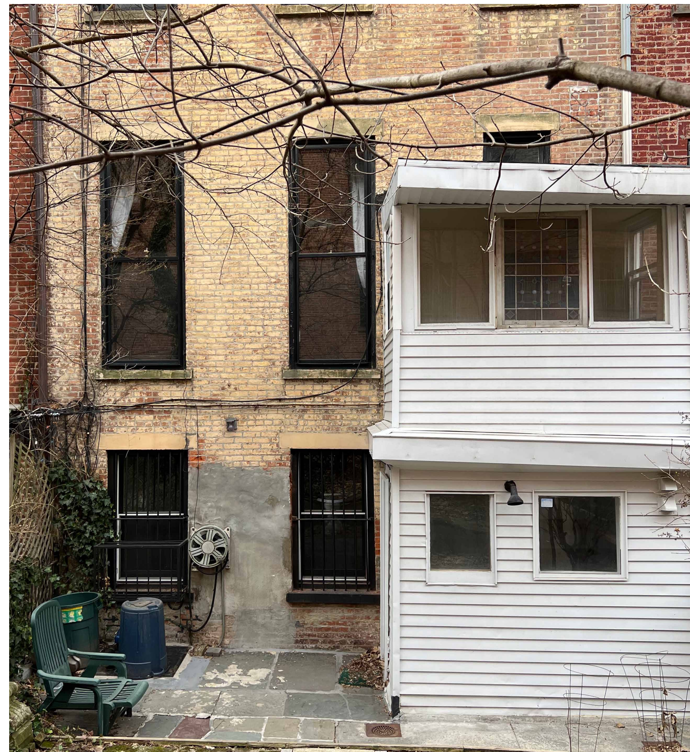
G VIEW FROM REAR YARD -- LOOKING WEST
