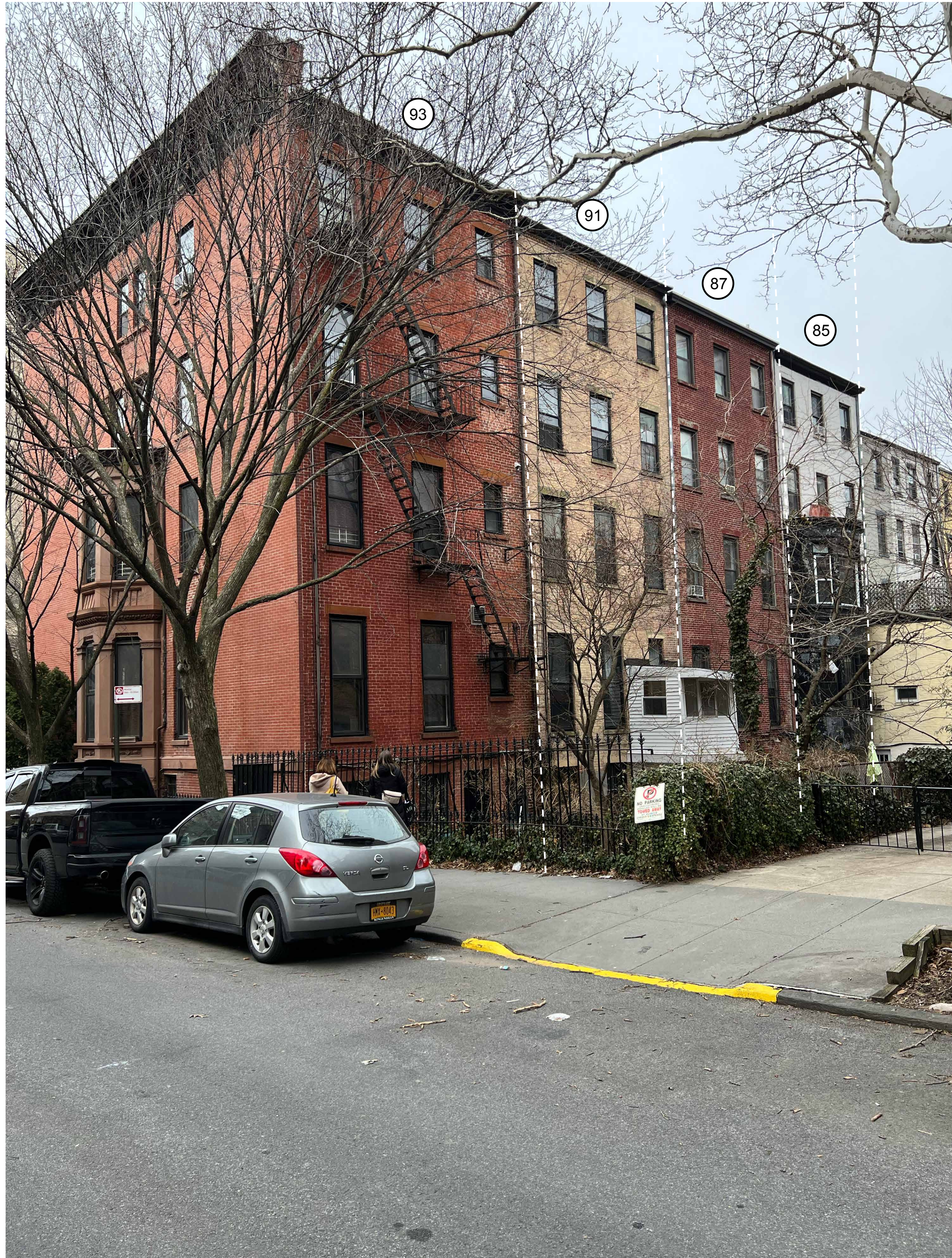
C STREET VIEW FROM PRESIDENT STREET -- LOOKING NORTH
