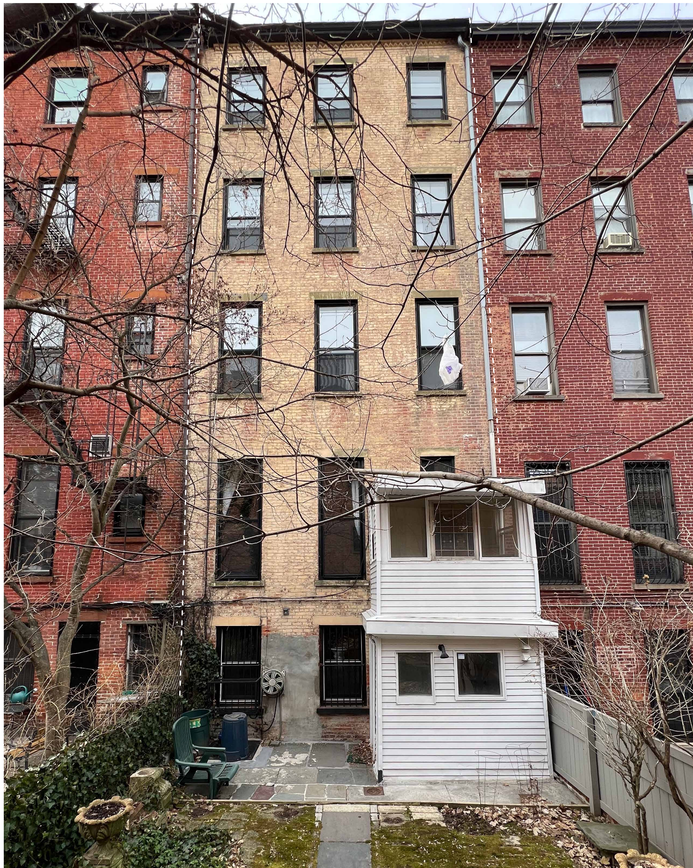
F VIEW FROM REAR YARD -- LOOKING WEST
