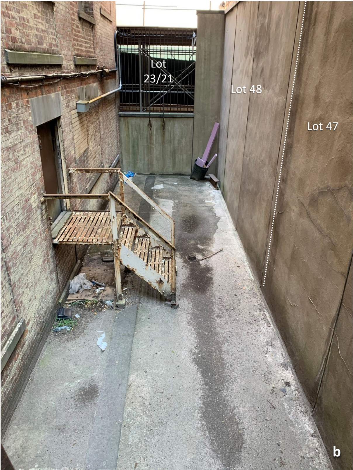
Current photo of rear yard, from neighbor to east (Lot 27)
