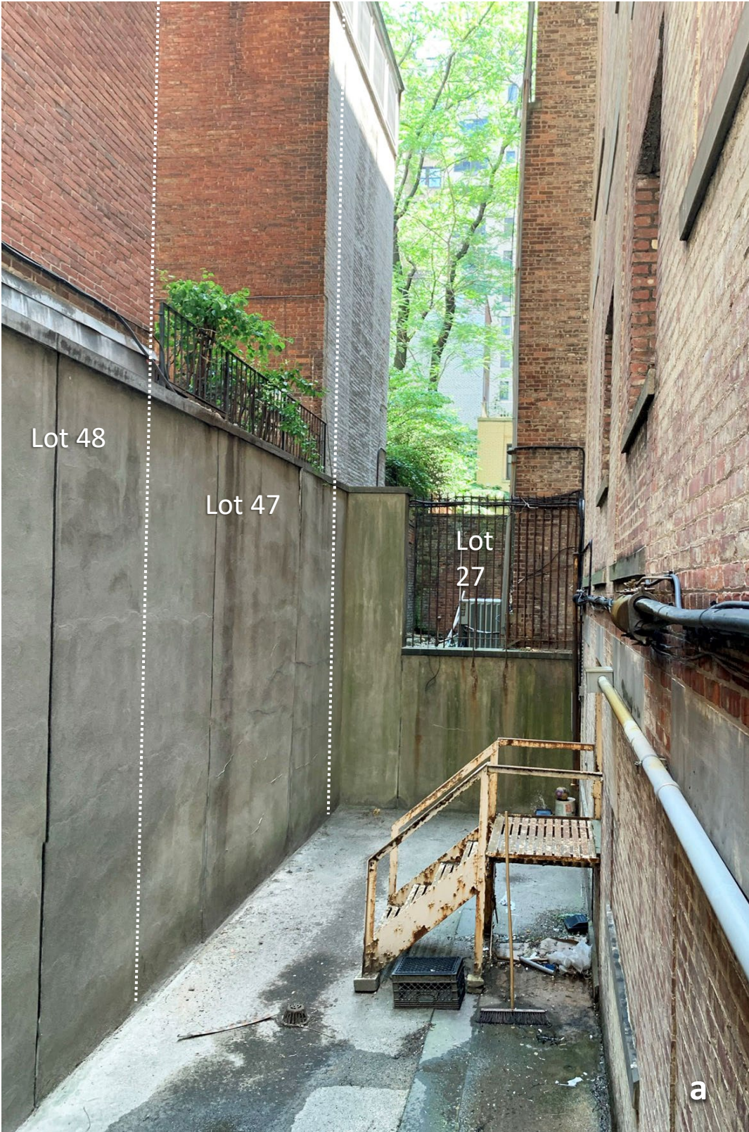
Current photo of rear yard, from neighbor to west (Lot 23)
