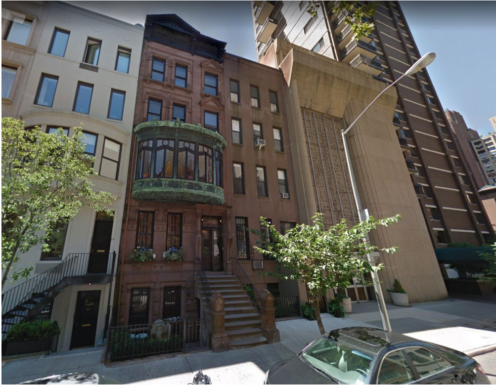
View from E 80 th St (site not visible)
