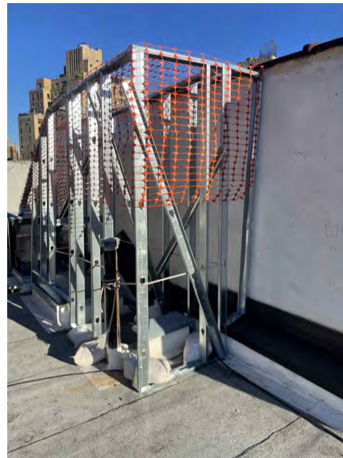
Mockup @ Stair Bulkhead
