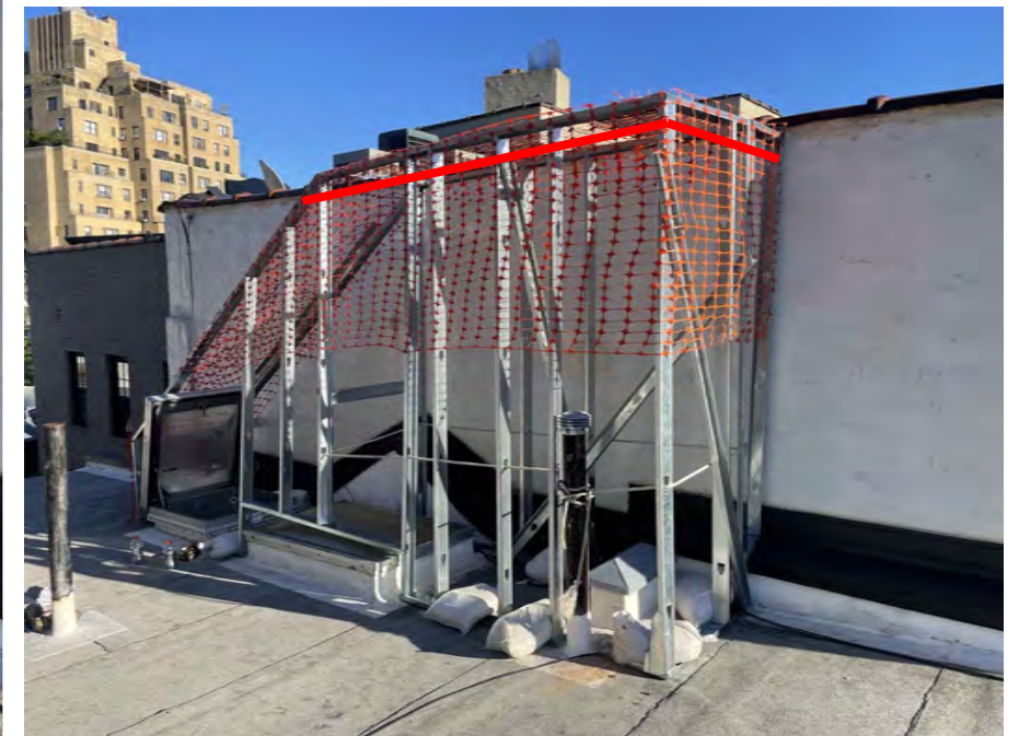
Mockup @ Stair Bulkhead
