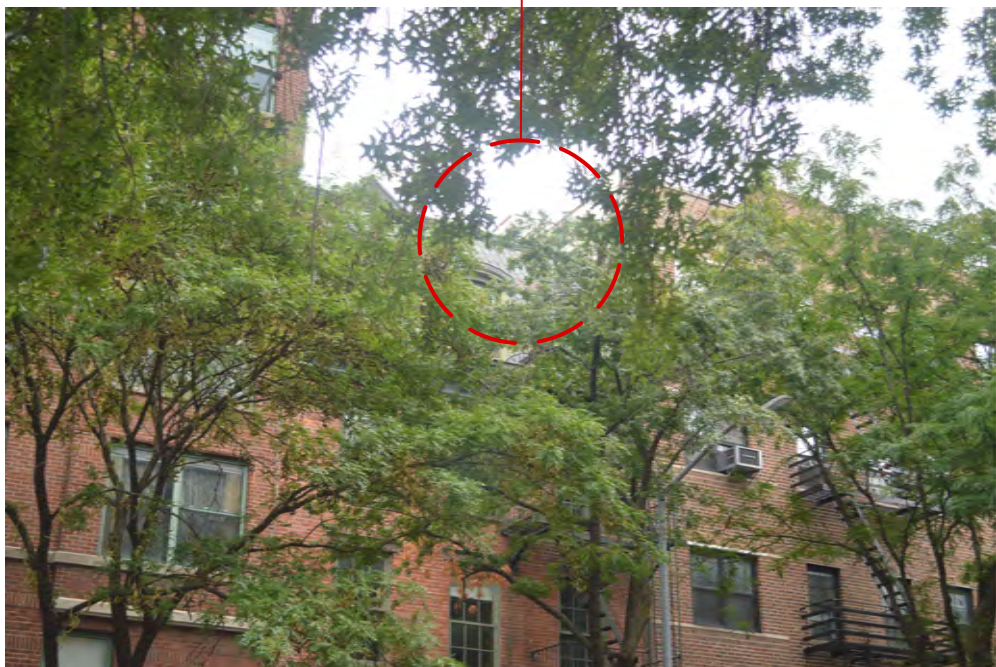
Front of Stair Bulkhead Partially Visible
