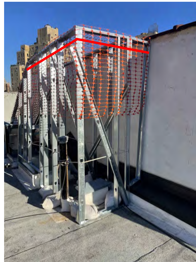
Mockup @ Stair Bulkhead
