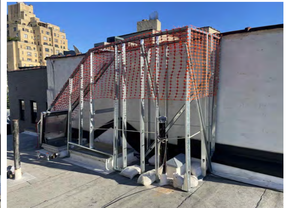
Mockup @ Stair Bulkhead
