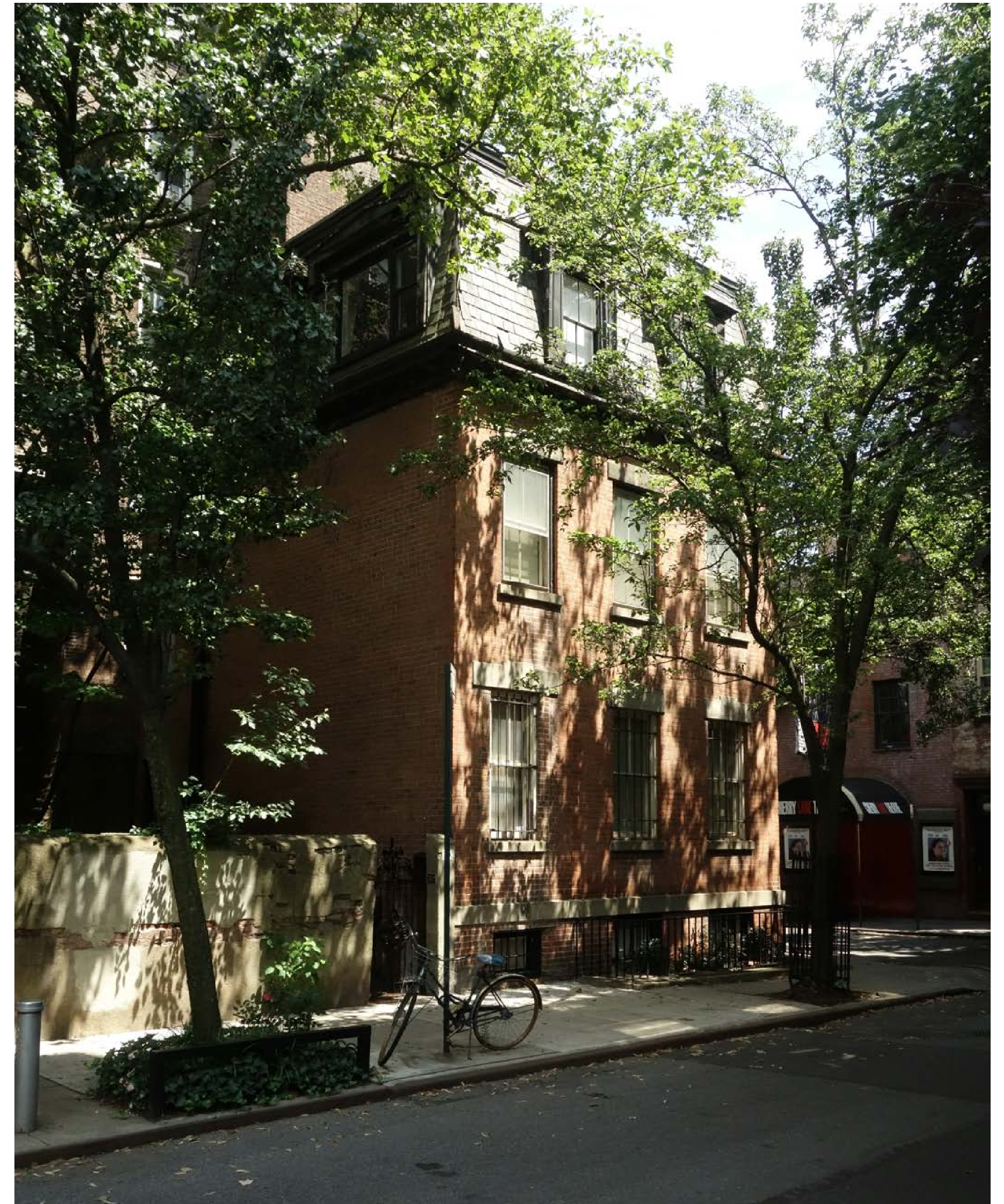
EXISTING BUILDING FACADE
