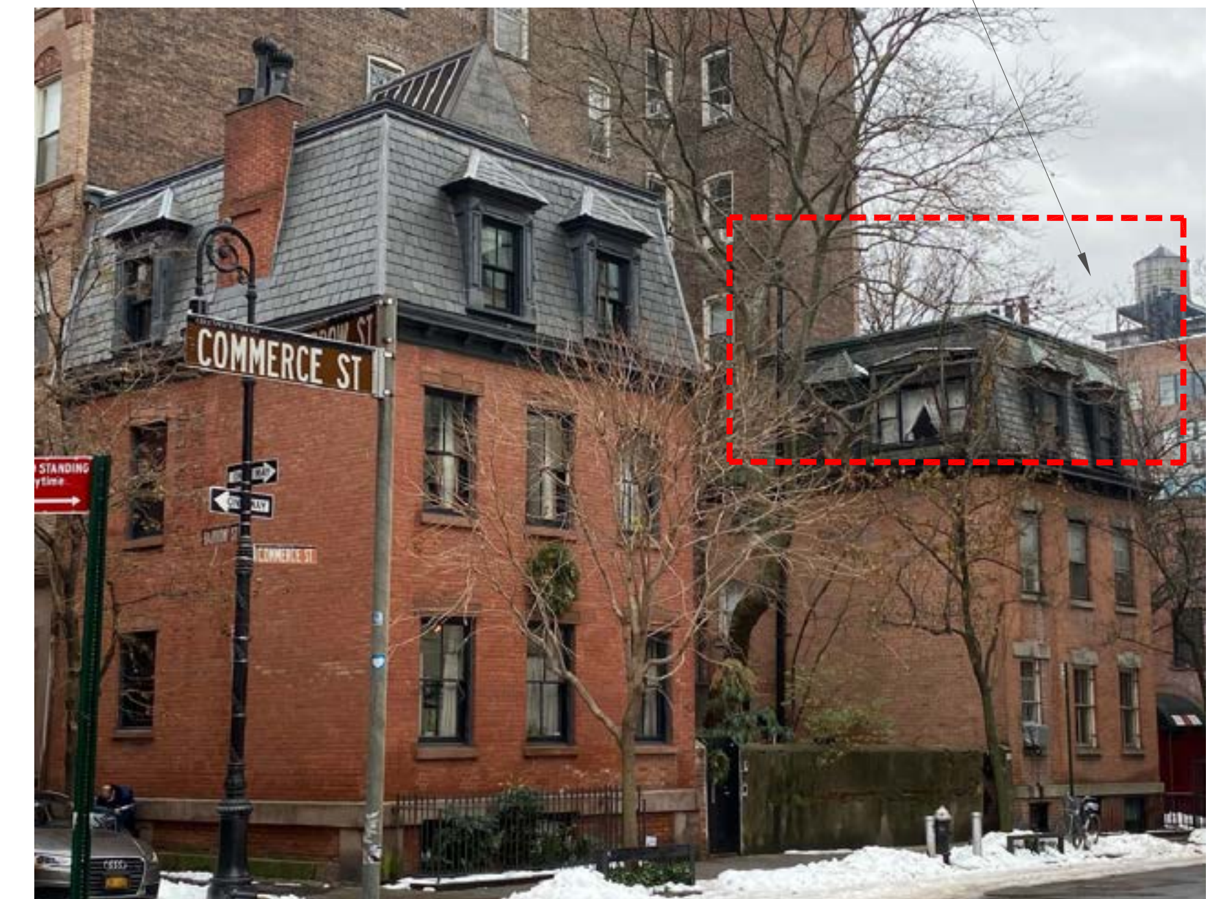
PHOTO OF COMMERCE STREET SOUTHWEST FACADE, 2021, N.T.S.
