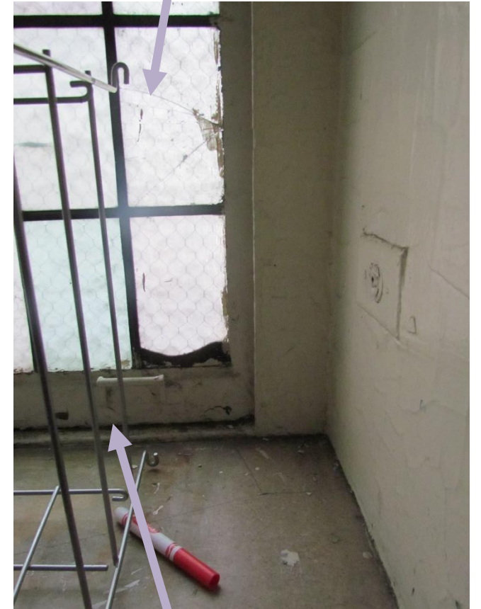
CRACKED GLAZING
