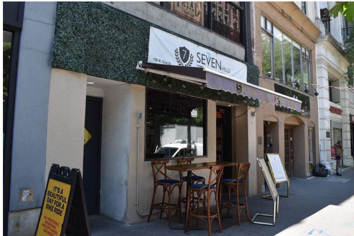
133 W 72nd St. - Stucco Storefront
