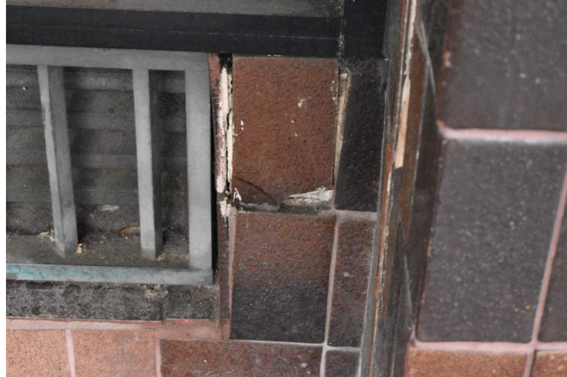
Cracked Tiles Delaminating From Substrate
