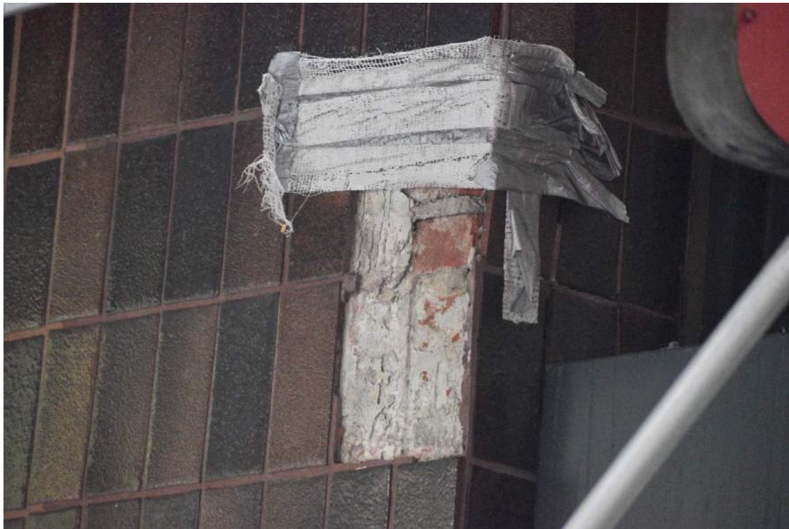
Delaminating Tiles Fallen From Substrate
