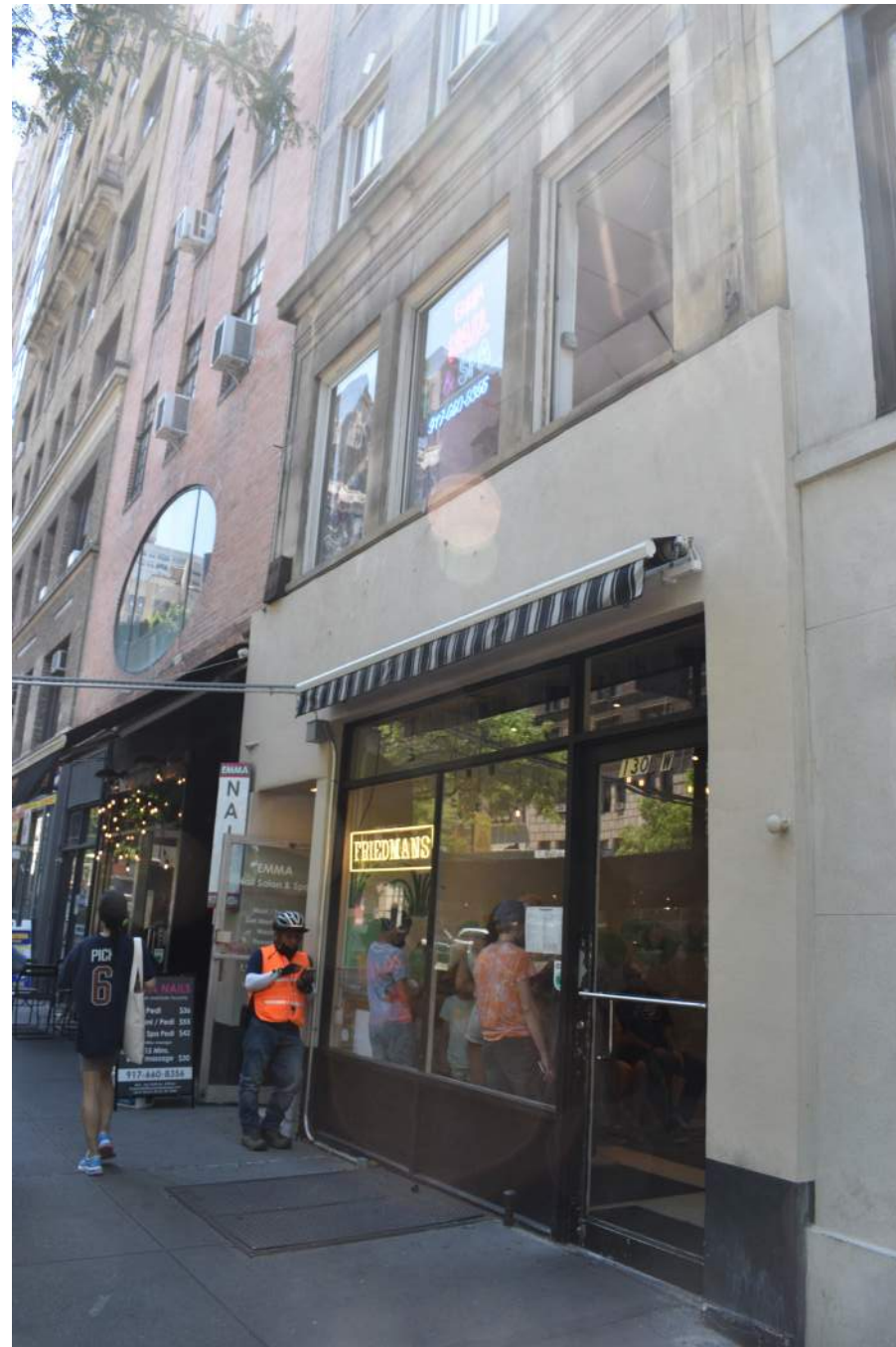
130 W 72nd St. - Stucco Storefront
