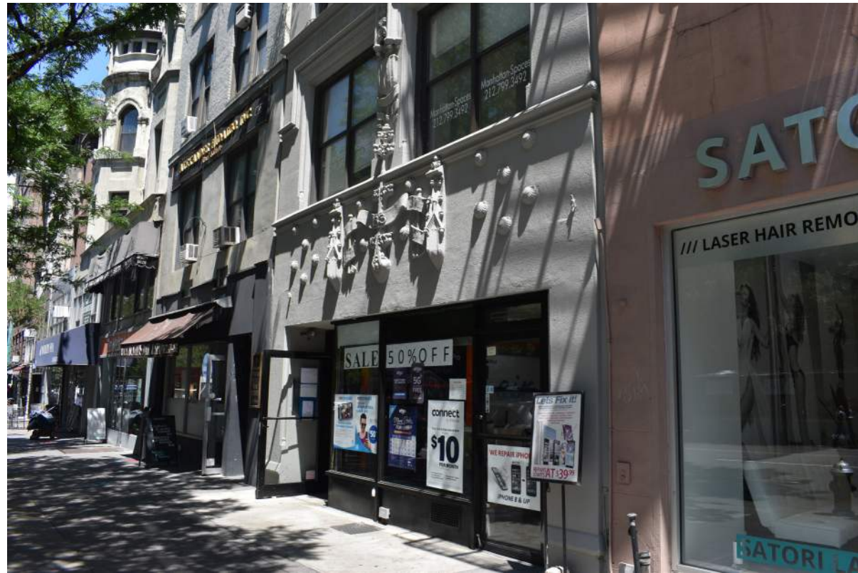
153 W 72nd St. - Stucco Facade
