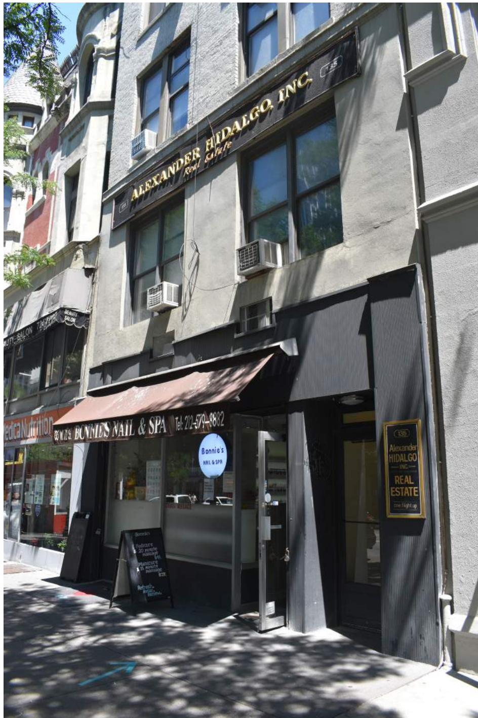
158 W 72nd - Stucco 2nd Floor
