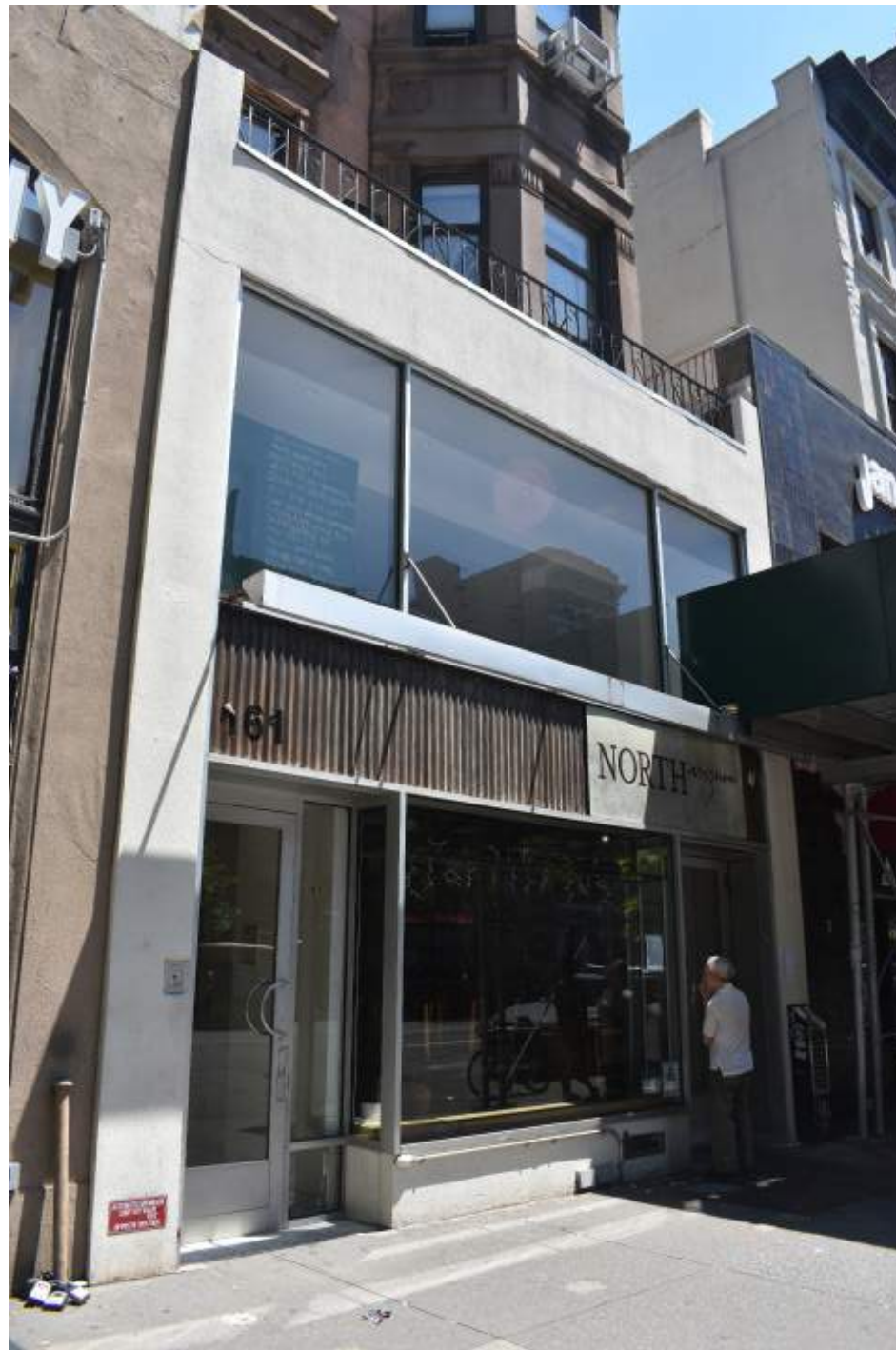
161 W 72nd - EIFS Facade
