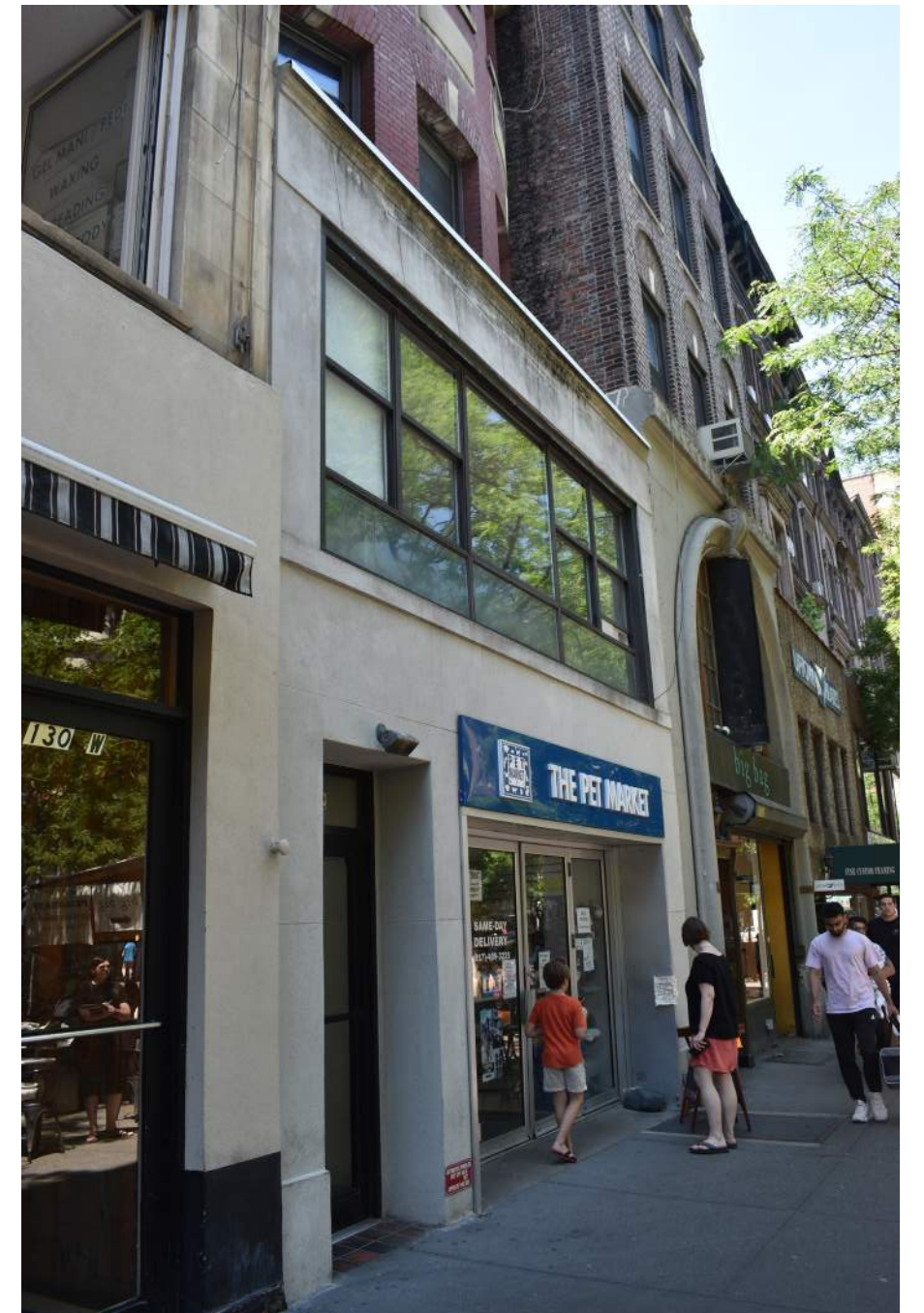
132 W 72nd St. - Stucco Facade
