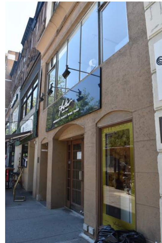
160 West 72nd St. - Stucco Facade
