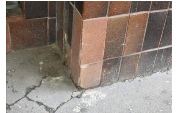
Spalled Tiles
