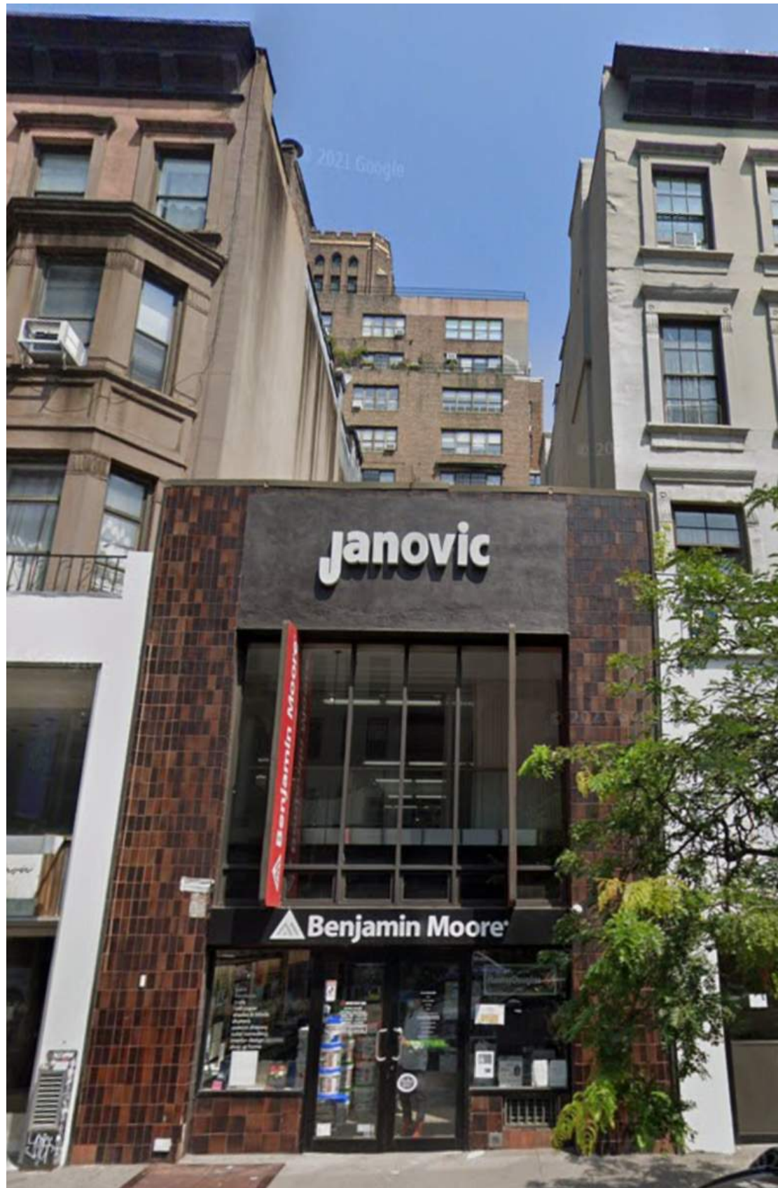
159 W 72nd, Existing Glazed Masonry Tiles
