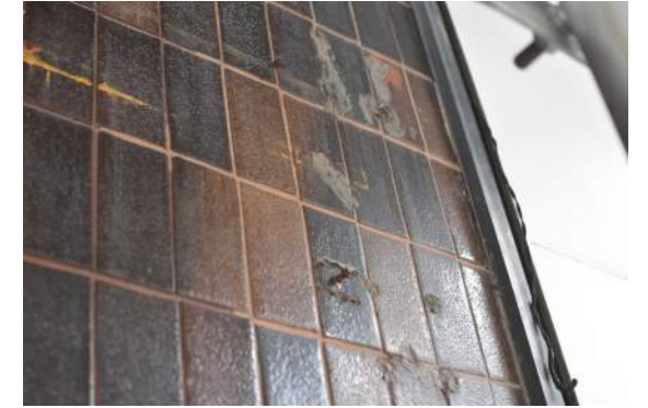
Spalled Tiles
