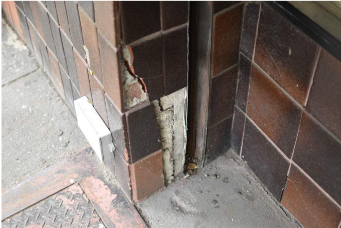
Cracked and Delaminated Tiles
