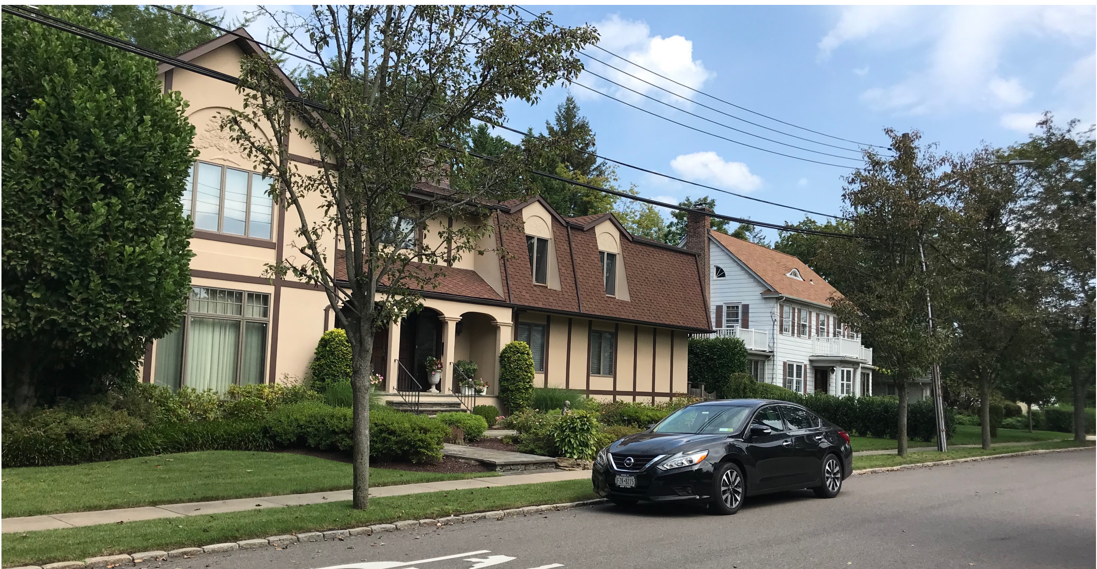
VIEW OF PREMISES STREETScape FROM WEST DRIVE
