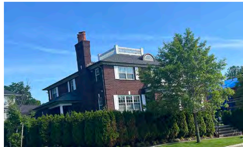
EXISTING REFERENCE: 27-03 SHORE RD, DOUGLASTON, NY
