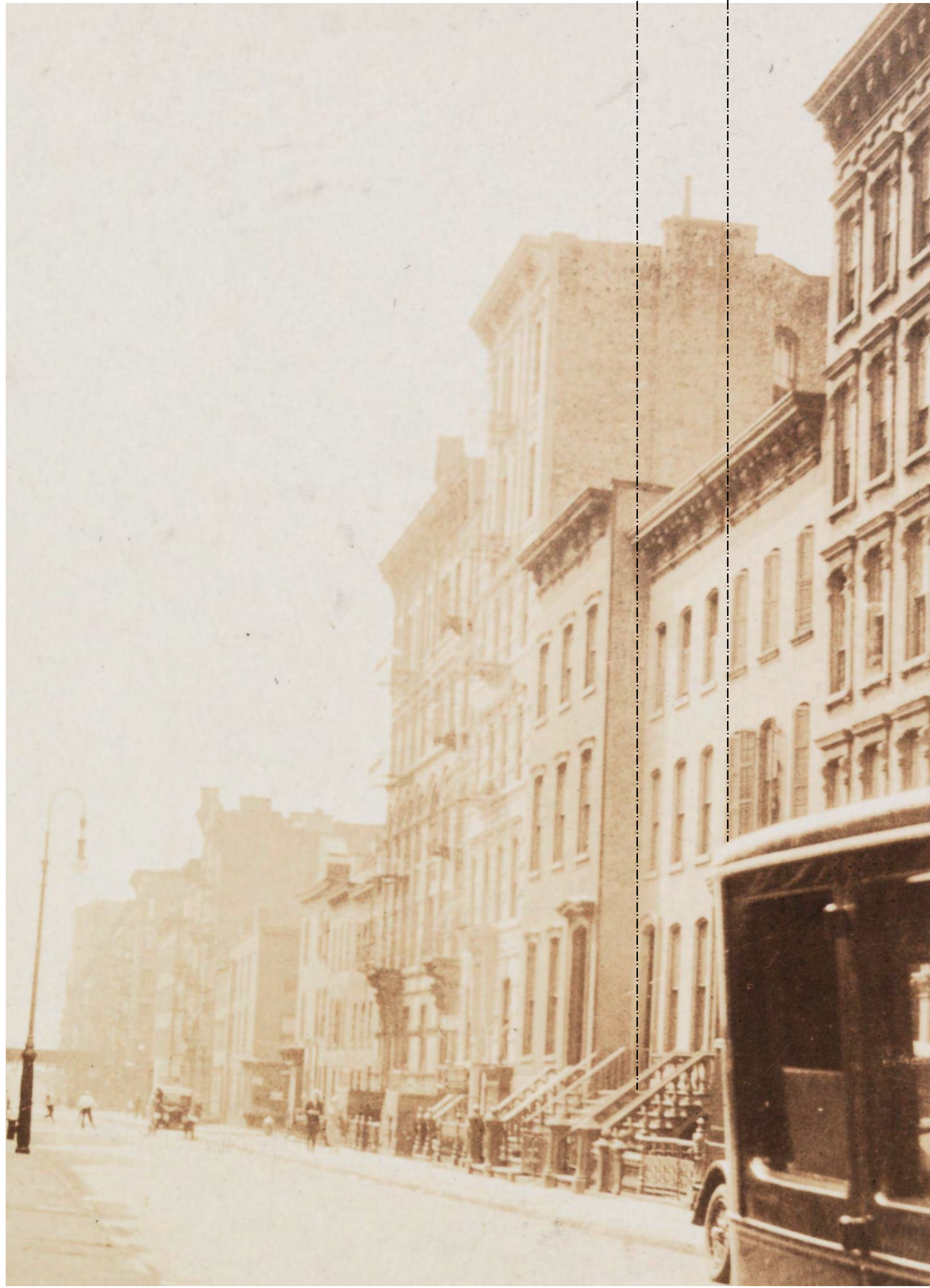
2 Perry St: (1925, Before Renovation) SCALE: 1:0.33
