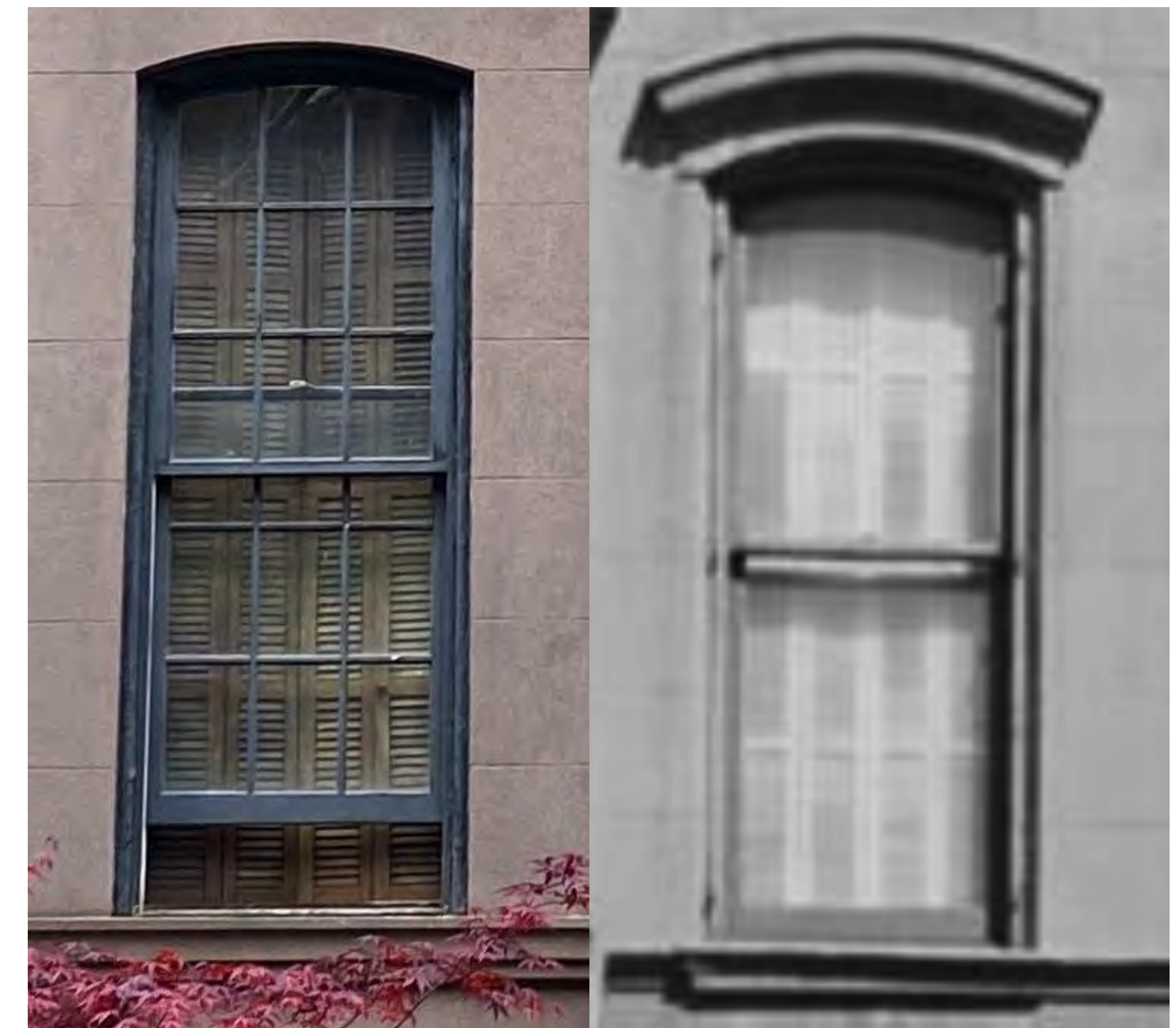
2 1st Floor Windows (Before & After Renovation) SCALE: 1:1.25
