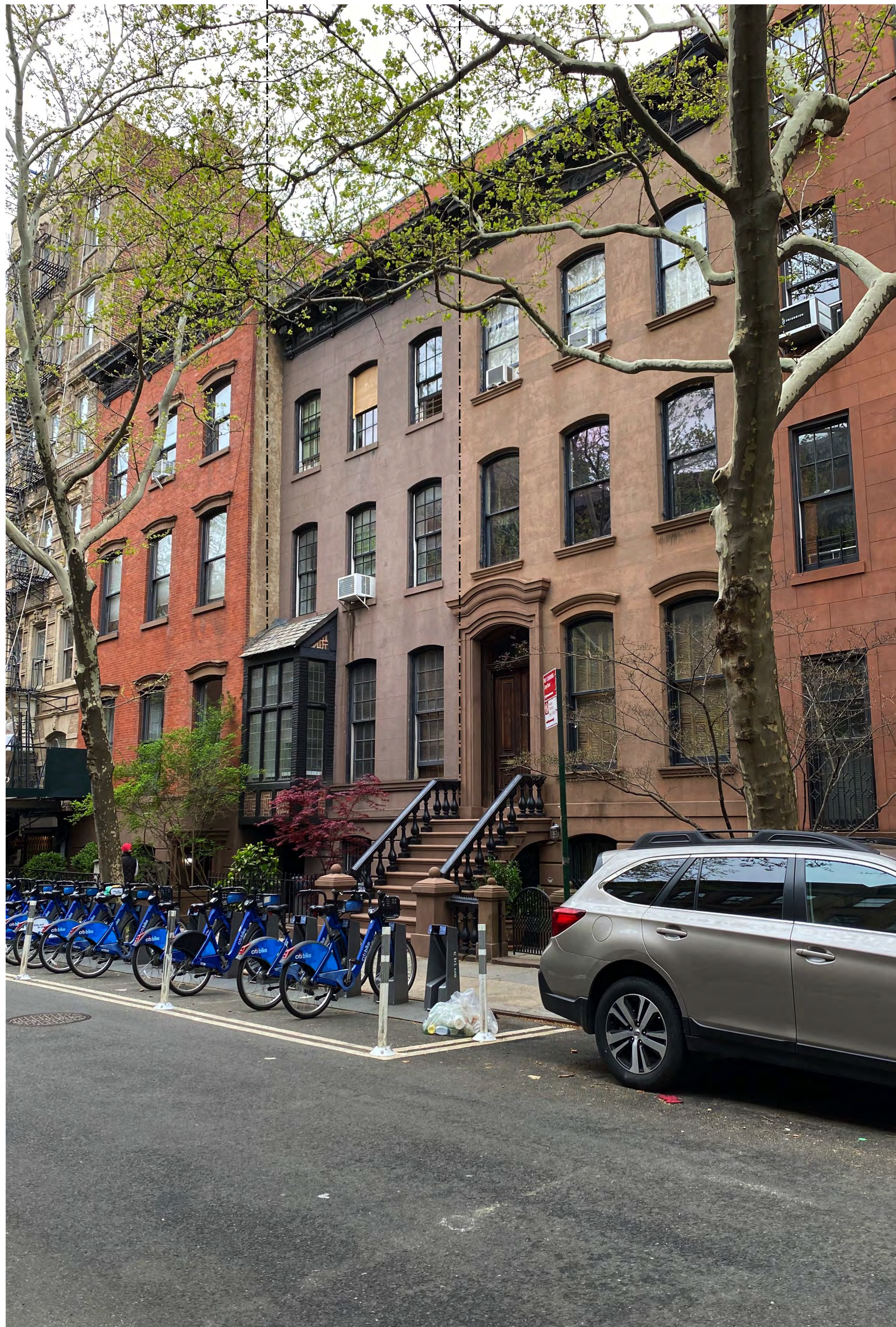
1 73 Perry St: Existing Photo SCALE: 1:2.70
