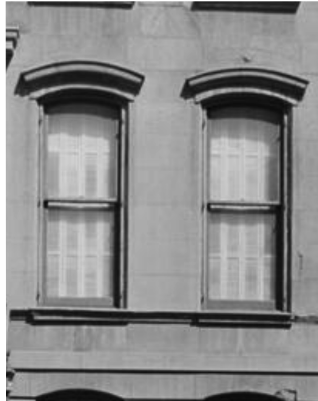
3 B: Window Lintel & Sill Details SCALE: 1:0.67
