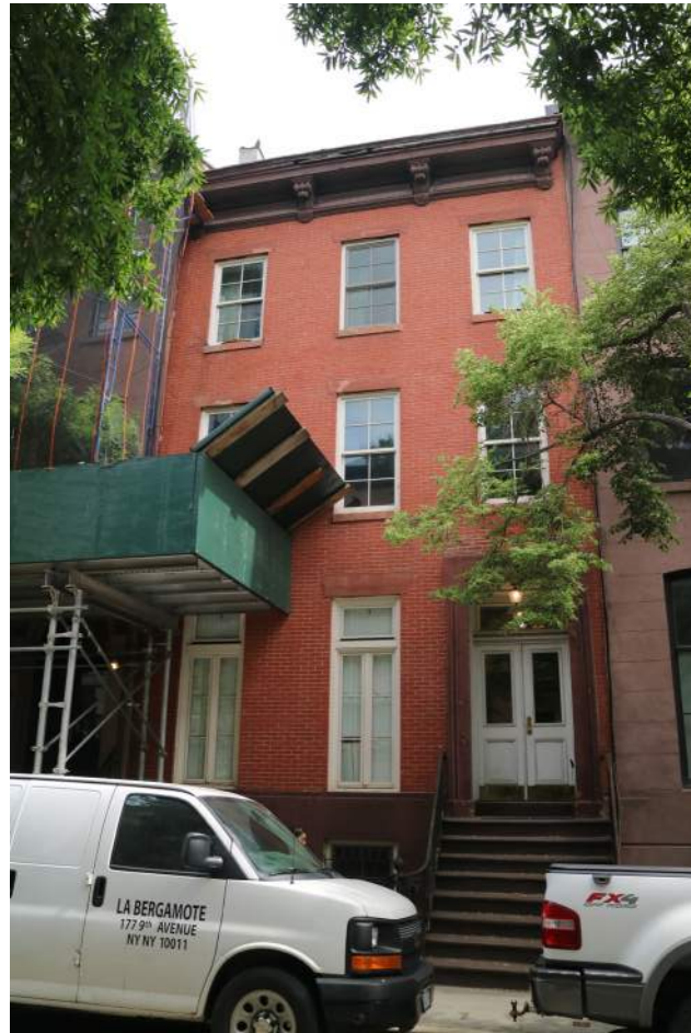
existing (close up)
