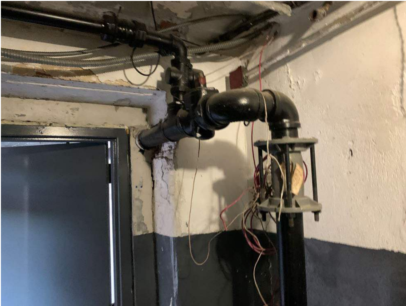
EXISTING GAS SERVICE LINE BELOW MAIN ENTRANCE FLOOR
