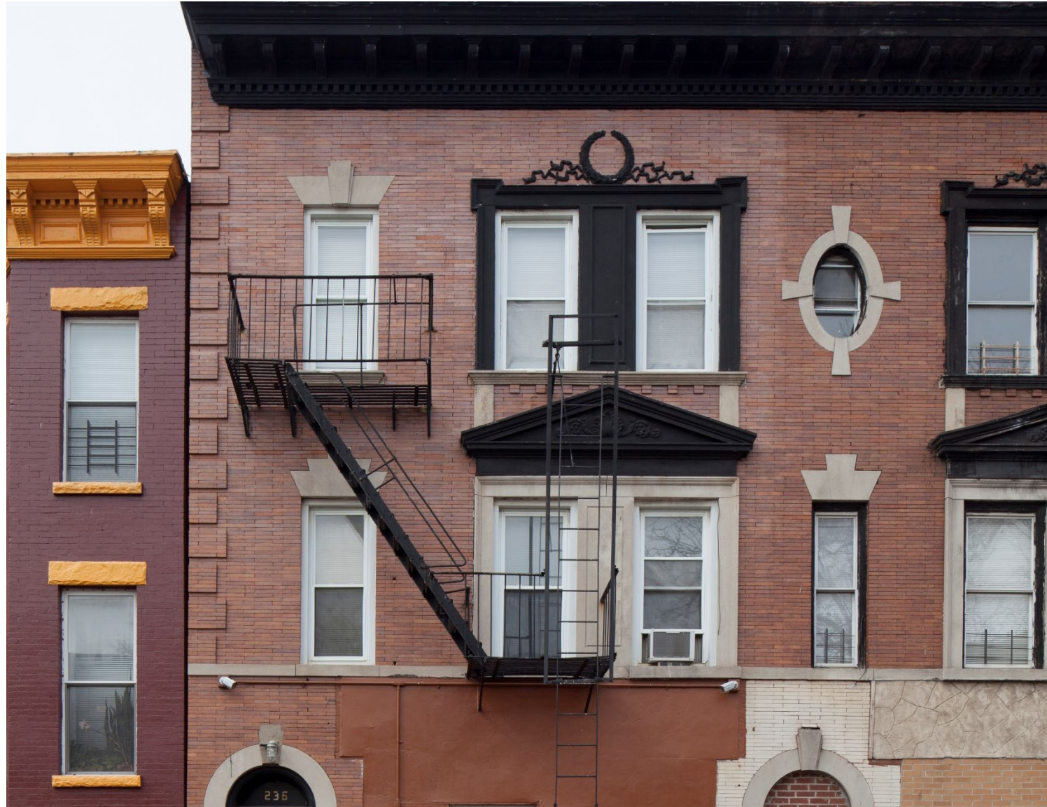
Upper floors – condition at LPC designation (c. 2015)
