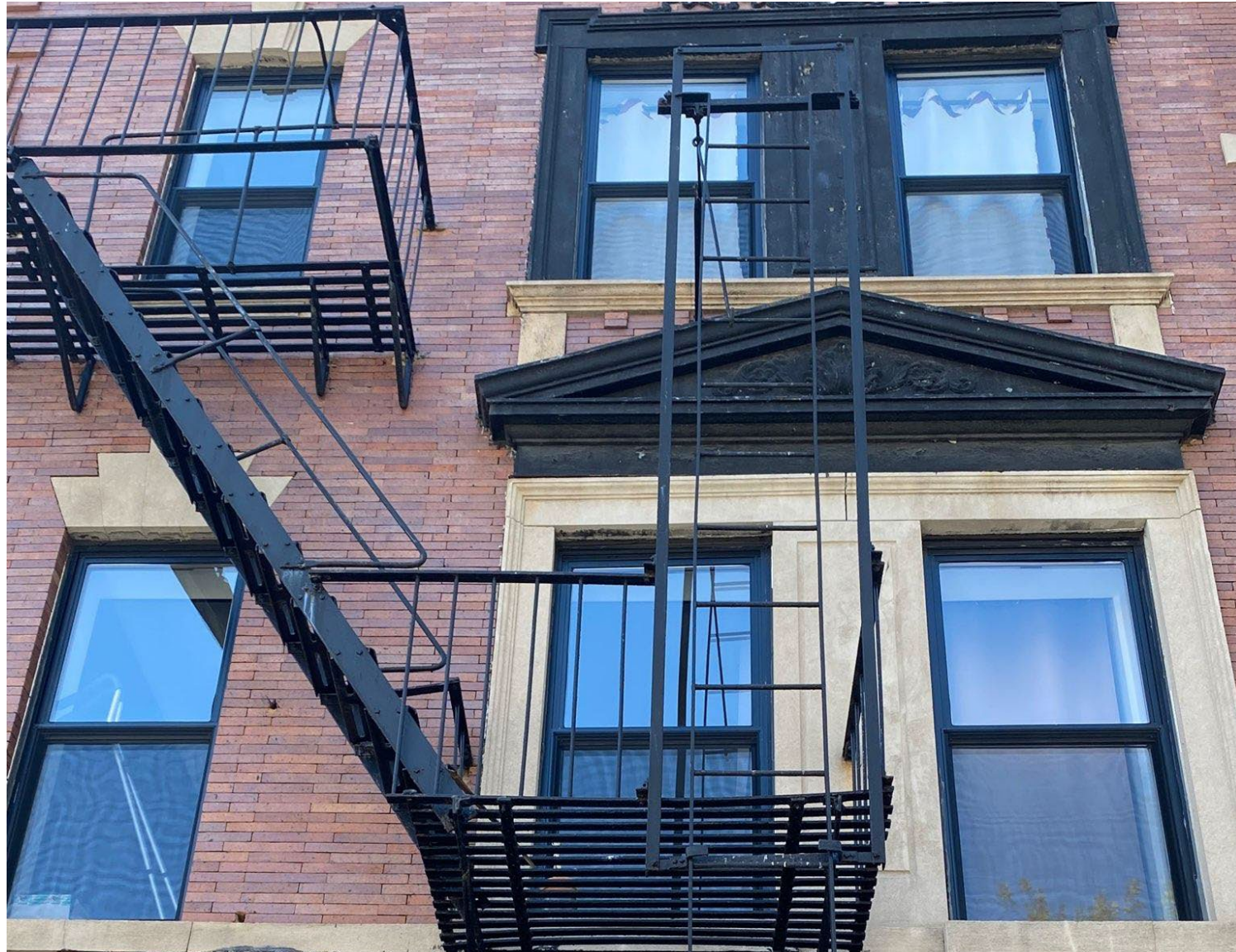
Close-up view of upper windows
