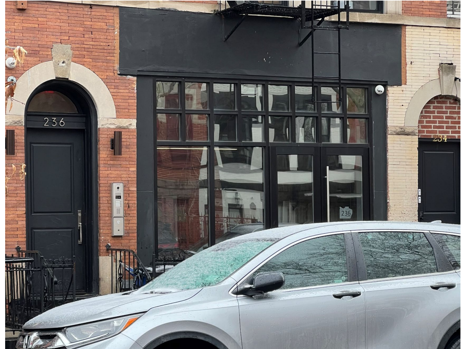
Close-up view of entry door and storefront
