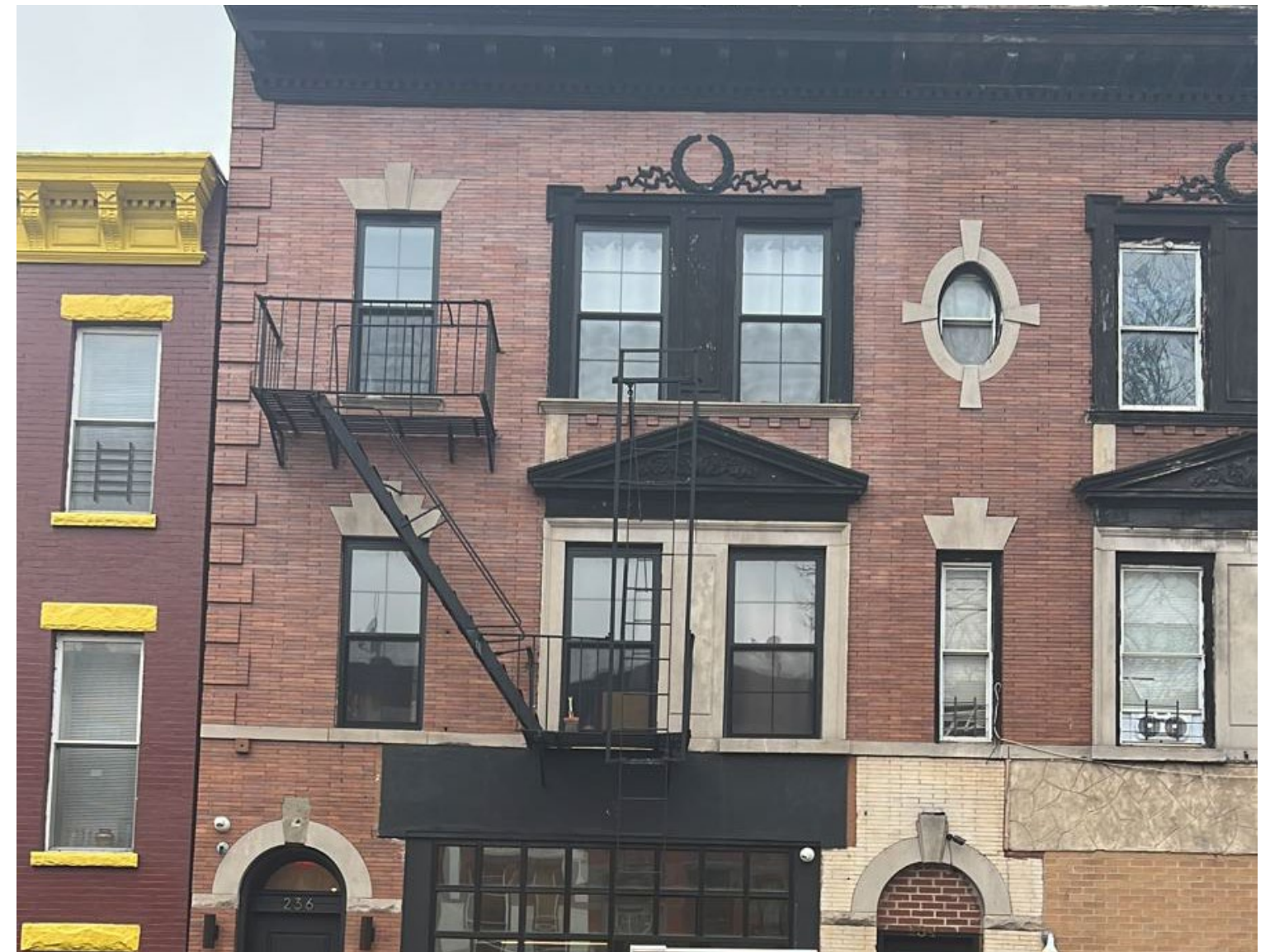
Warning Letter 22-0218 issued for "Replacement of windows at 2nd and 3rd floors and entry door at ground floor without permit(s)."
