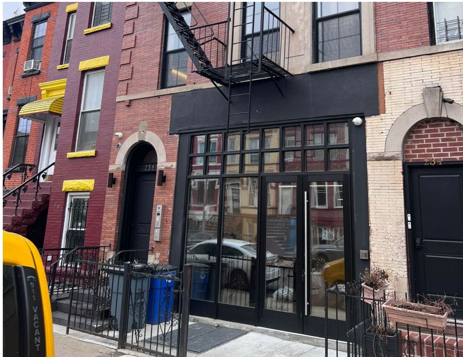
Warning Letter 22-0217 issued for "Installation of storefront infill at ground floor without permit(s)."
