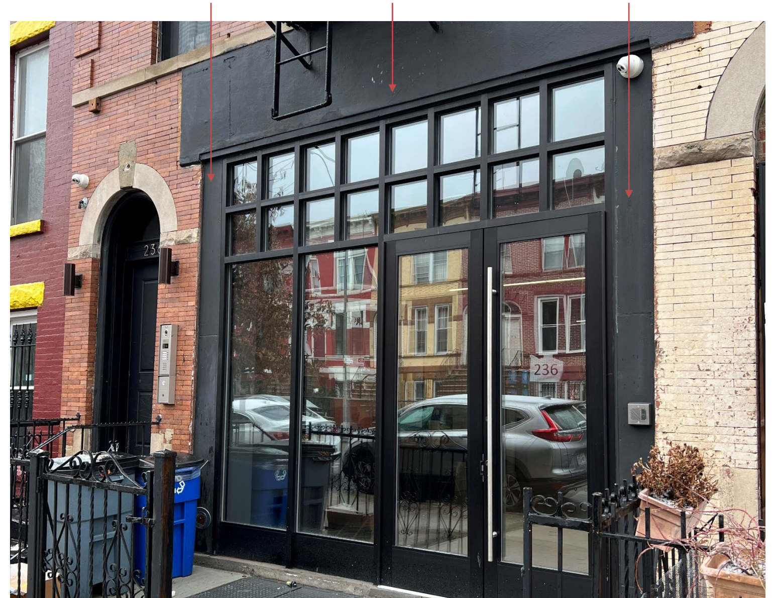
Additional views of 1 st floor work
