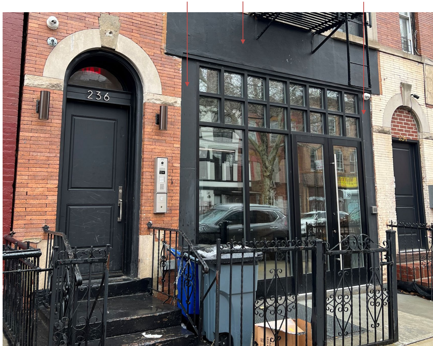
Additional views of 1 st floor work
