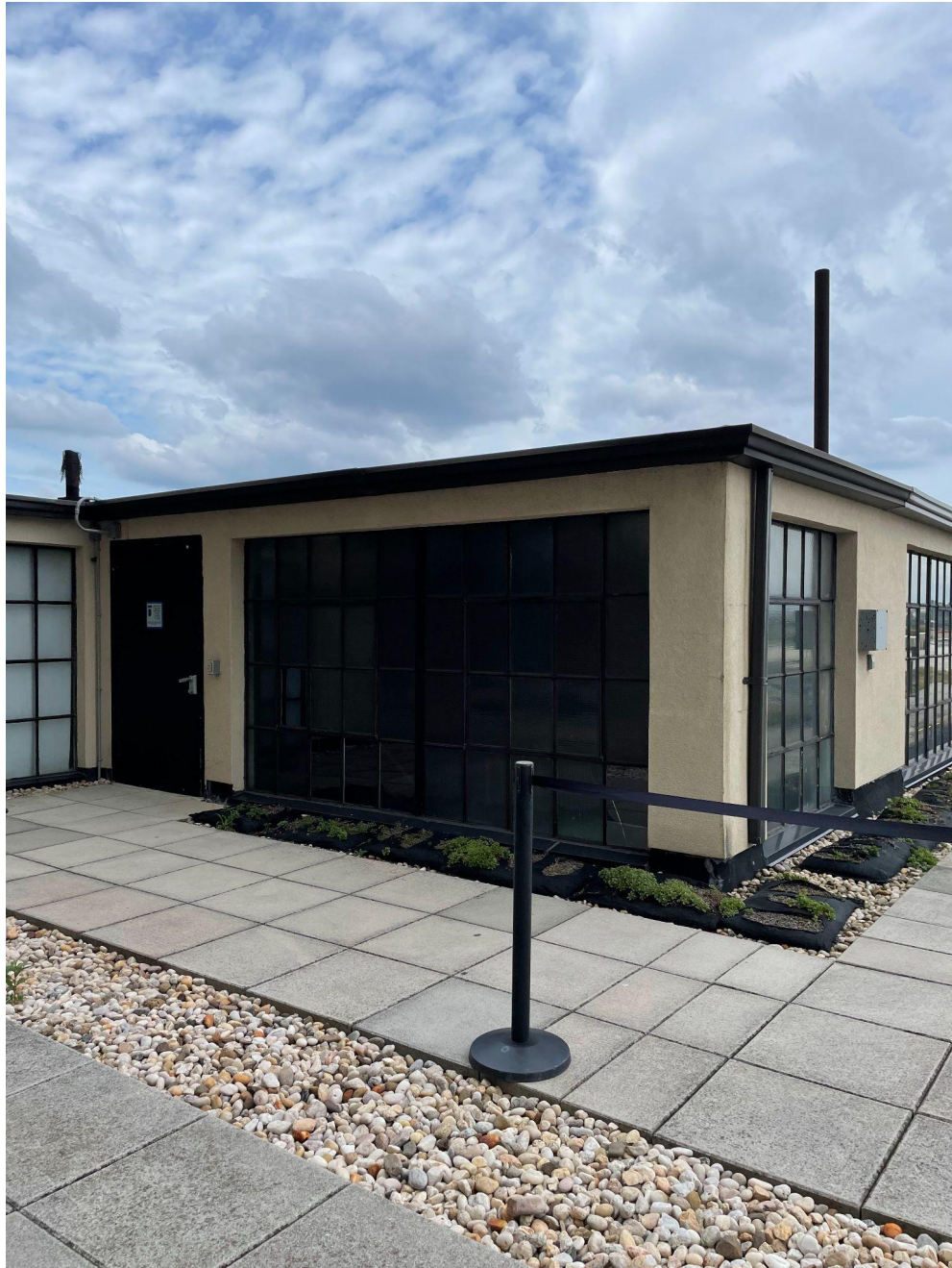
STAIR D EXISTING CONDITIONS 10TH FLOOR
