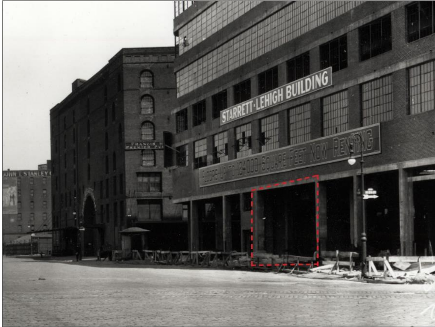
1931 Historic Photo, View Northeast at 12th Avenue Facade (Municipal Archives)
