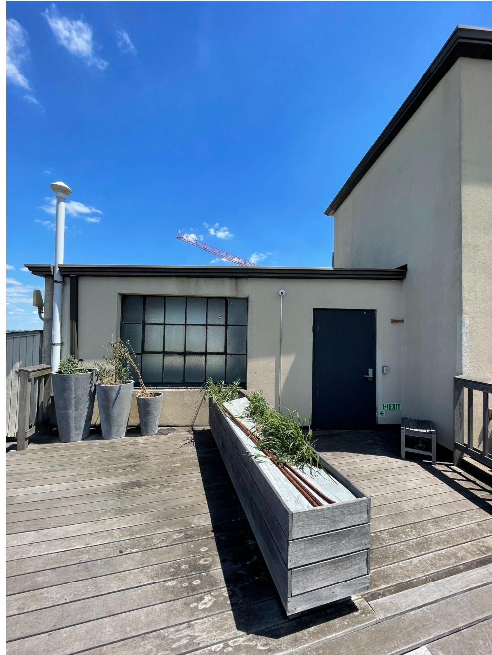
STAIR E AND BULKHEAD EXISTING CONDITIONS
