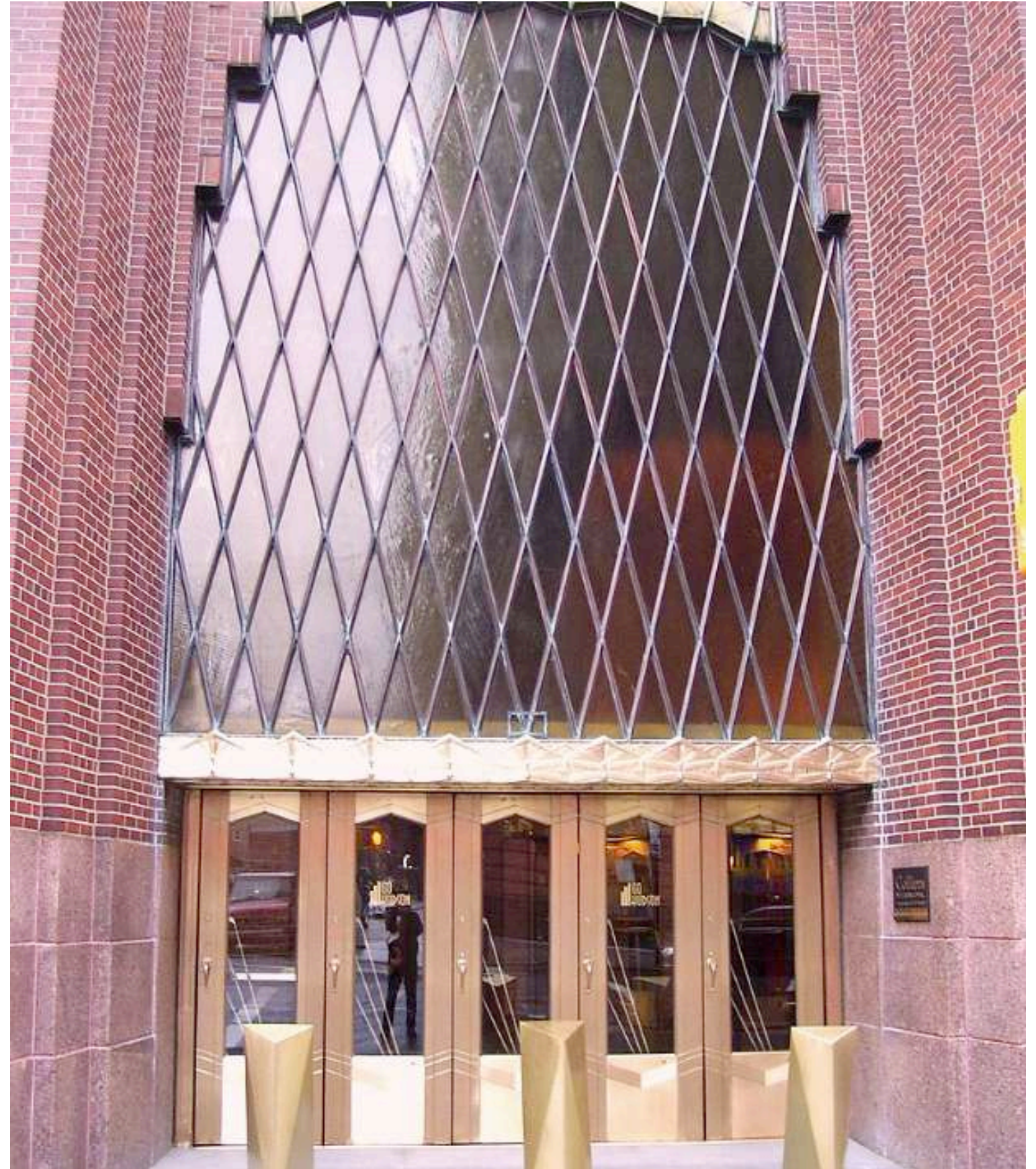
EXISTING ENTRANCE CONDITION
