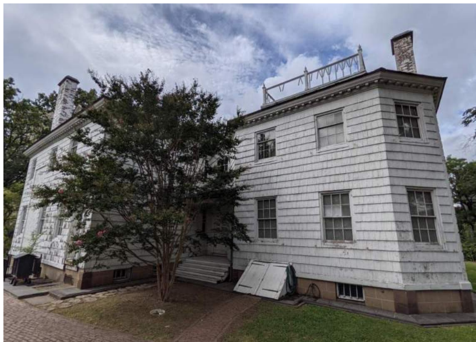
6. View of East Elevation at location of proposed ramp
