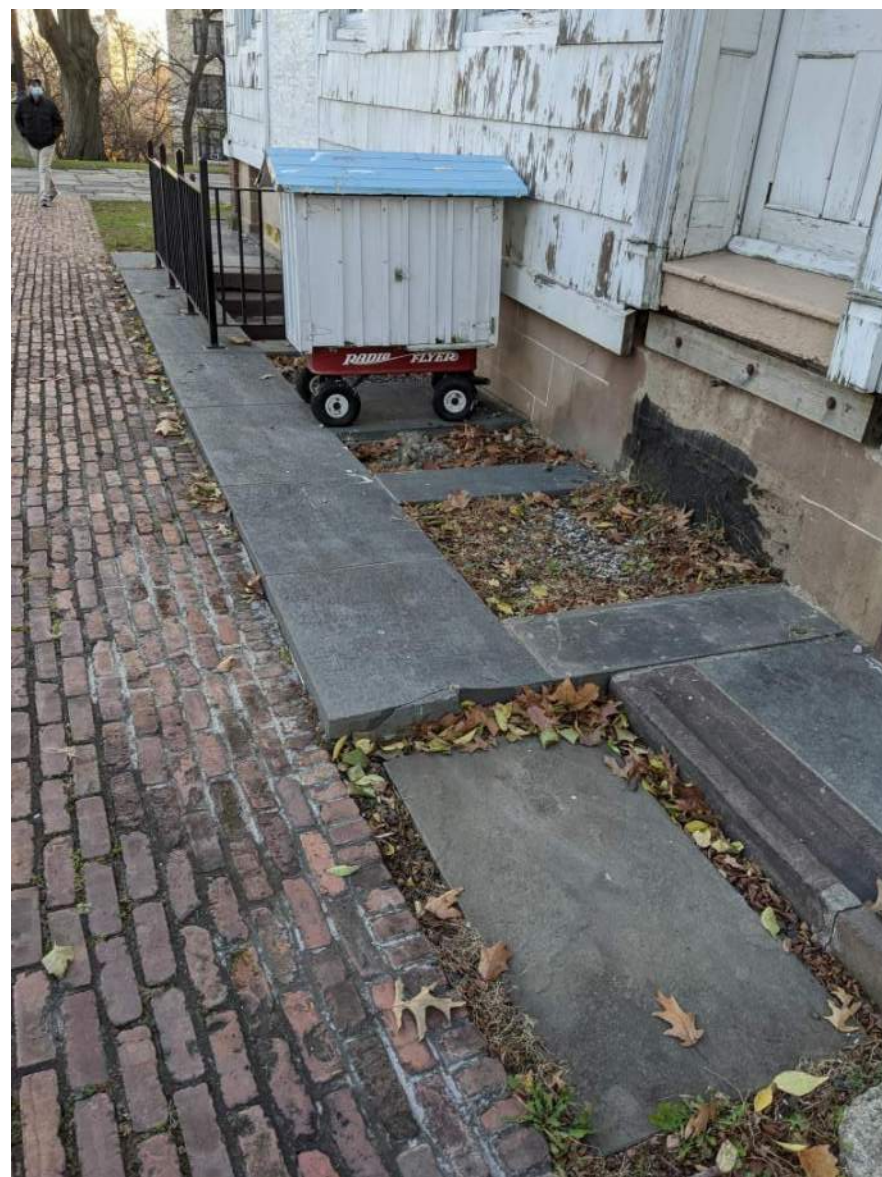
14. View of East walking path at location of proposed ramp
