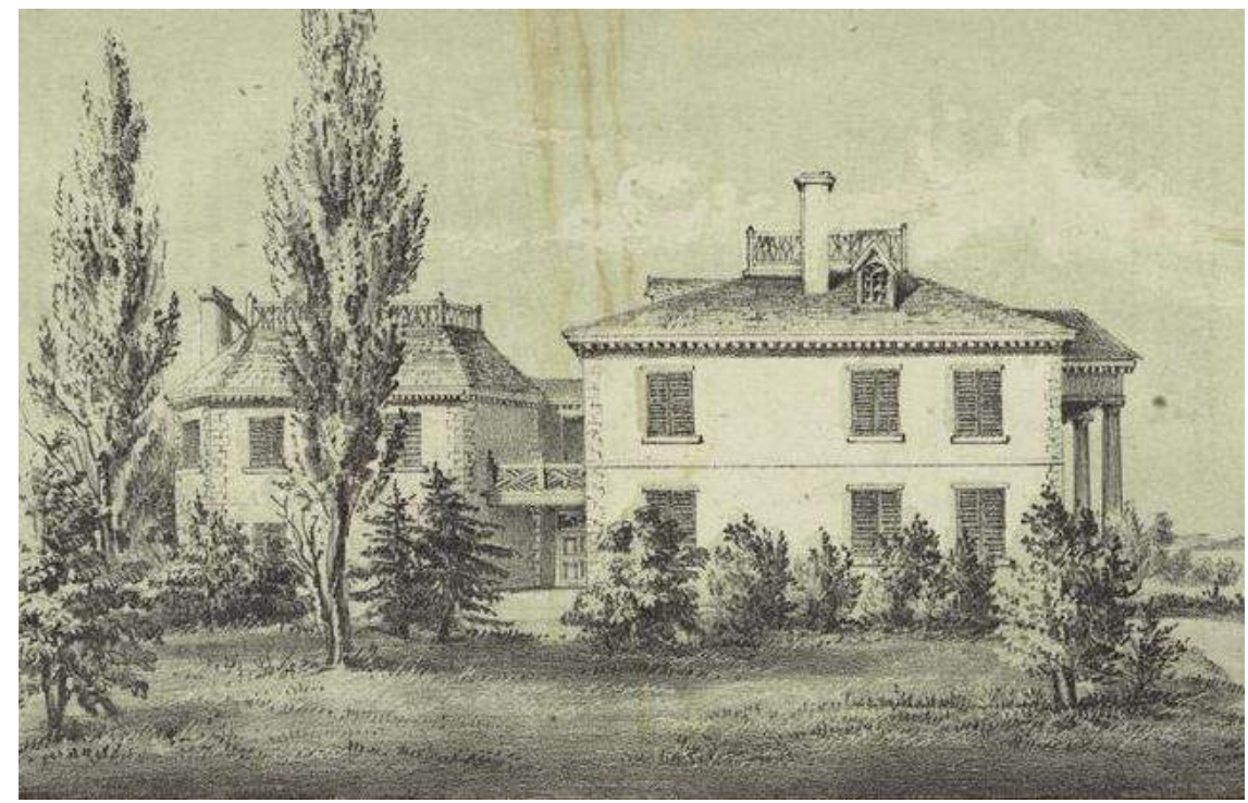
Engraving of the West Elevation. Note the roof railings at the Main Block, Octagon Wing & Hyphen C. 1854, NYPL
