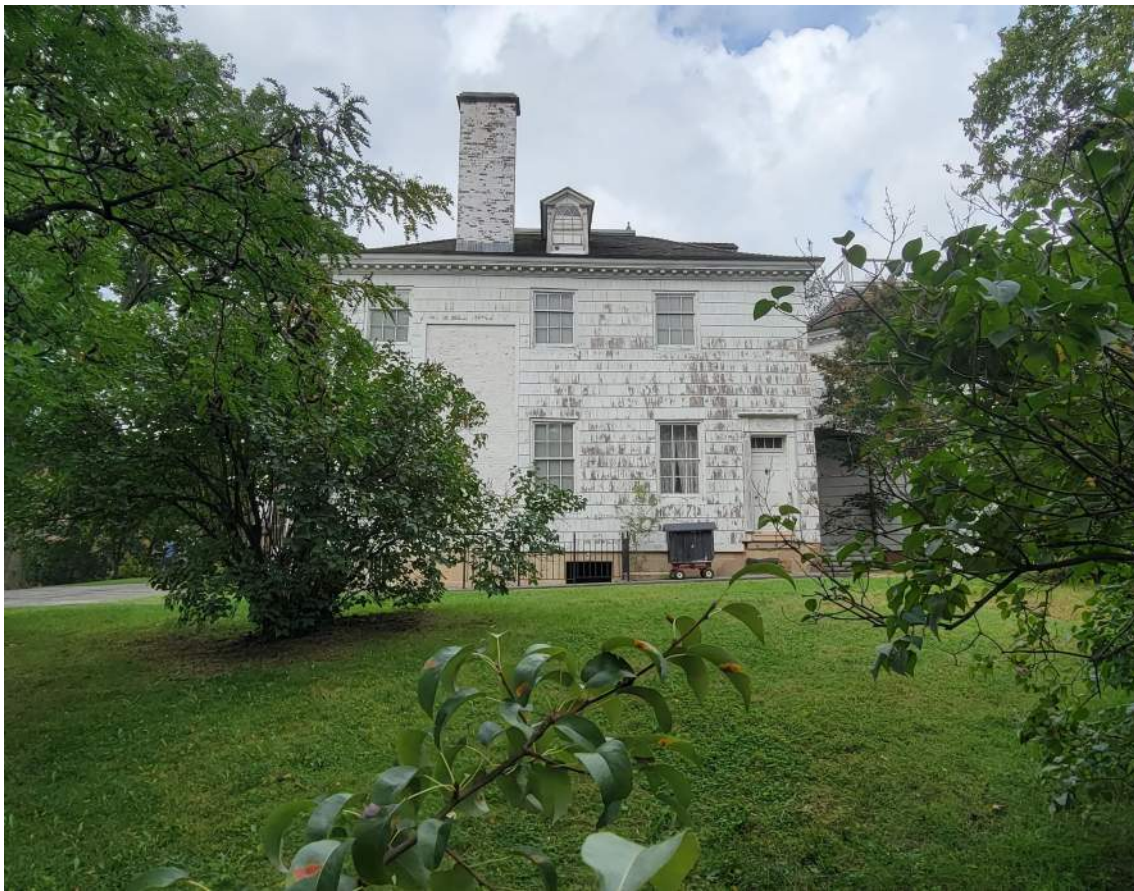
9. View of Southern end of East Elevation, Existing Conditions
