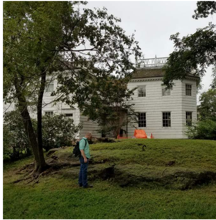
11. View of East Elevation, Existing Conditions
