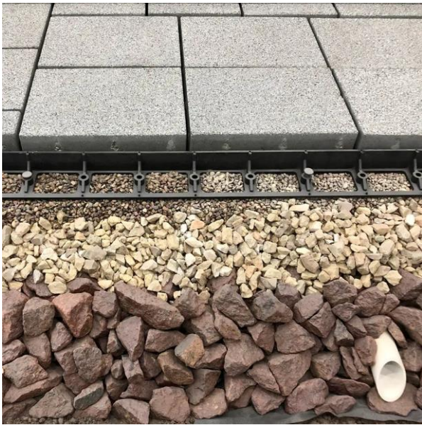
Permeable paving at Hessian Hut area
