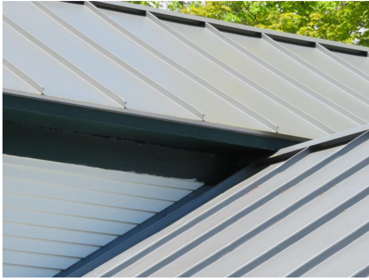
Standing seam metal roofing
