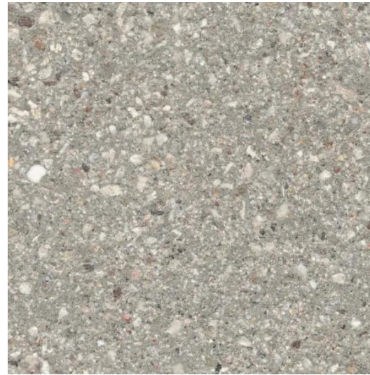
Permeable pavers & concrete
