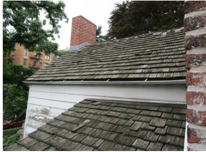
Wood shingle roofing
