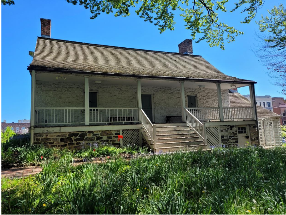
West elevation and porch
