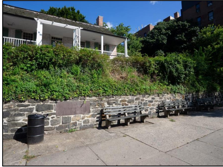
Broadway sidewalk with east porch above
