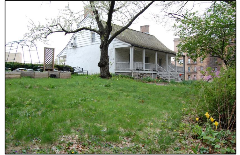
East elevation from the Hessian Hut
