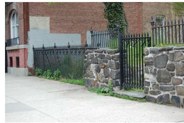
Existing wall and fence at 204 th Street
