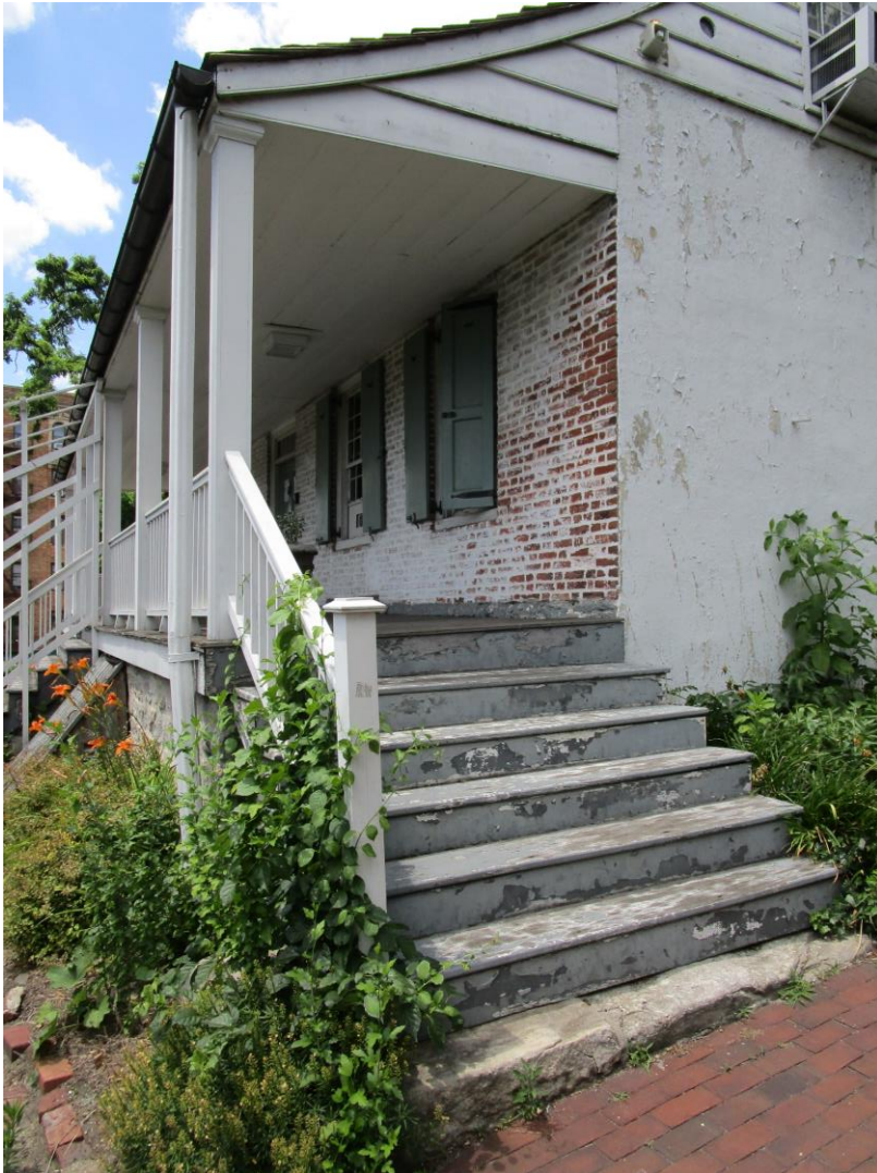
Northeast stair to porch
