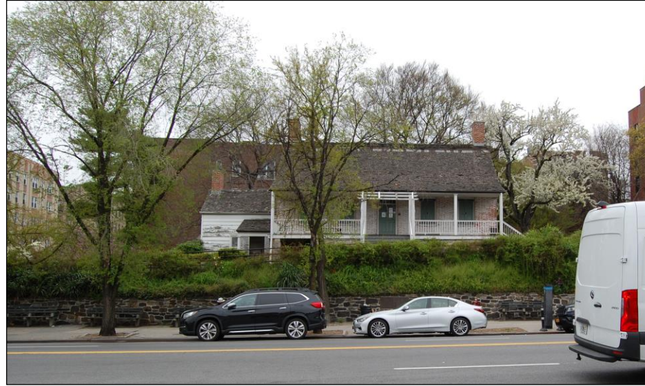
East elevation from Broadway
