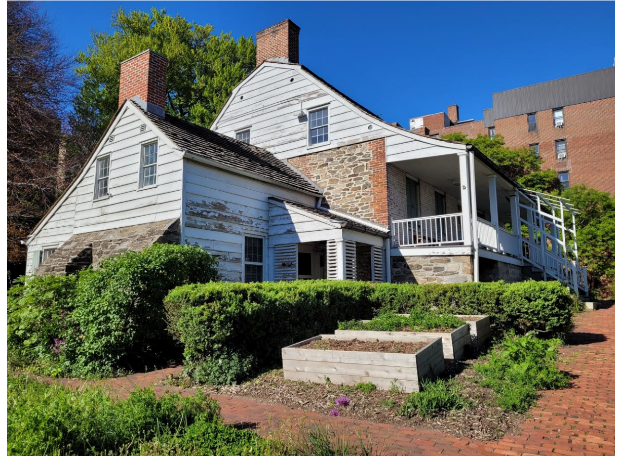
View from the southeast
