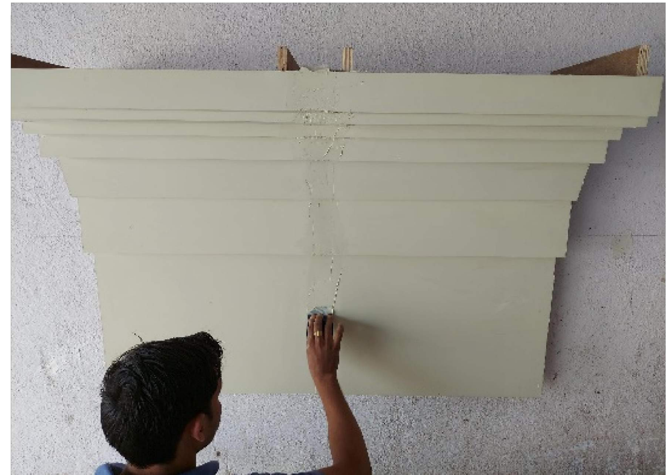
9. APPLY PUTTY TO TAPED JOINT
