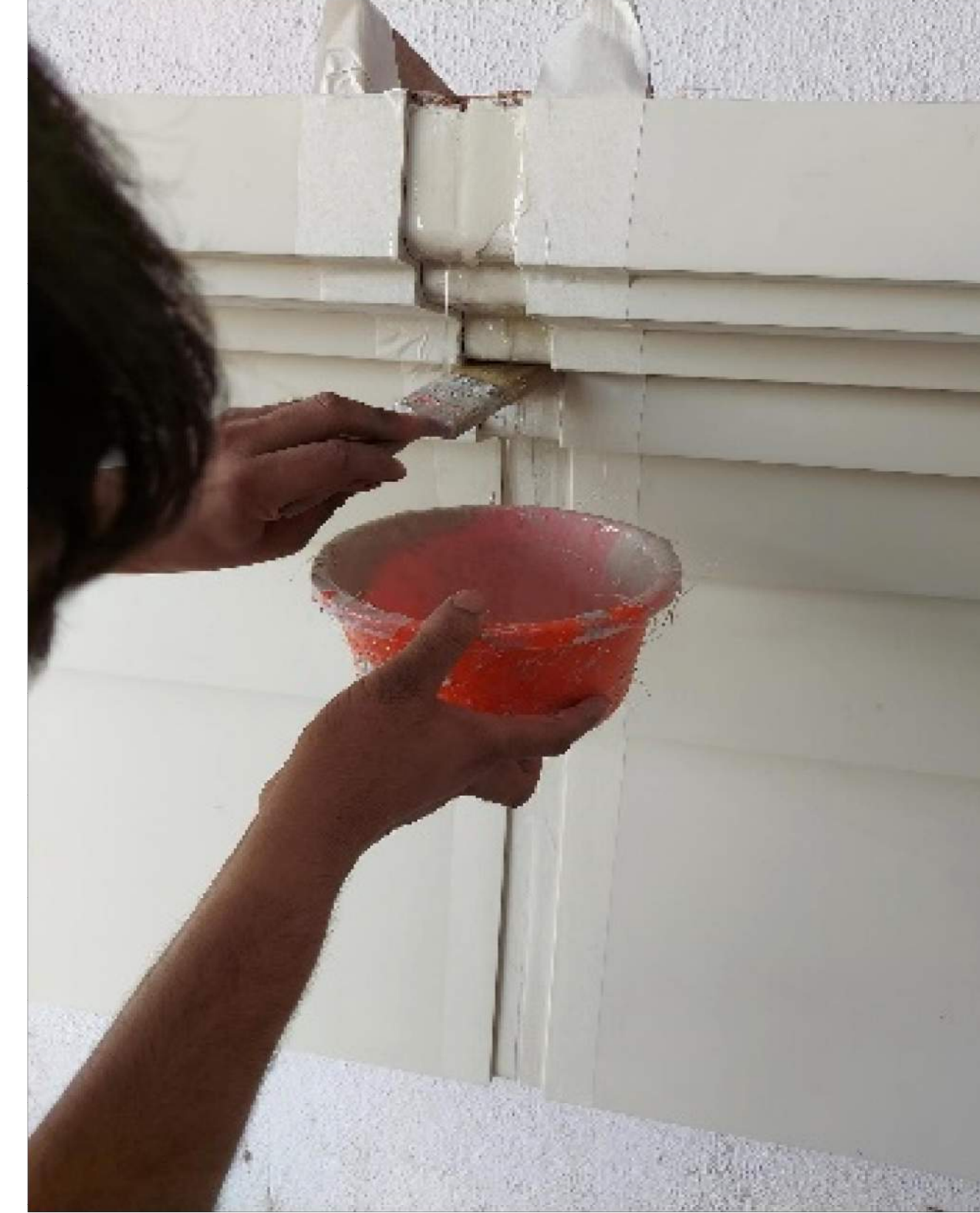
5. APPLY RESIN ON RECESS JOINT AREA
