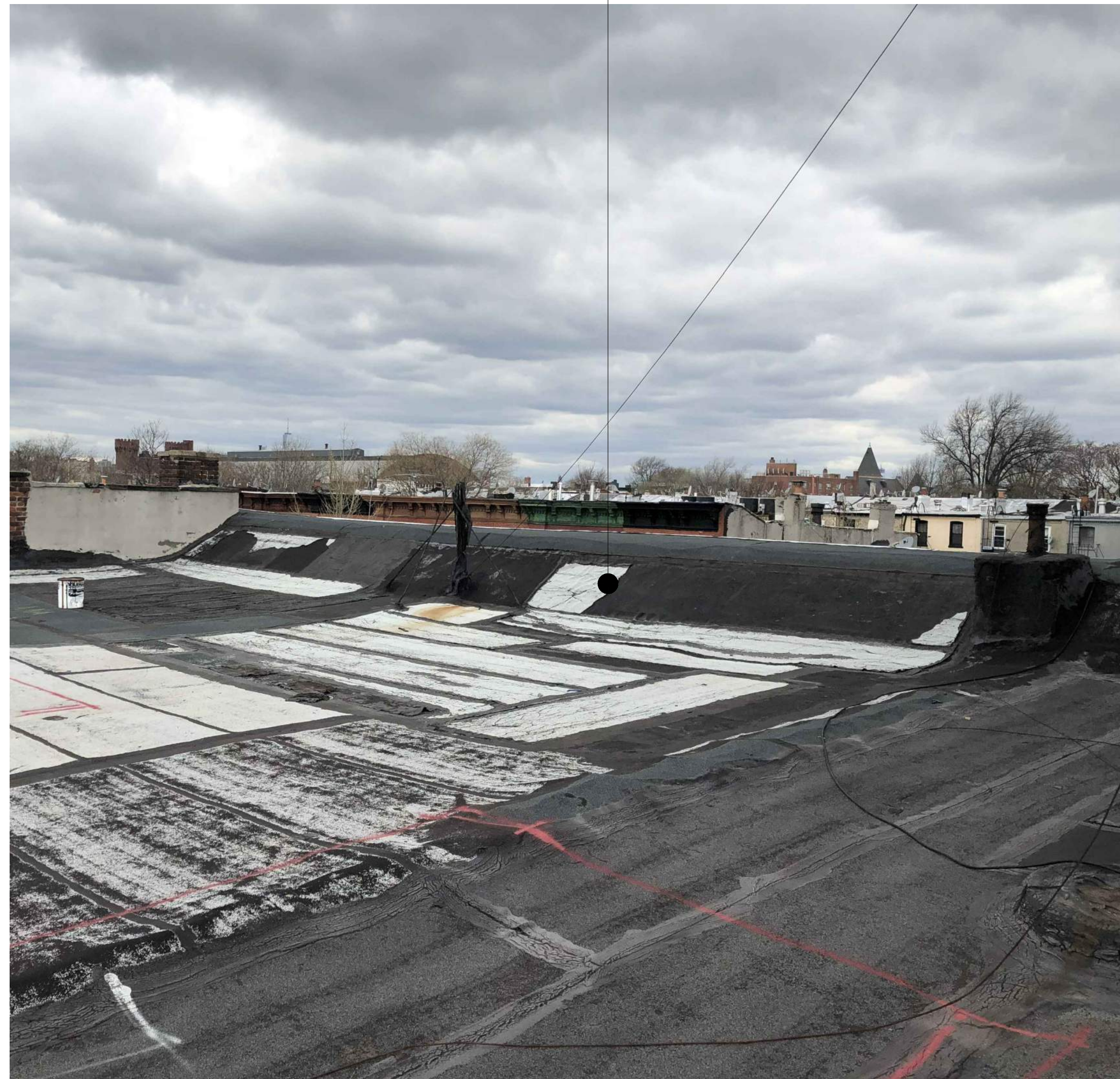
PRIOR TO CONSTRUCTION ROOF PHOTO
