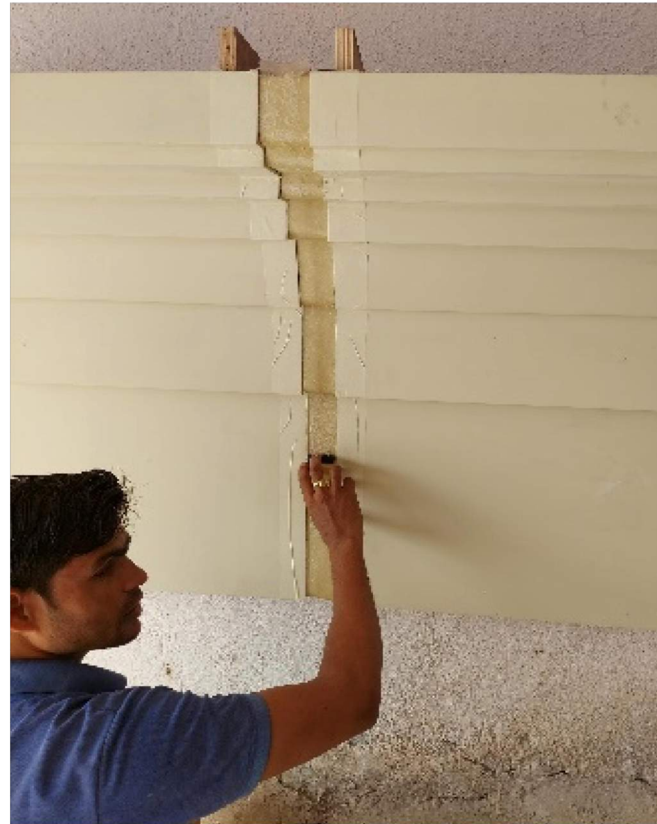
8. SAND TAPED JOINT
