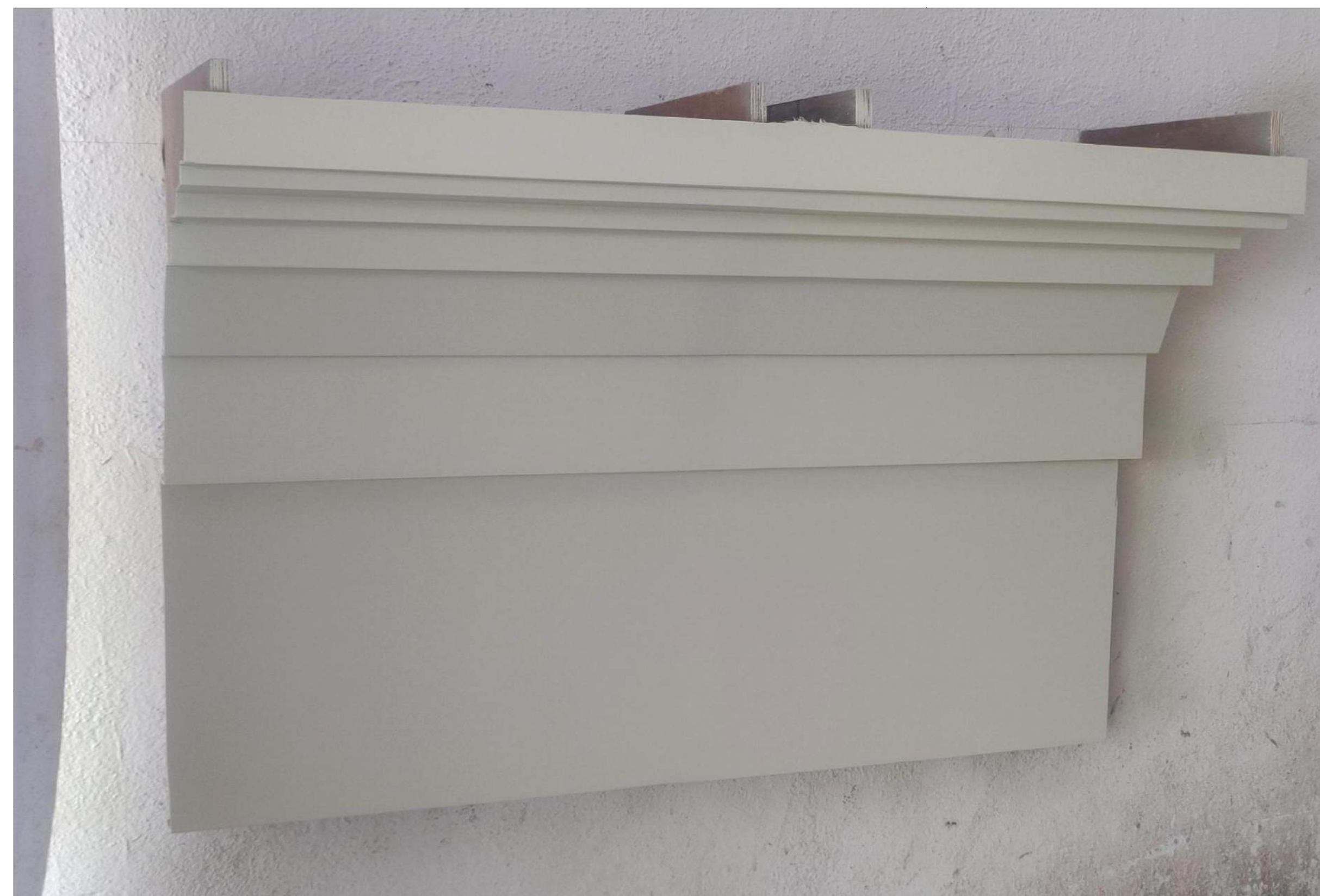
11. FIELD PAINT THE FINISHED CORNICE
