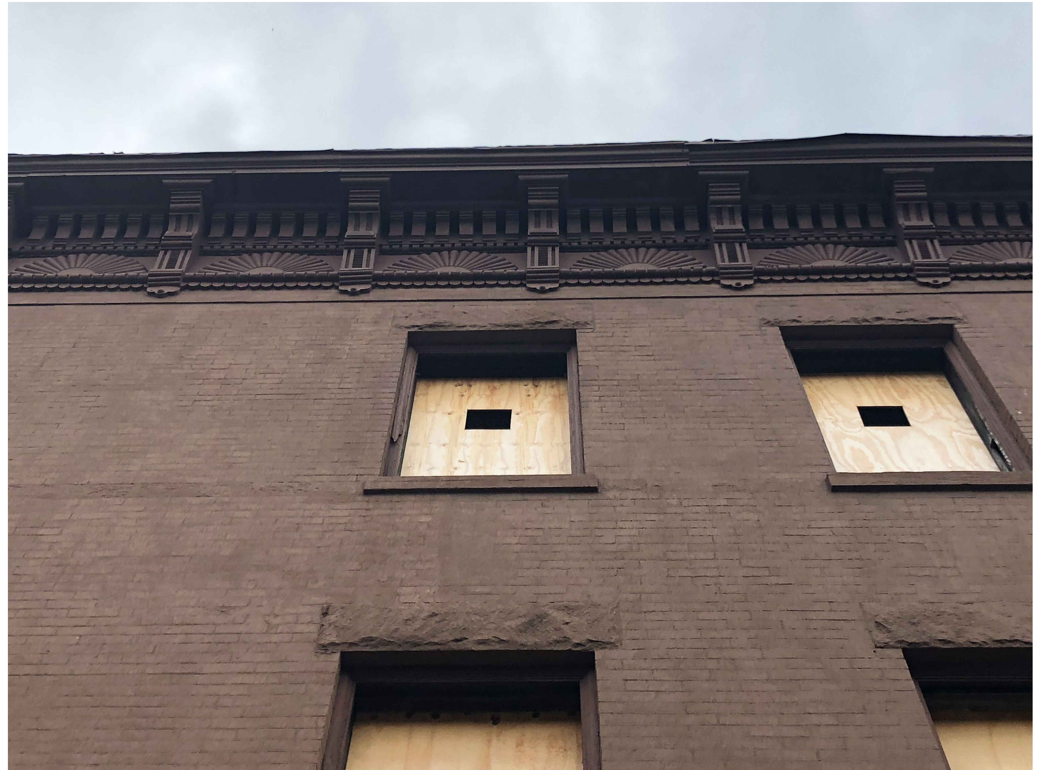
PRIOR TO CONSTRUCTION CORNICE PHOTO
