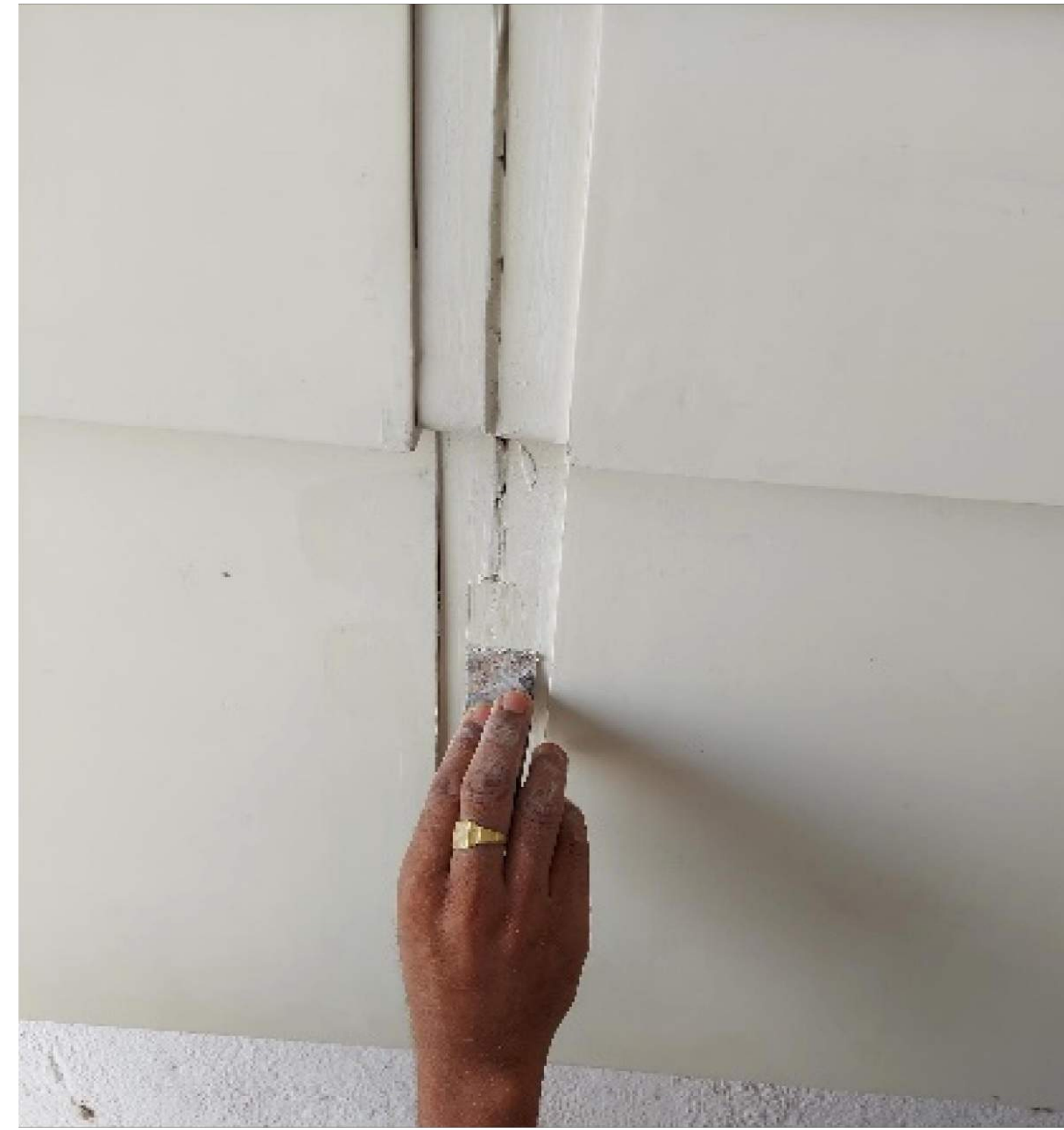
2. INFILL JOINT WITH PUTTY
