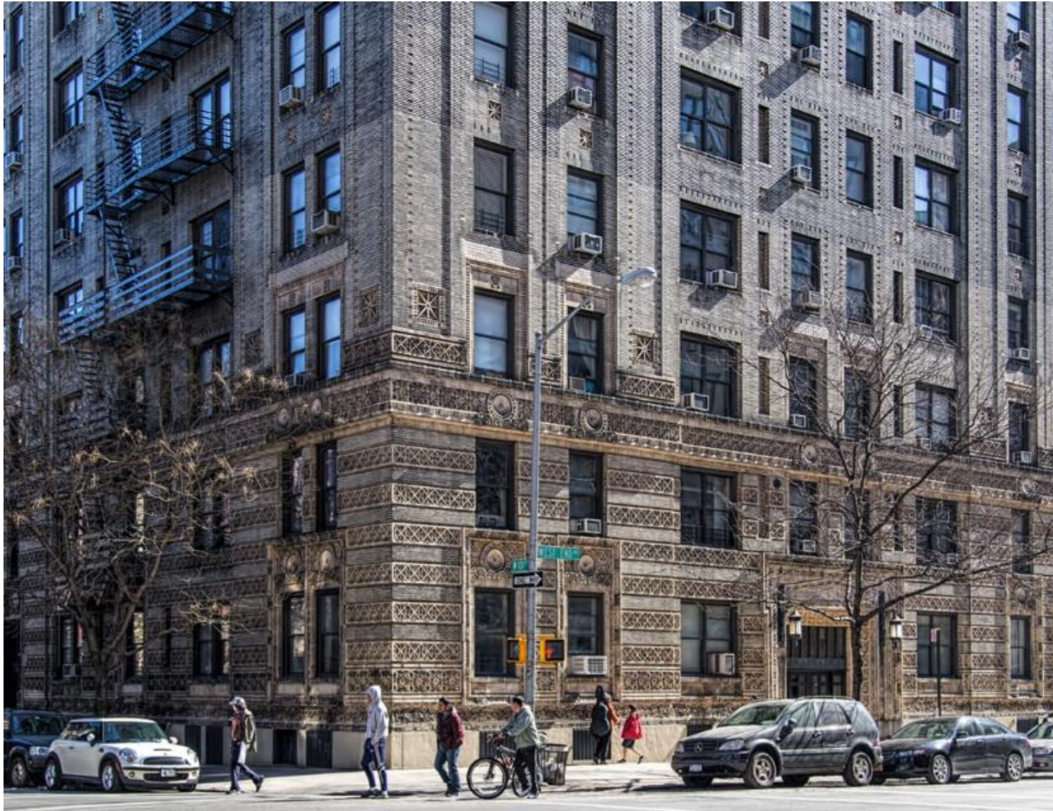
The Dallieu at 838 West End Avenue and 101 st Street (1912-13) is covered with rich geometric terra cotta panels.
