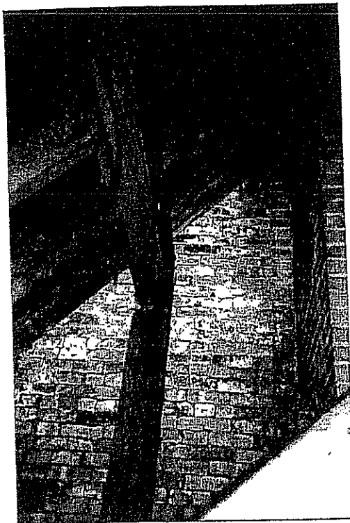
Photo 10: Water stains run down east masonry wall.
