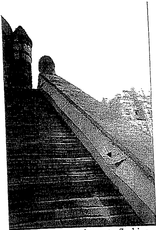
Photo 16: Damaged counterflashing.
