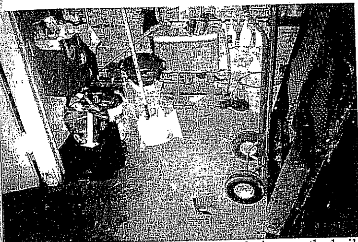
Photo M4: View of slop sink & floor drain near the boilers.
