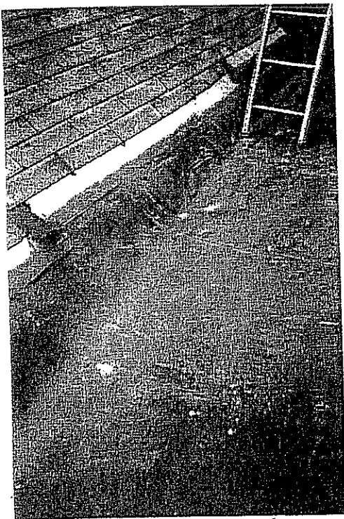
Photo 23: Warped roof membrane with soft spots at north gutter area.
