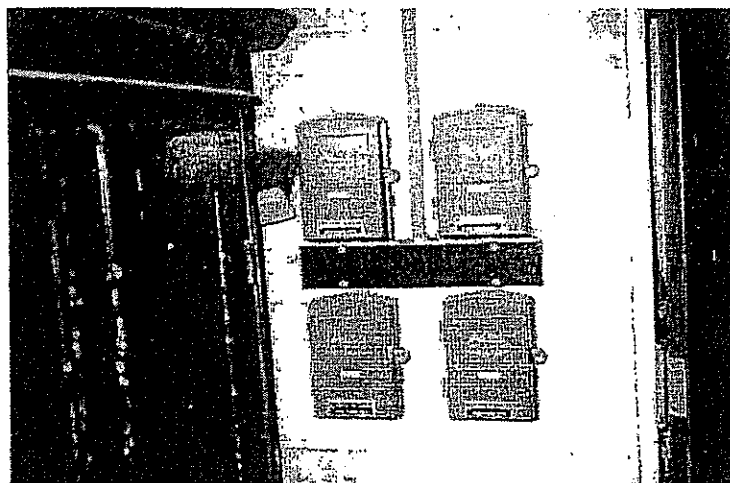
Photo M13: View of old alarm relays in basement.
