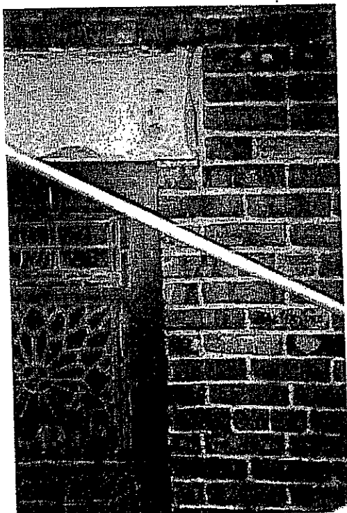
Photo 51: Cracks through masonry, running from head to sill.
