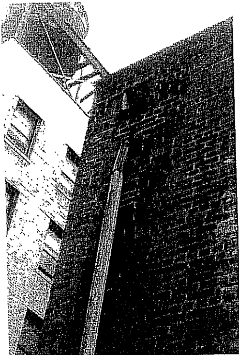
Photo 41: Leader and downspout no longer connected at northwest corner.
