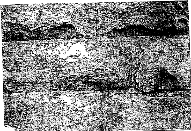
Photo 42: Deteriorated brownstone.
