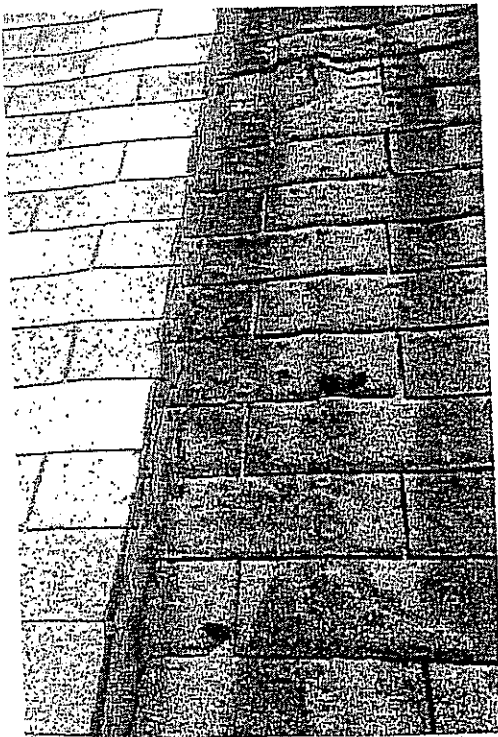
Photo 10: Water stains run down east masonry wall.
