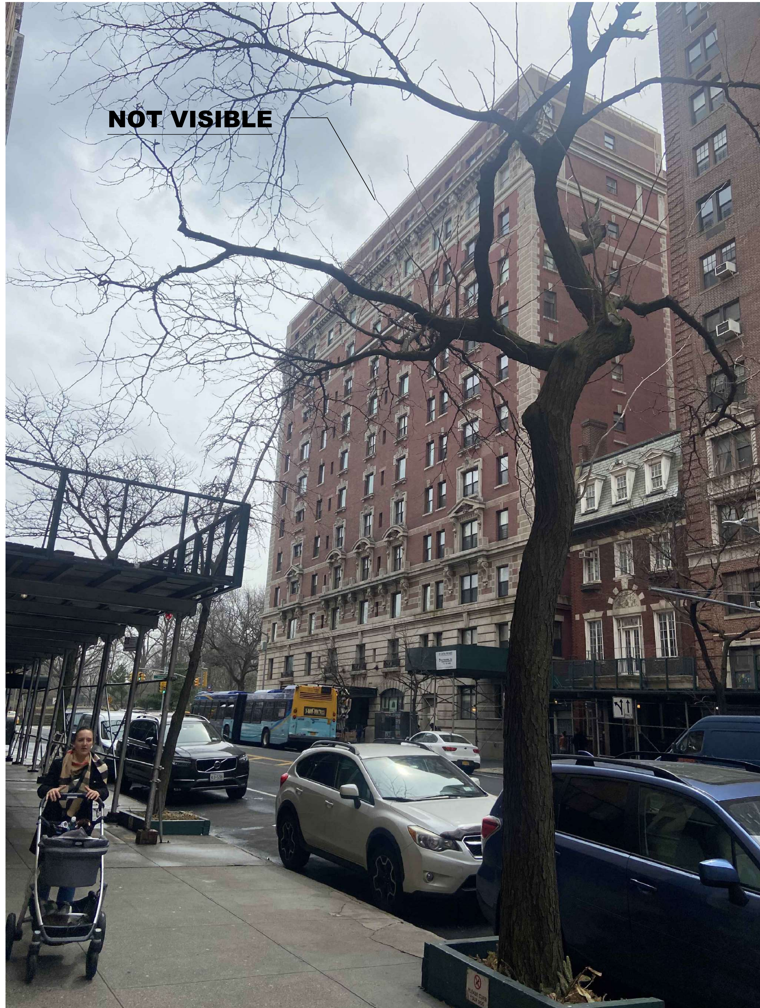
VIEW FROM 86TH STREET
