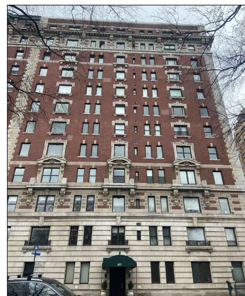
257 CPW BUILDING - VIEW A
