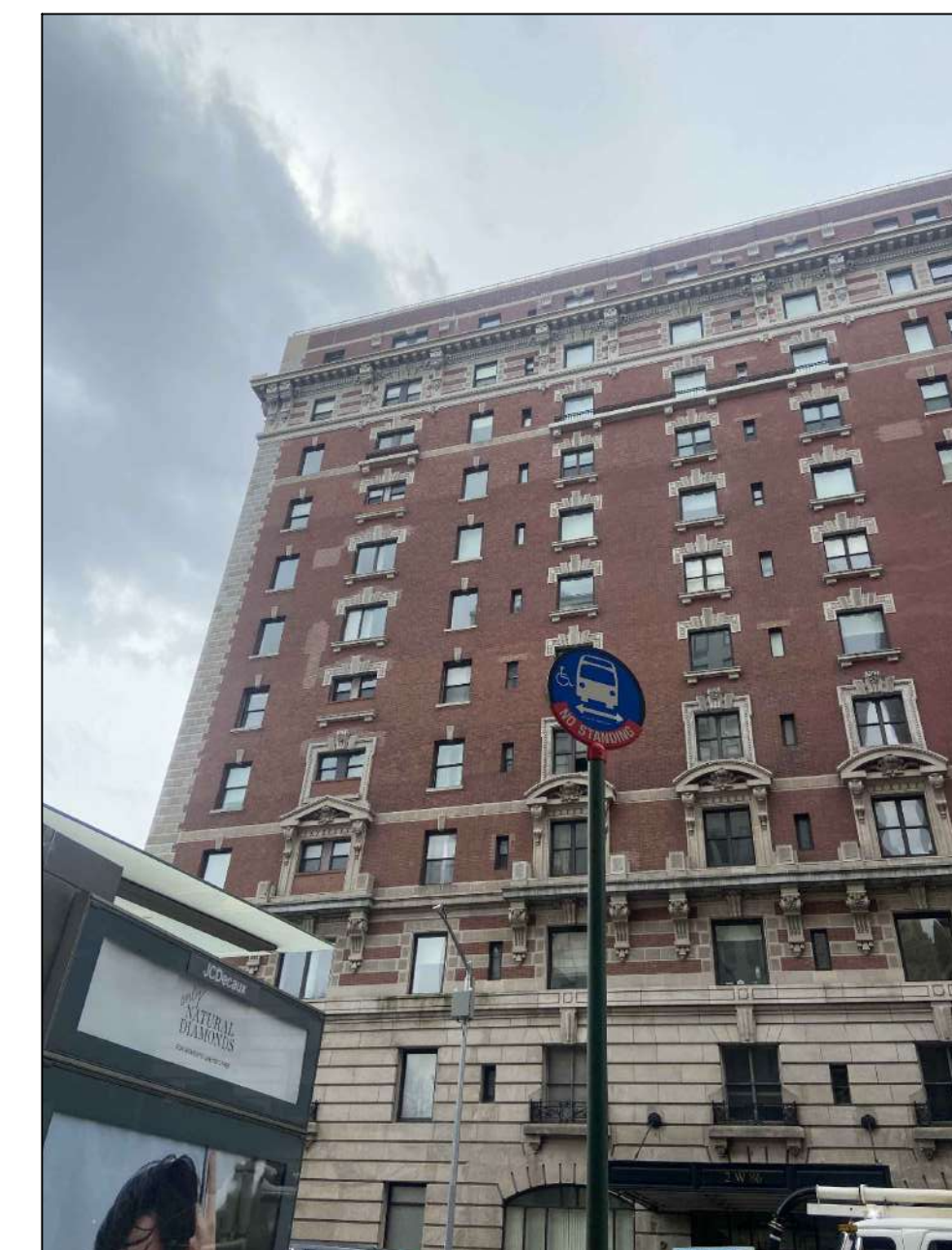
EXISTING PHOTO - 86TH STREET
