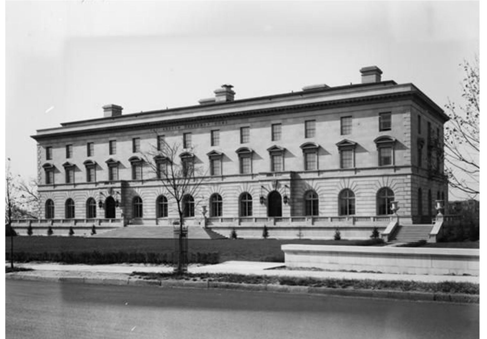
View from Grand Concourse. Prior to Addition of Wings. 1924.
