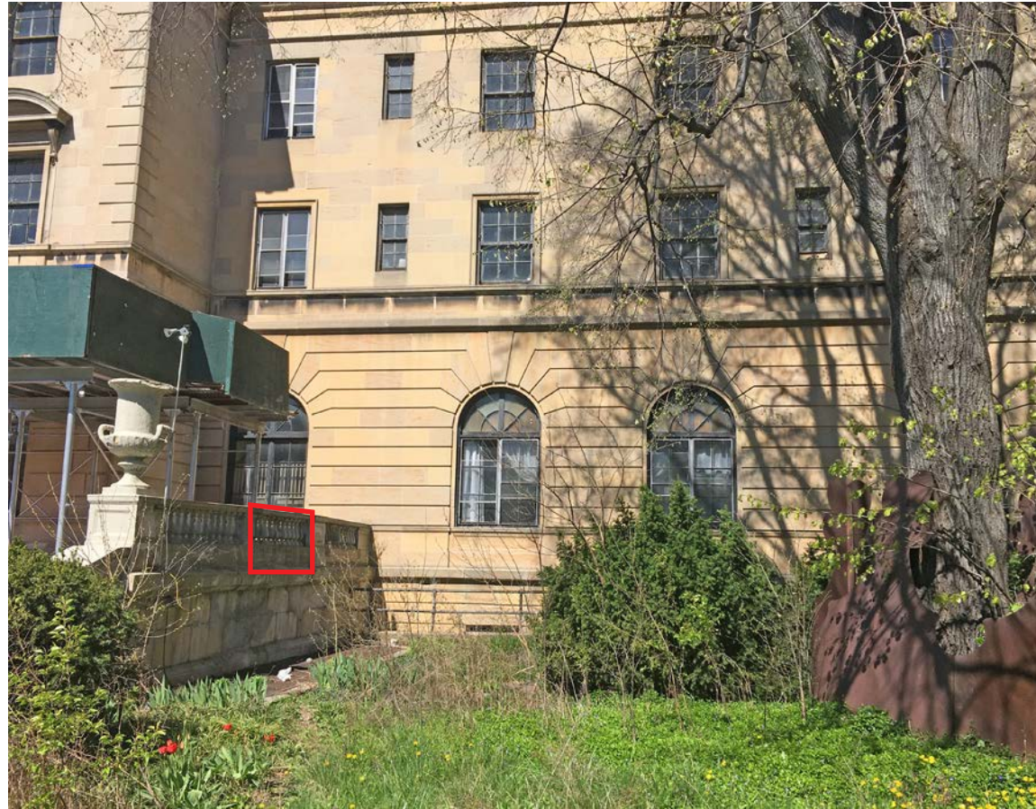
A. AREA PROPOSED FOR NEW ADA RAMP FROM FRONT LANDSCAPE
