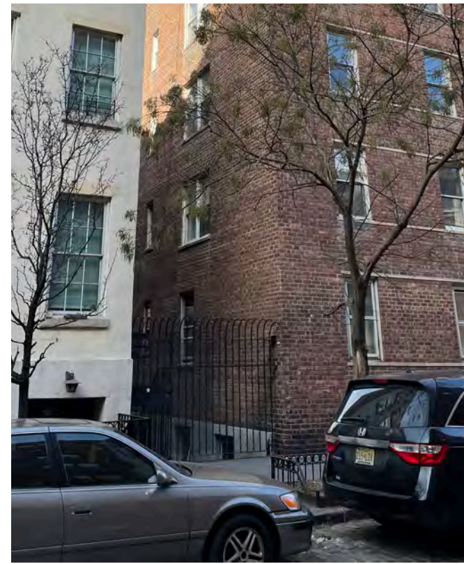
2. View of Existing 105 Alley fence
