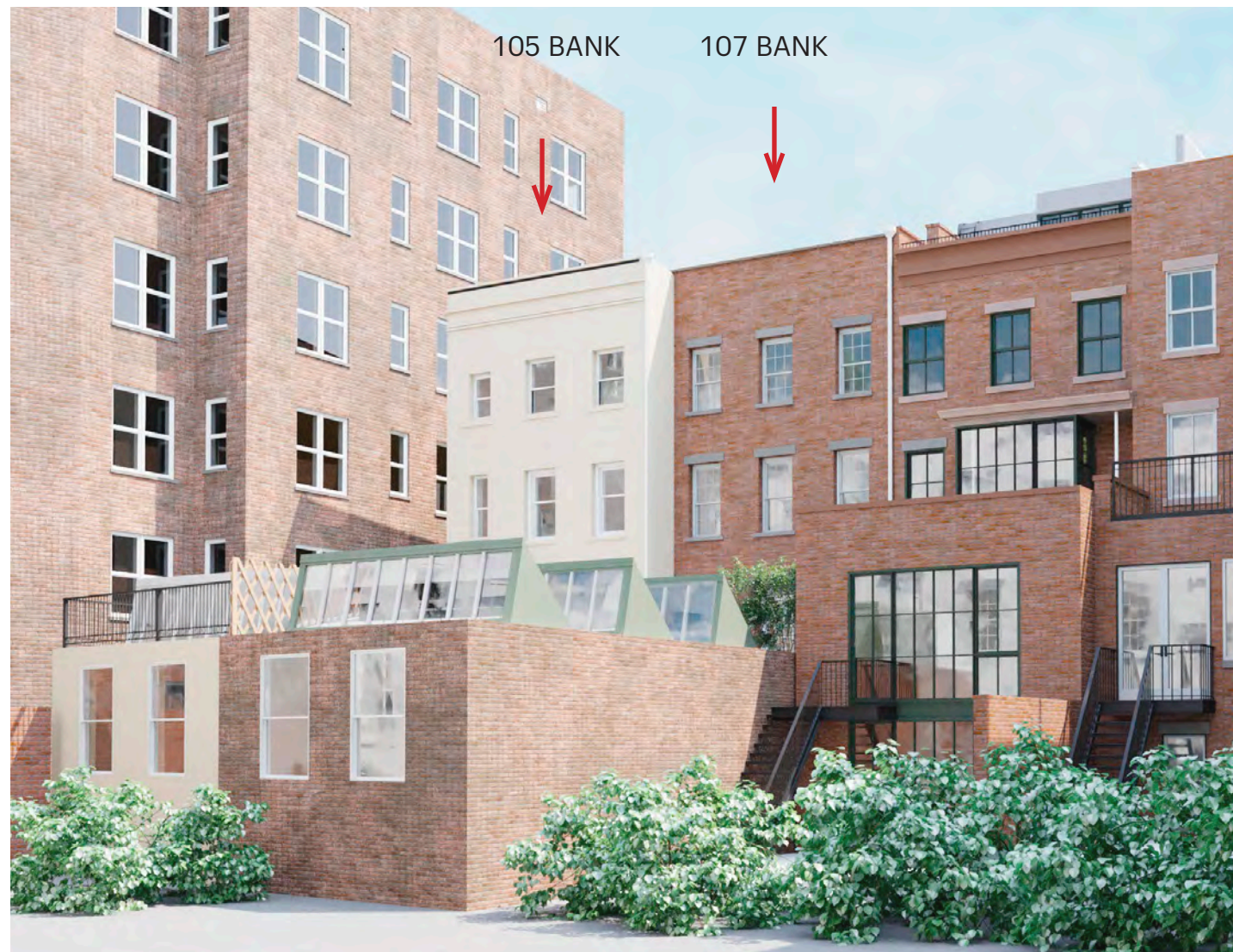
Existing rear of 105 and 107 Bank Street
