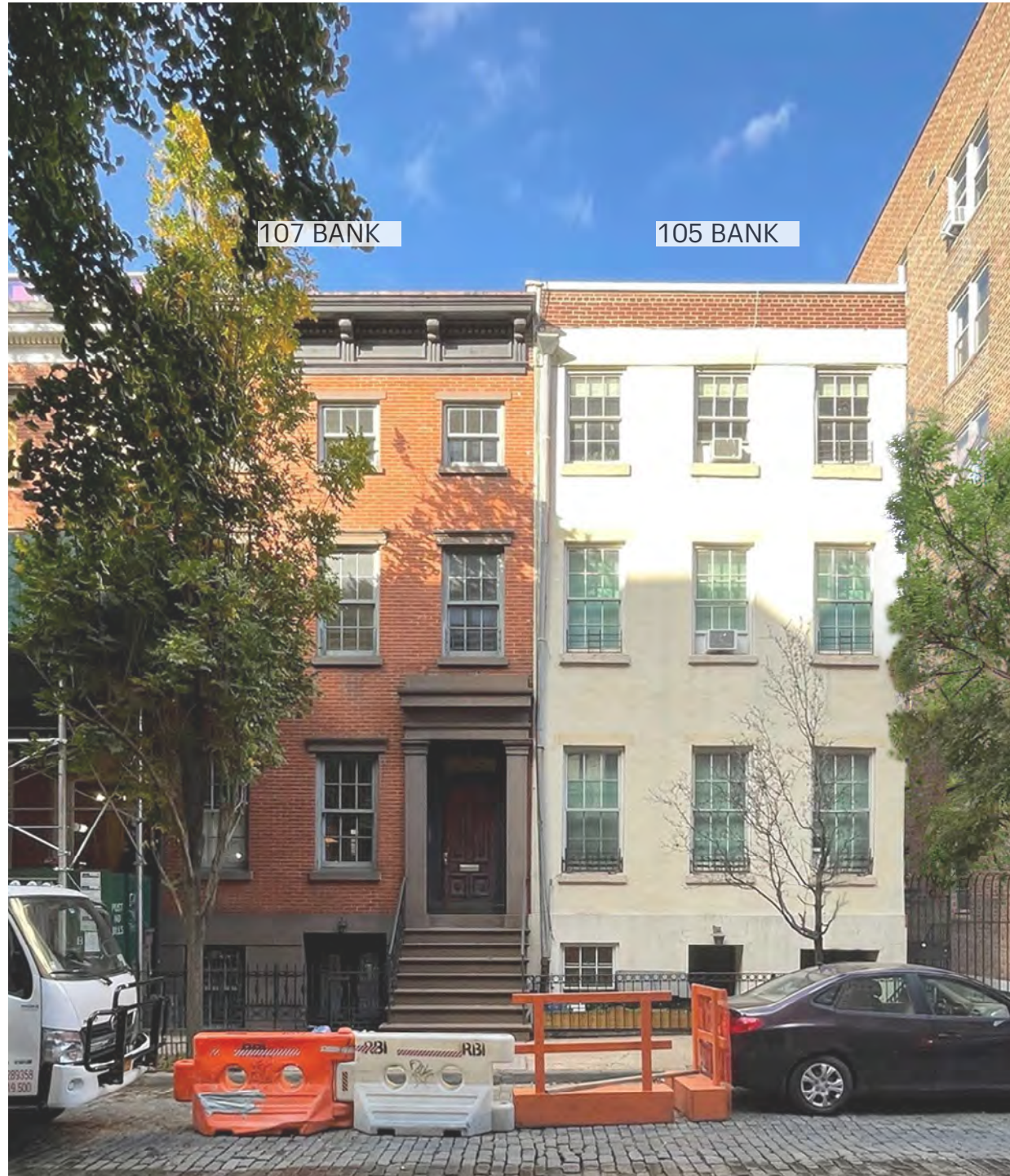
Existing 107 and 105 Bank
