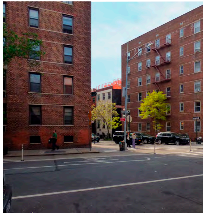
Visibility from Greenwich Ave. (5-5-22 Photo)
