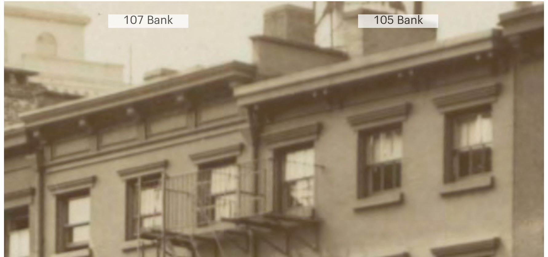
107 - 105 Bank historic cornice, 1932 (nypl)
