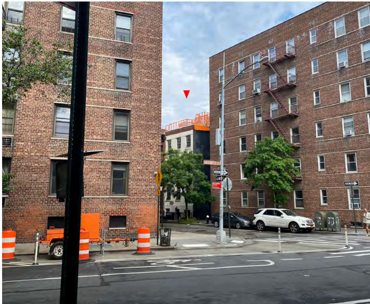
Visibility from Greenwich Ave. (6-1 Photo)
