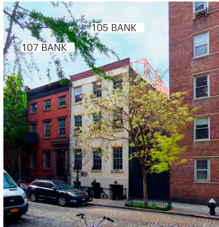
Visibility from Bank Street (5-5-22 Photo)
