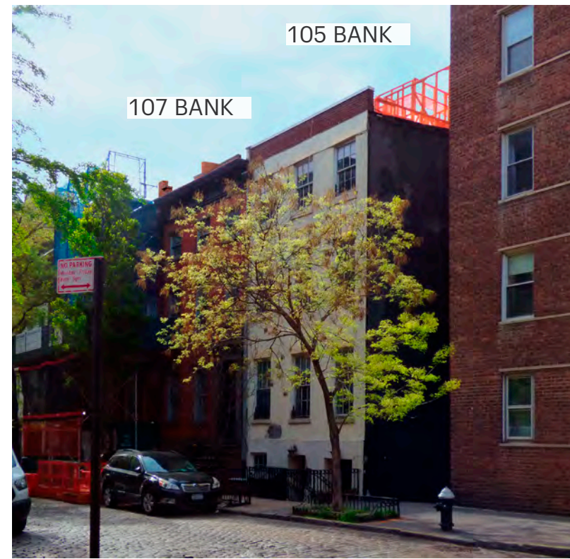
Visibility from Bank Street (5-5-22 Photo)
