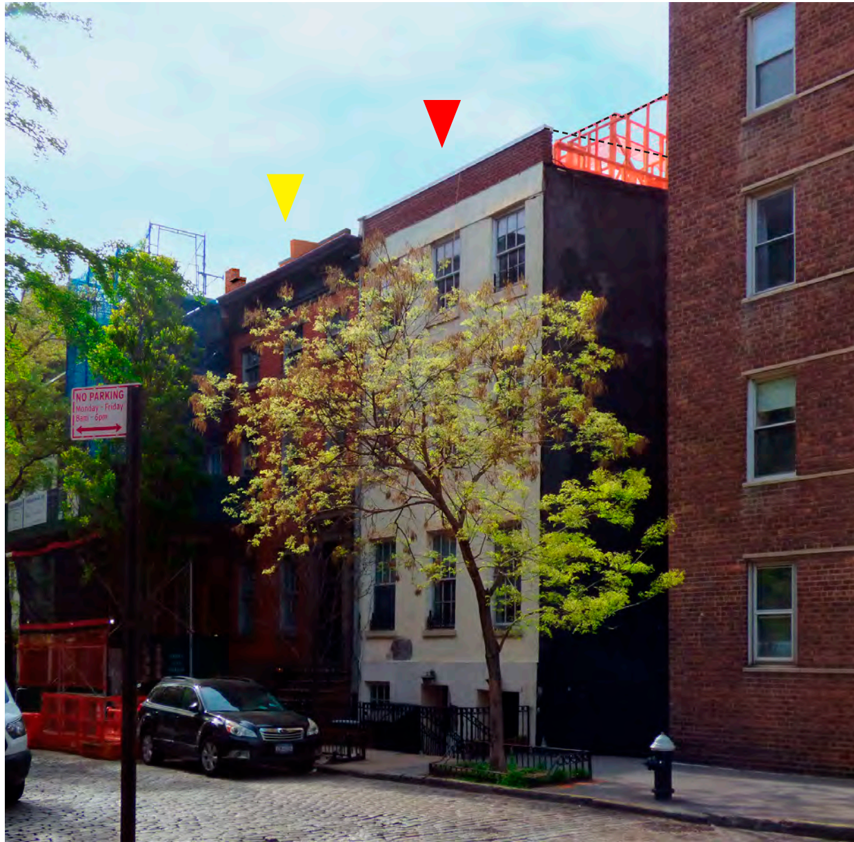
Visibility from Bank Street (5-5-22 Photo)
