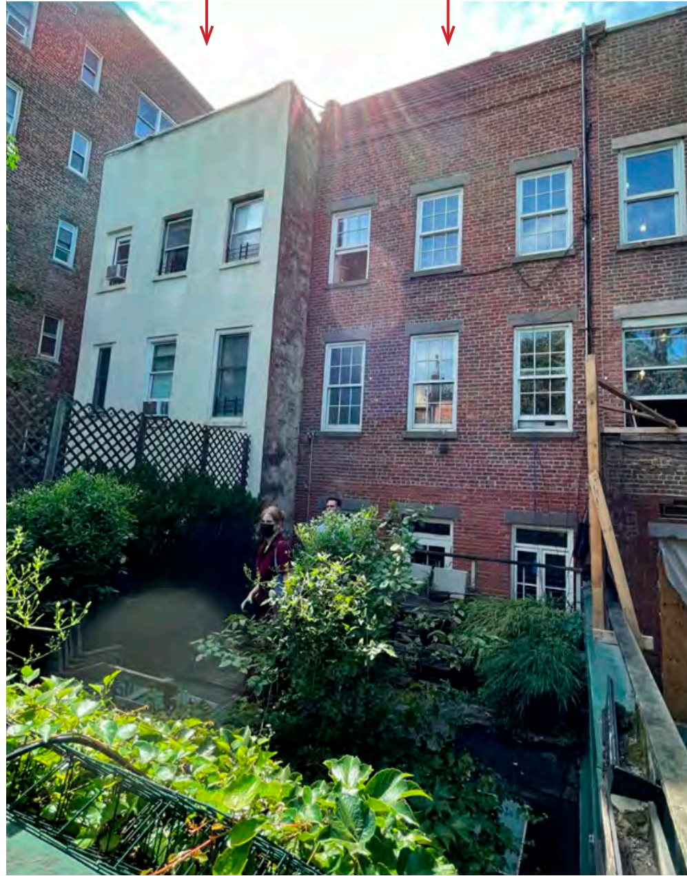
105 and 107 Bank - Current Rear Elevation
