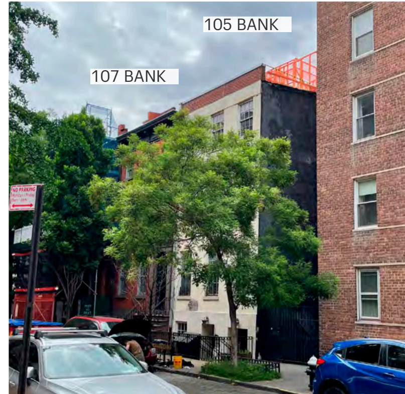
Visibility from Bank Street (5-26-22 Photo)
