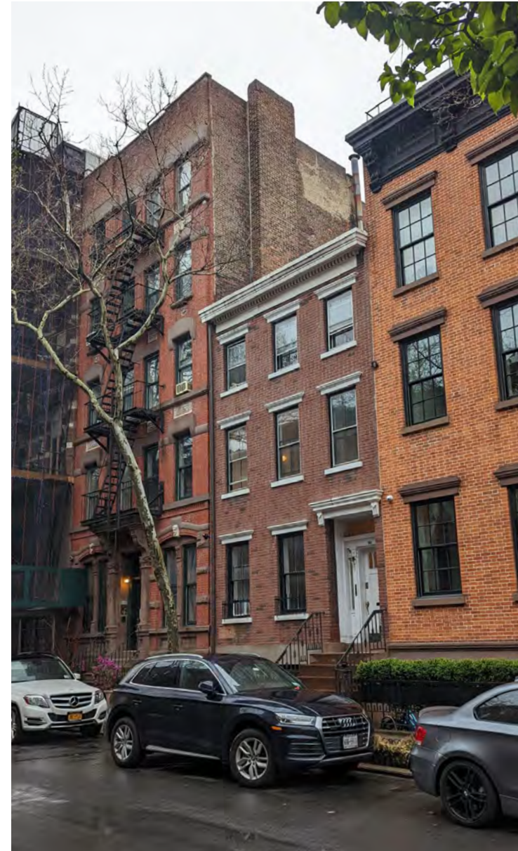
03. TO THE WEST OF 90 CHARLES STREET - FRONT FACADE (NORTH)
