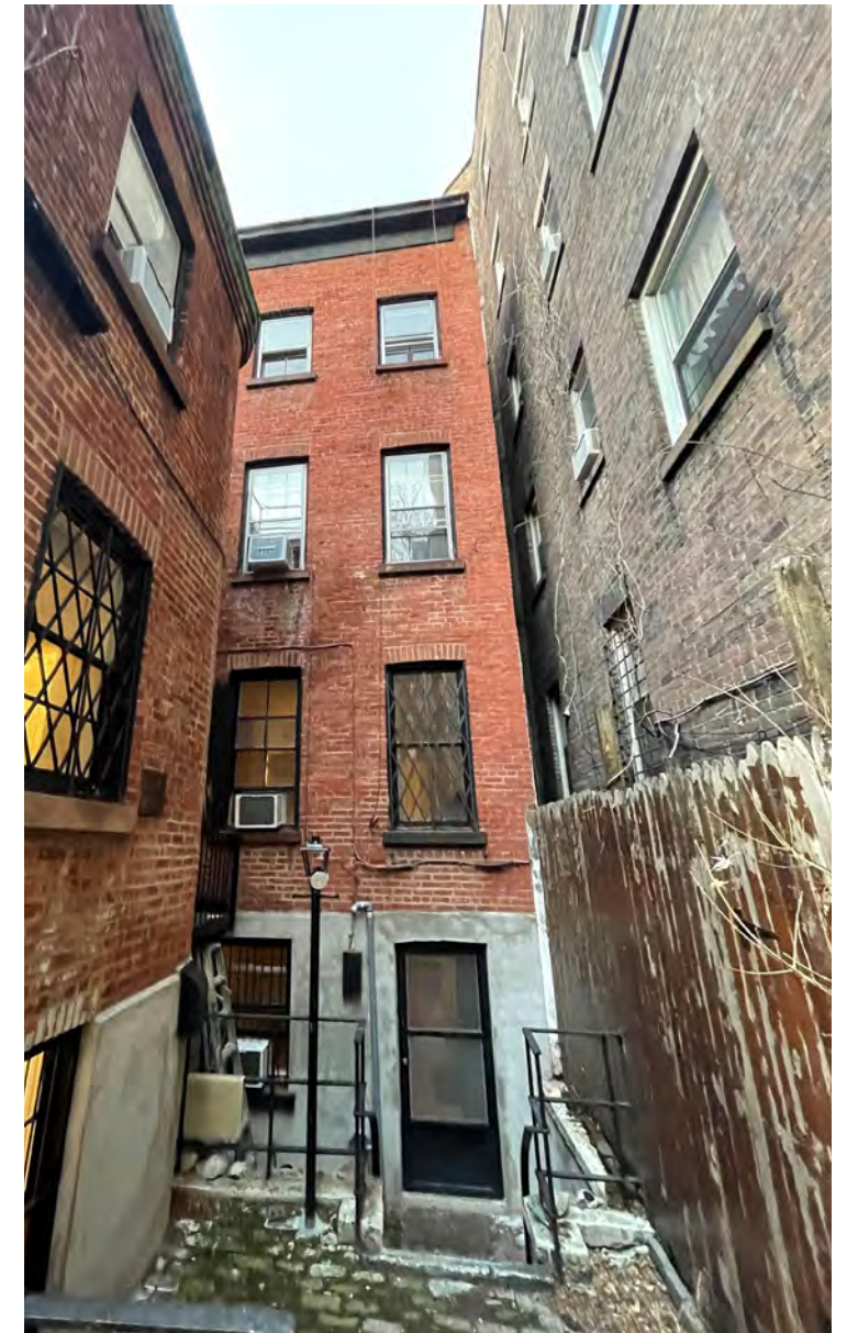
90 CHARLES STREET - REAR FACADE (SOUTH)
