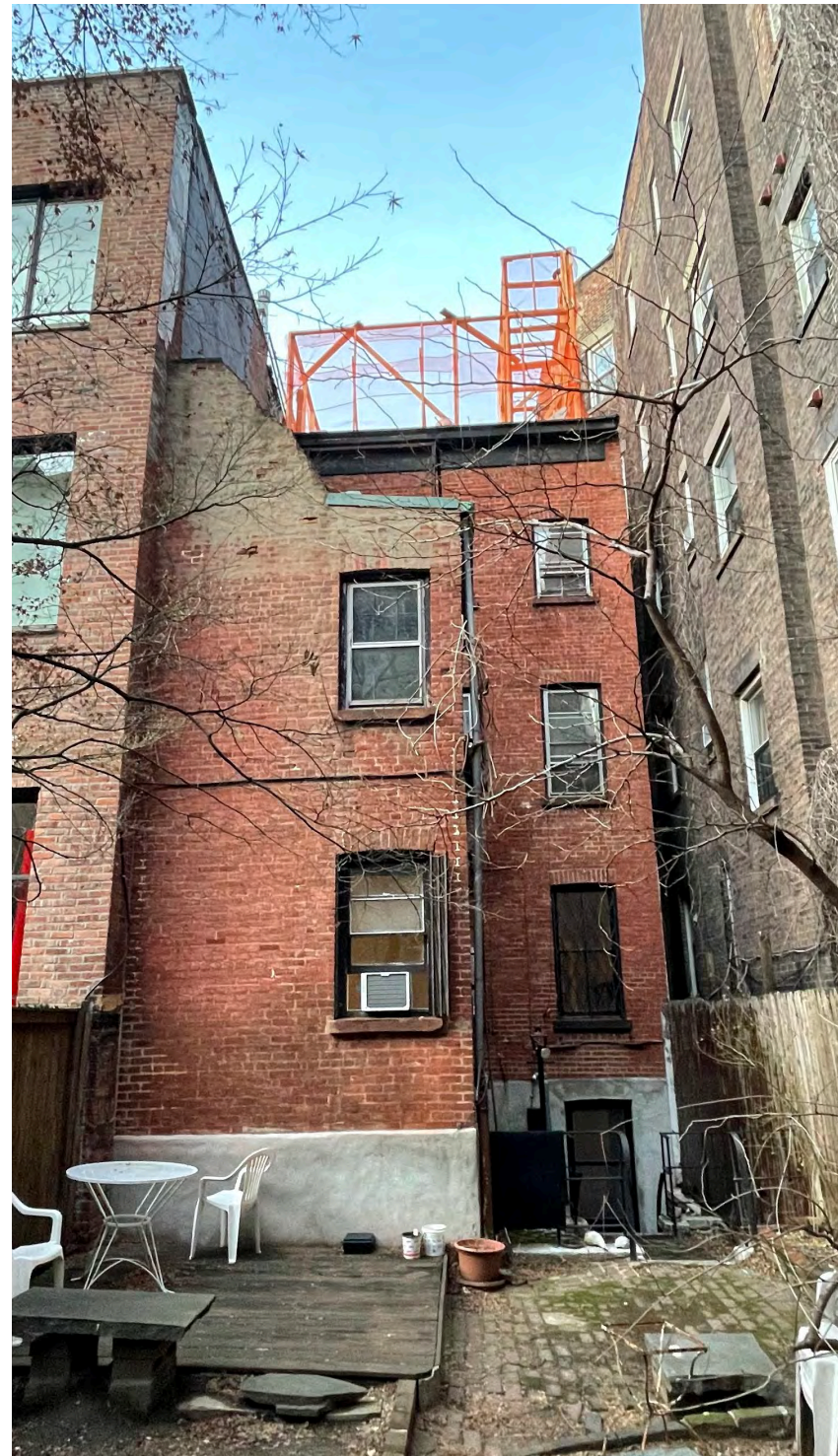
EXISTING REAR FACADE
