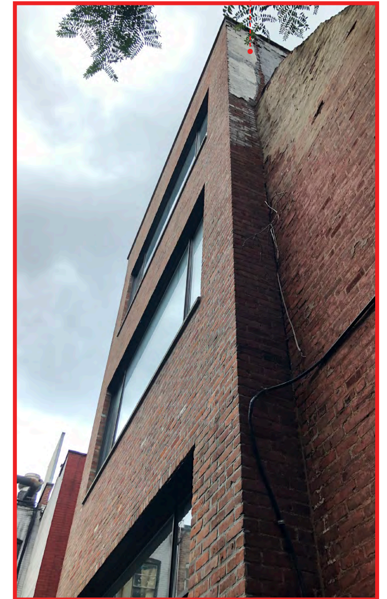
92 CHARLES STREET - REAR FACADE (SOUTH)
