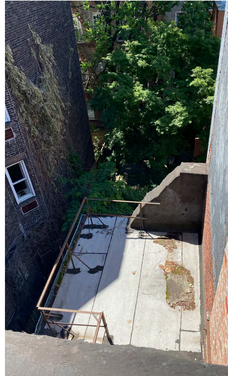
REAR YARD ADDITION FROM ROOF
