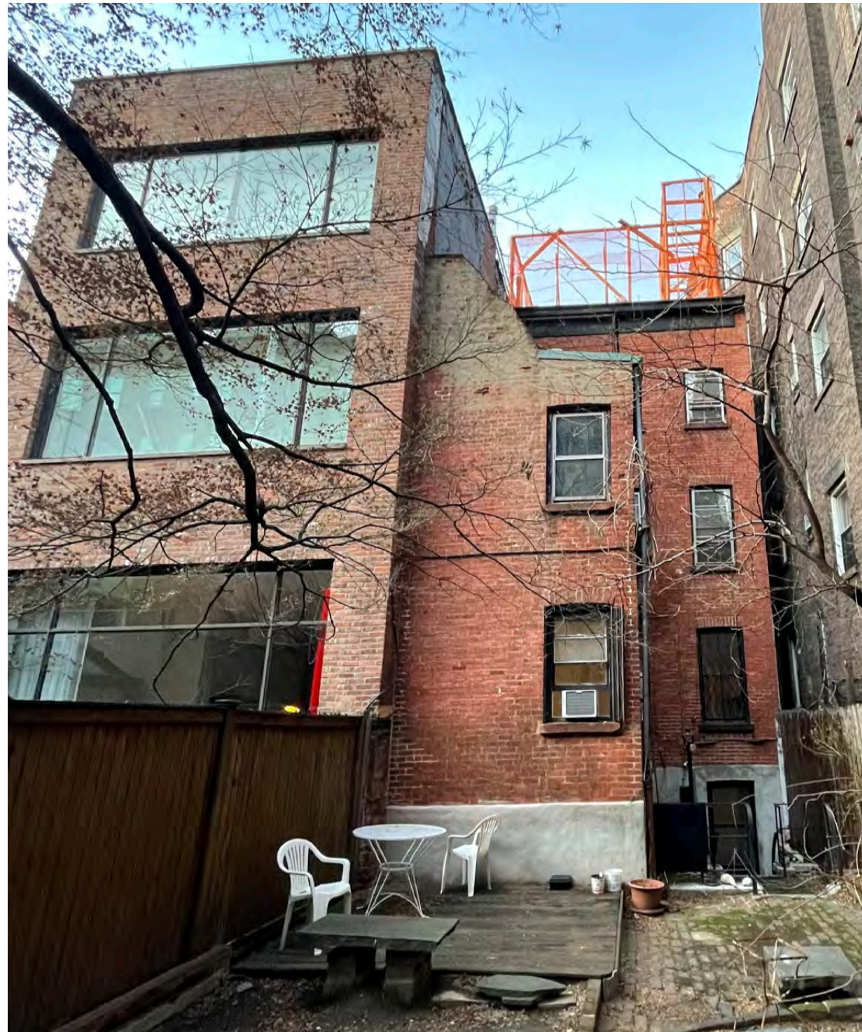
EXISTING REAR FACADE
