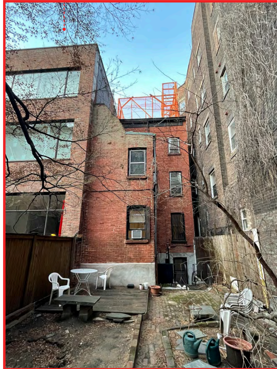
SOUTH FACADE AND YARD
