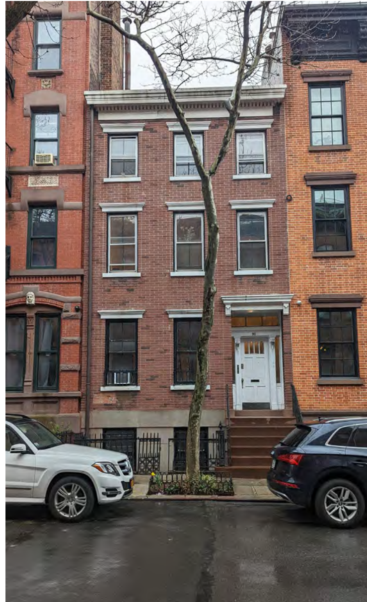
02. 90 CHARLES STREET - FRONT FACADE (NORTH)
