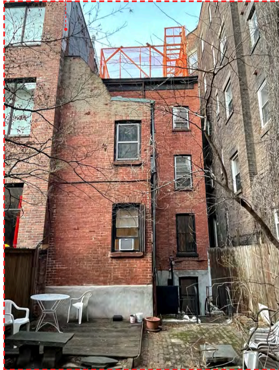
SOUTH FACADE AND YARD
