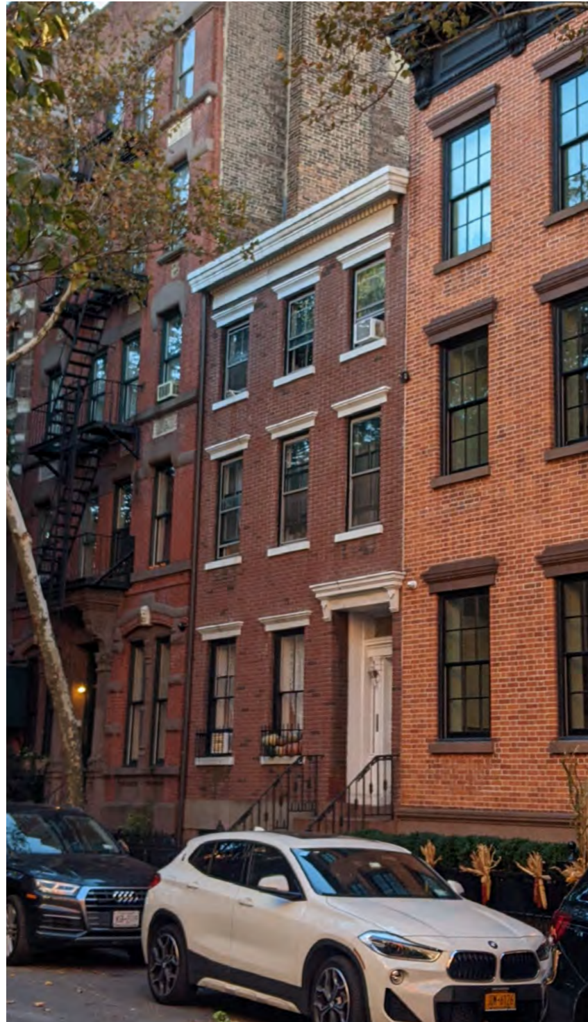
EXISTING FRONT FACADE
