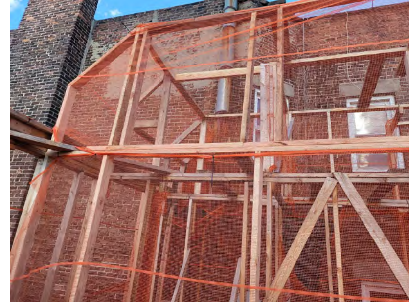
MECHANICAL BULKHEAD MOCK-UP
