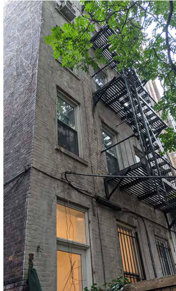
88 CHARLES REAR FACADE
