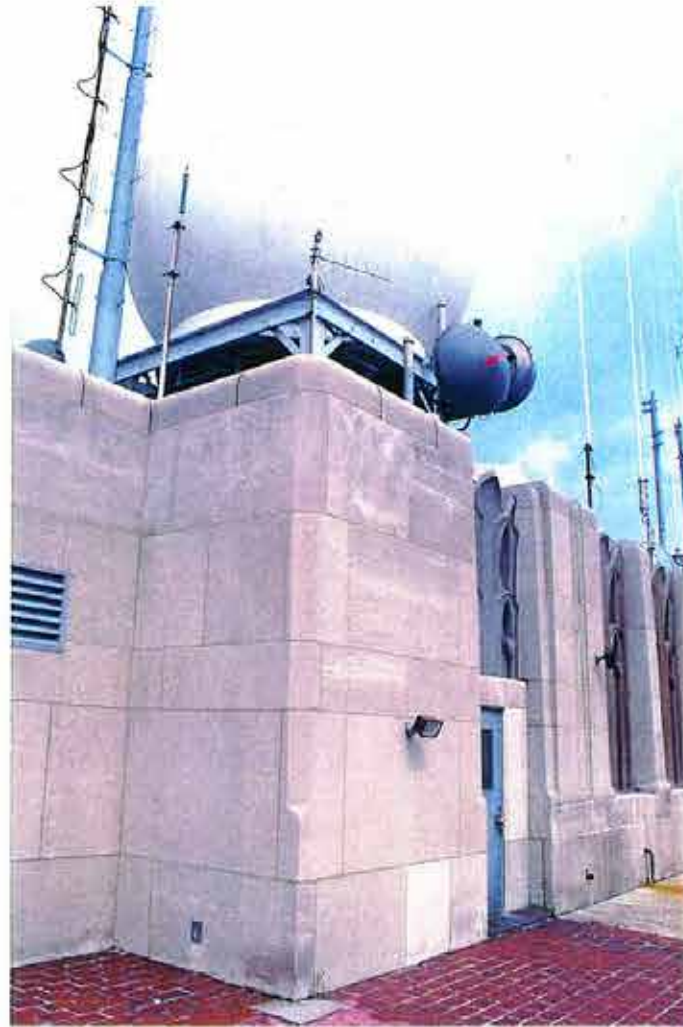
EXISTING WEST STAIR ENCLOSURE
