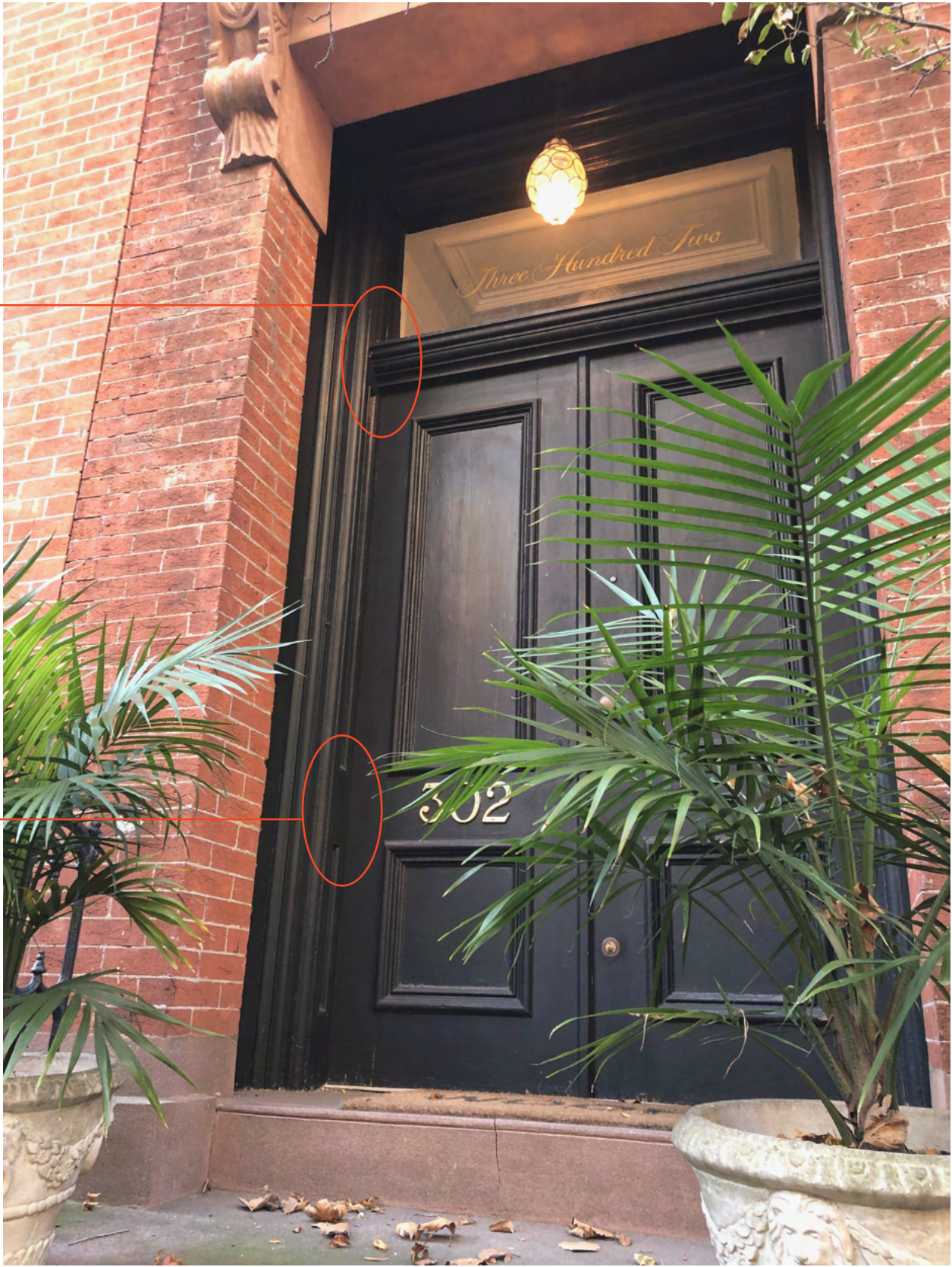
302 STATE STREET EXISTING PANELED ENTRY DOOR ENFRAMEMENT
