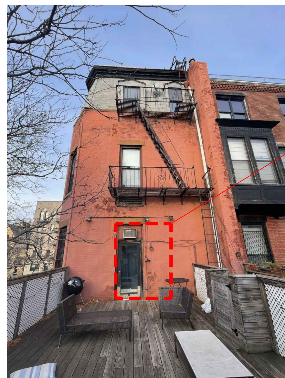
EXISTING SECONDARY FACADE PHOTO
