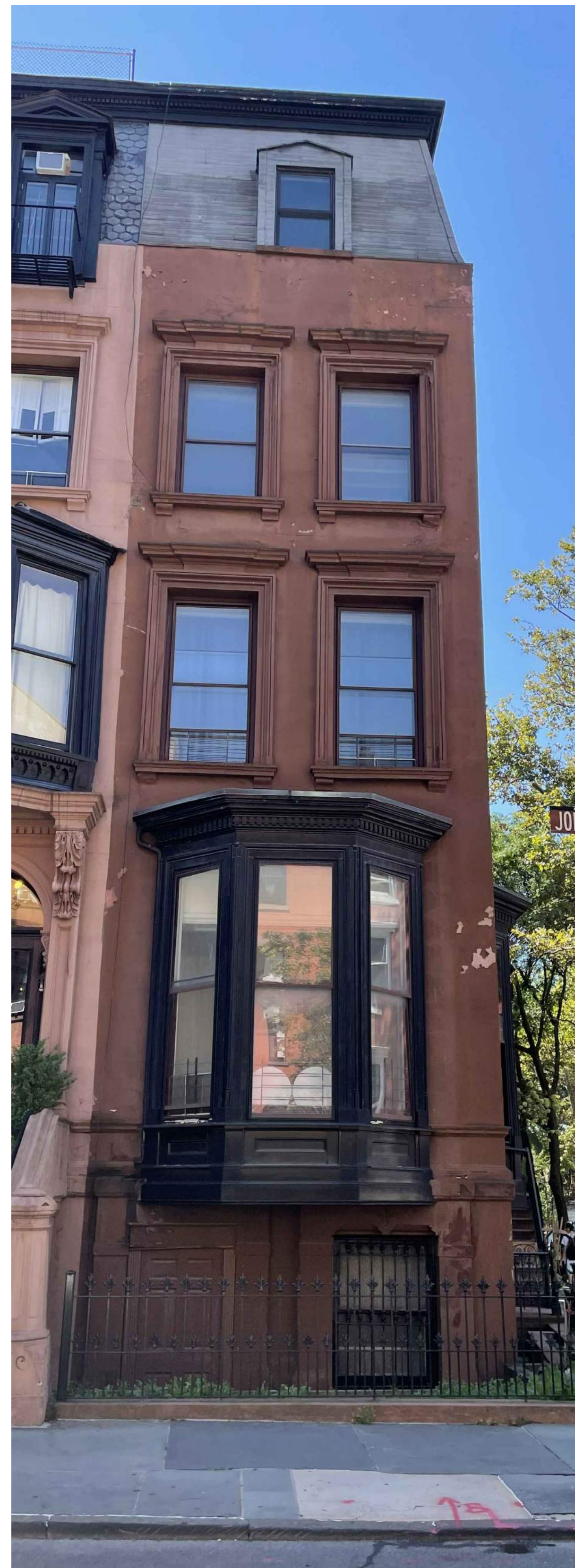
EXISTING JORALEMON ST ELEVATION PHOTO
