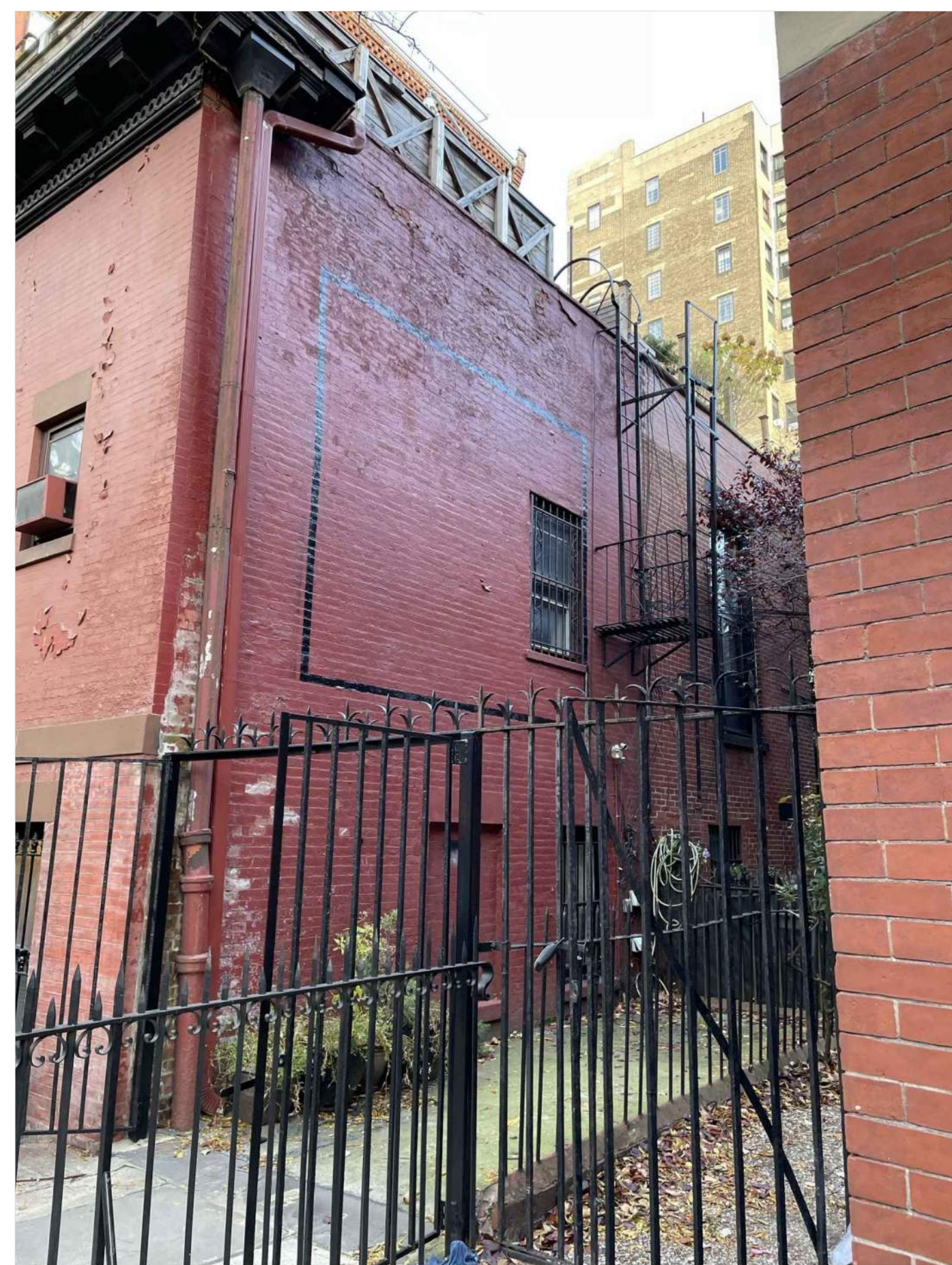
EXISTING PARKING SPACE PHOTO
