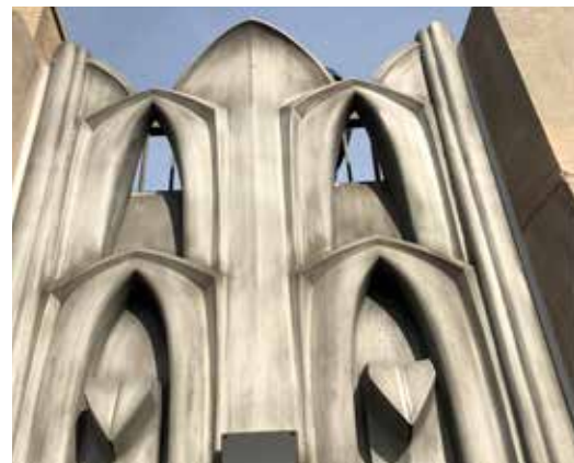
Existing cast metal panels (match)
