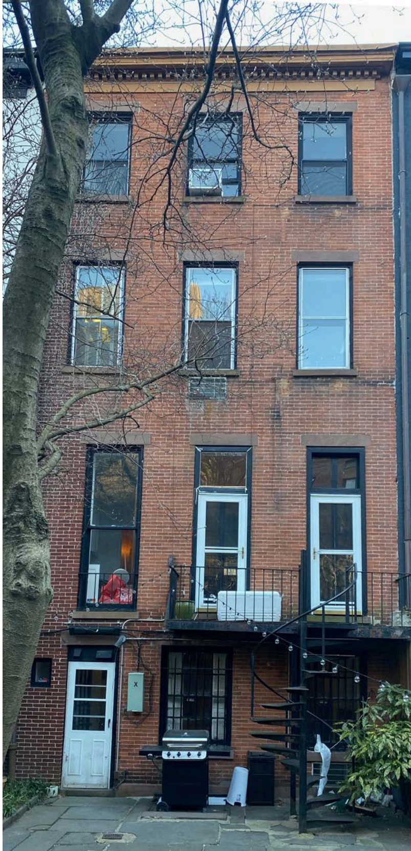
EXISTING REAR FACADE - 9 SLP
