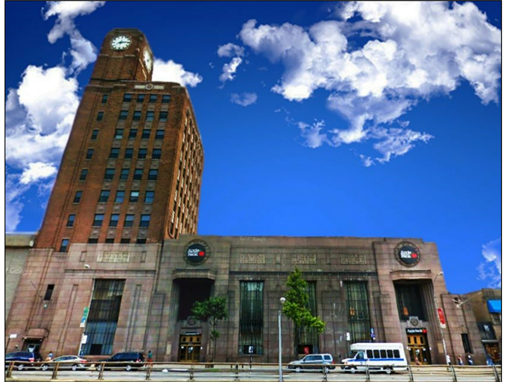
RECENT PHOTO (FORMER APPLE BANK)
