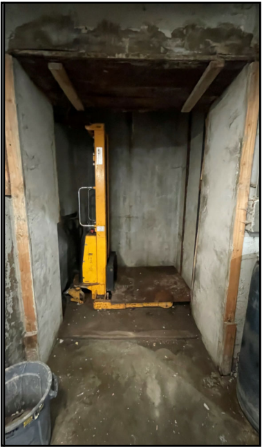
CELLAR EXISTING LOADING ROOM
