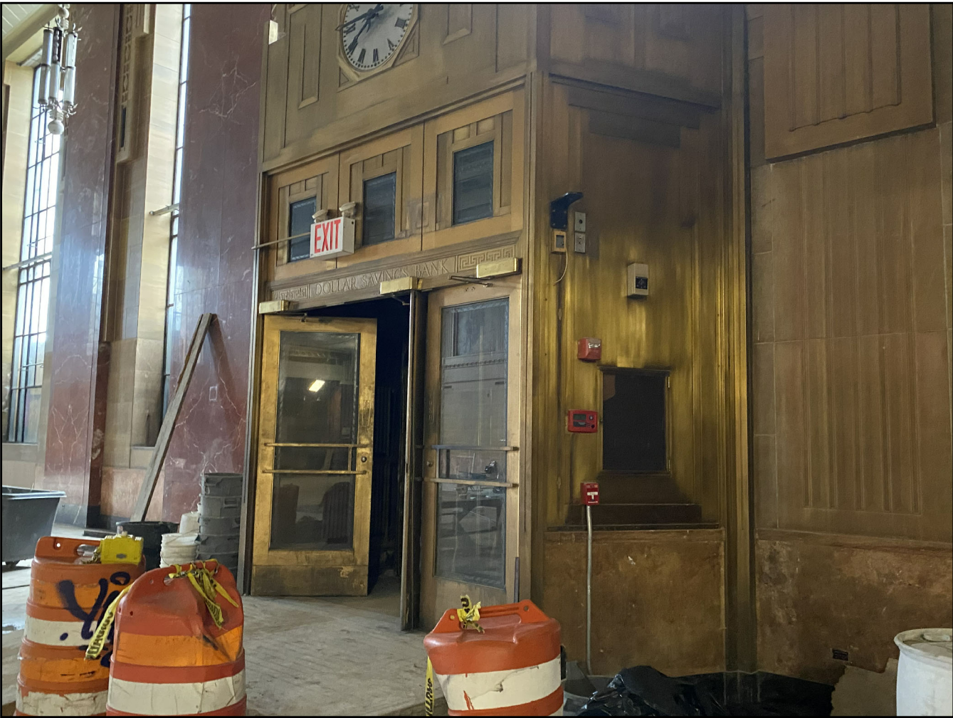
EXISTING NORTH VESTIBULE PHOTO
