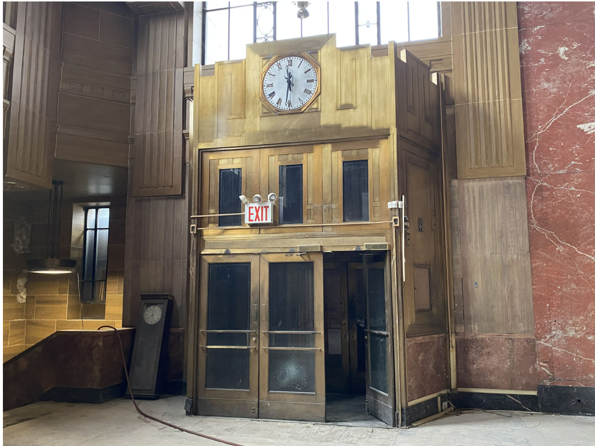
EXISTING SOUTH ENTRANCE VESTIBULE
