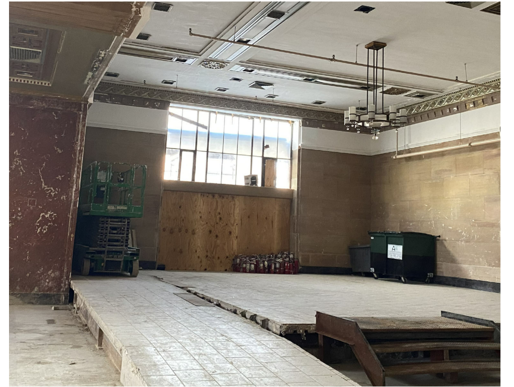
EXISTING INTERIOR ELEVATION 2021
