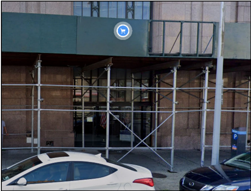
EXISTING NORTH ENTRY
