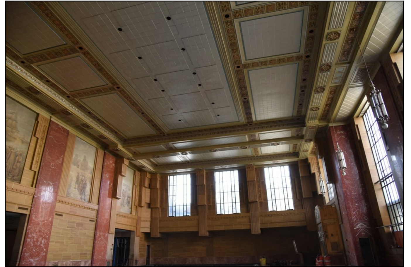
EXISTING INTERIOR PHOTO
