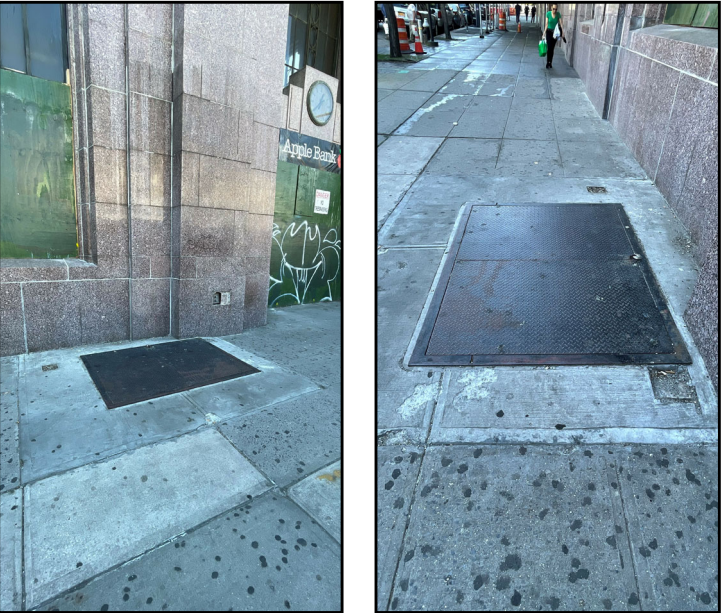
1ST FL. EXISTING LOADING HATCH
