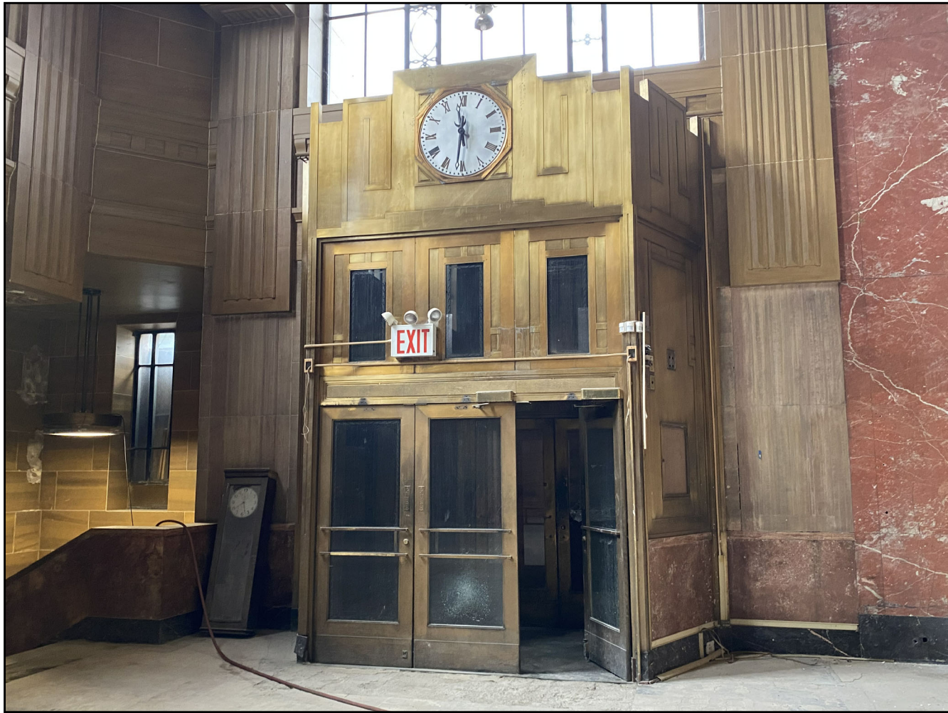
EXISTING SOUTH VESTIBULE PHOTO
