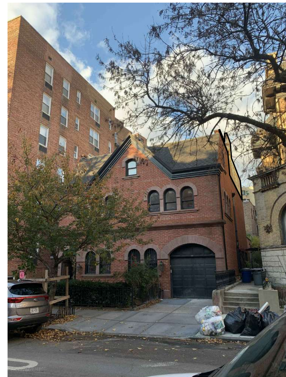
F VISIBILITY PHOTO FROM F (122 JORALEMON) LPC-5 SCALE: N.T.S. (PARAPET & CHIMNEY VISIBLE)
