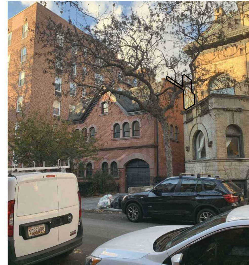
D VISIBILITY PHOTO FROM D (126 JORALEMON) LPC-6 SCALE: N.T.S. (PARAPET & CHIMNEY VISIBLE)
