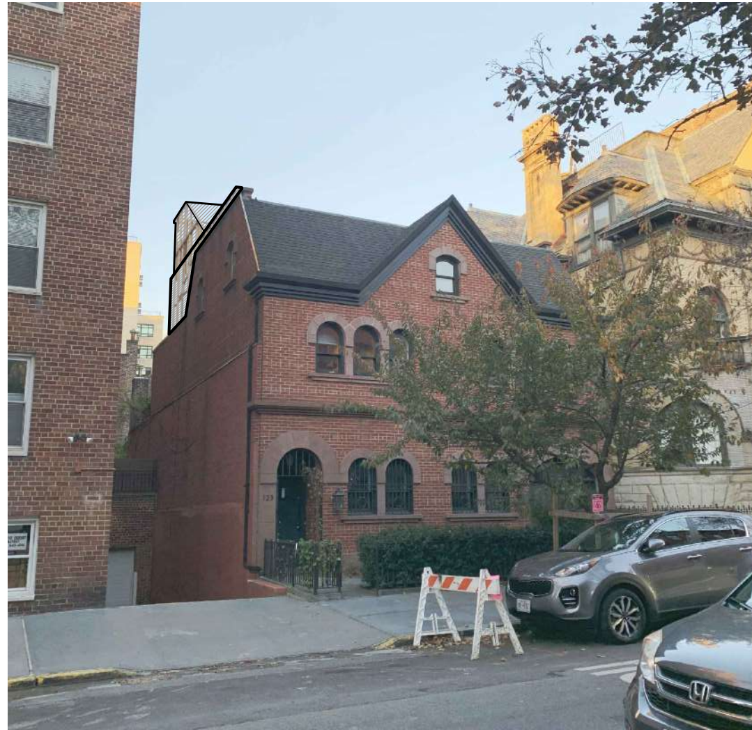
H VISIBILITY PHOTO FROM G (118 JORALEMON) LPC-6 SCALE: N.T.S. (PARAPET & BULKHEAD VISIBLE)
