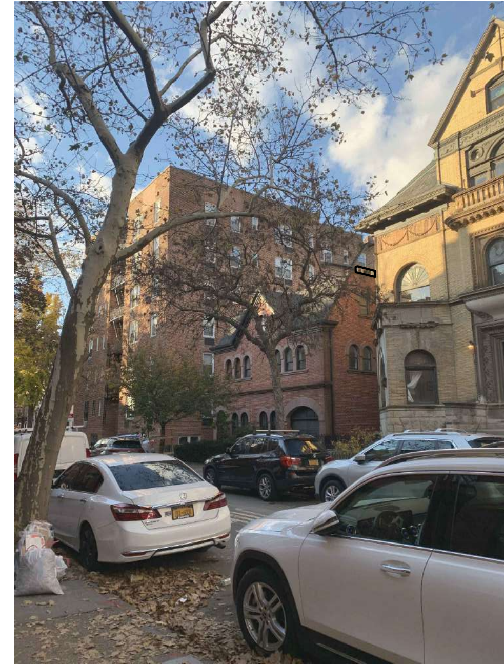
C VISIBILITY PHOTO FROM C (128 JORALEMON) LPC-5 SCALE: N.T.S. (PARAPET VISIBLE)
