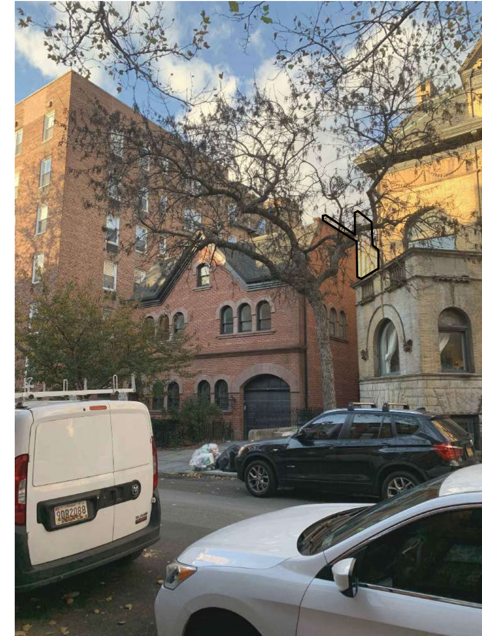
D VISIBILITY PHOTO FROM D (126 JORALEMON) LPC-5 SCALE: N.T.S. (PARAPET & CHIMNEY VISIBLE)
