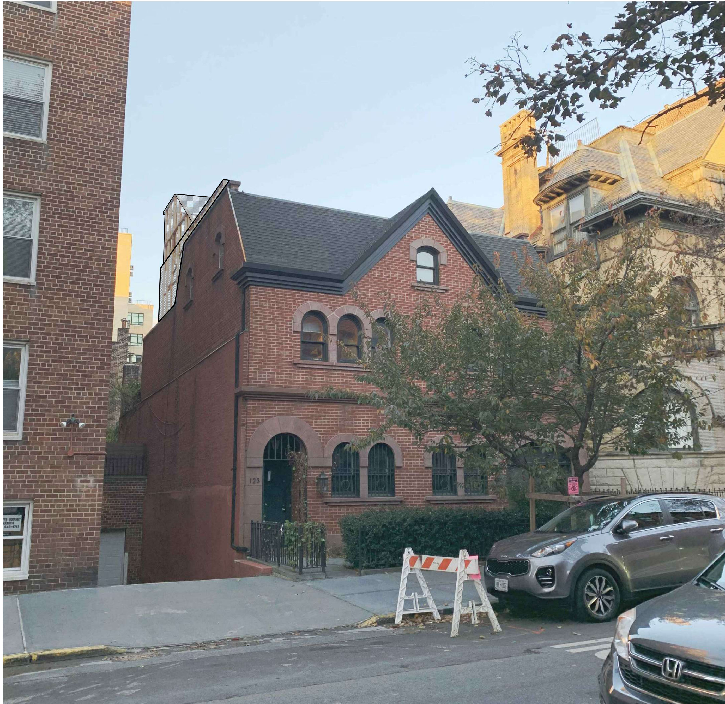
H VISIBILITY PHOTO FROM G (118 JORALEMON) - CLOSE UP LPC-6 SCALE: N.T.S. (PARAPET & BULKHEAD VISIBLE)
