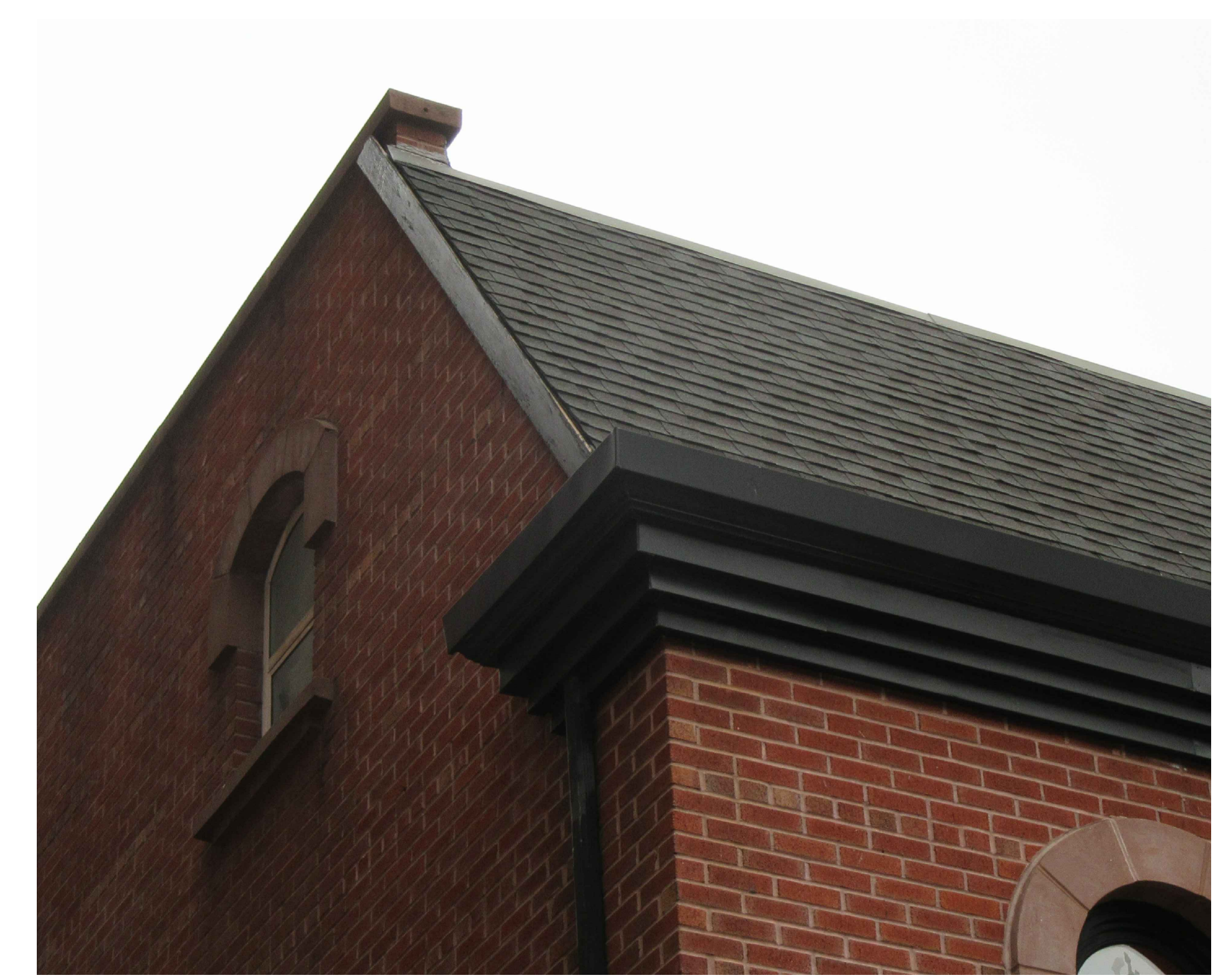
4 EXISTING FRONT ROOF PHOTO SCALE: NOT TO SCALE
