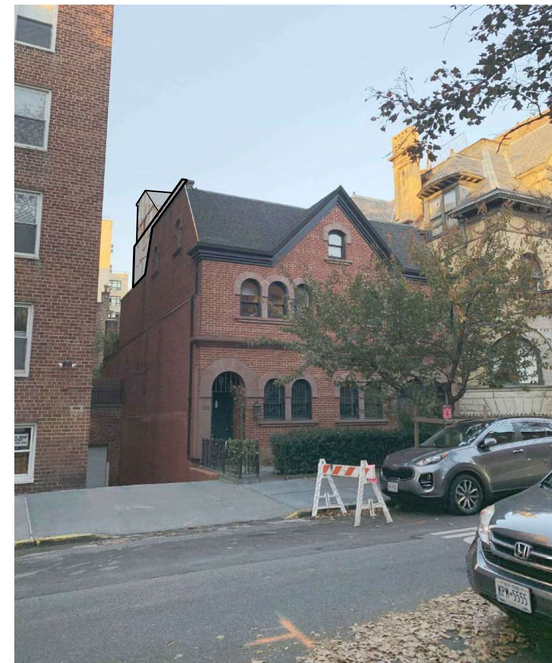
H VISIBILITY PHOTO FROM G (118 JORALEMON) LPC-5 SCALE: N.T.S. (PARAPET & BULKHEAD VISIBLE)
