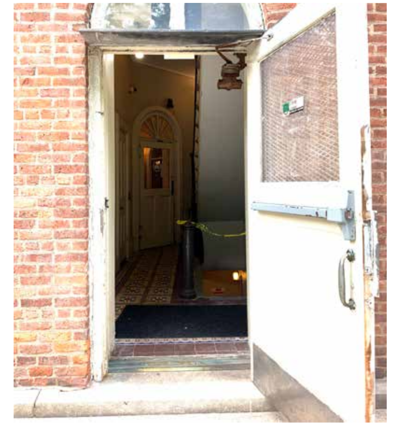
EXTERIOR DOOR AT REAR ENTRY
