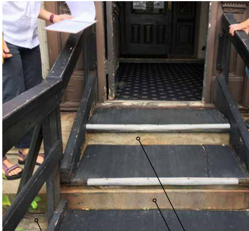
5 Door sill must be removed and door reversed to meet code
