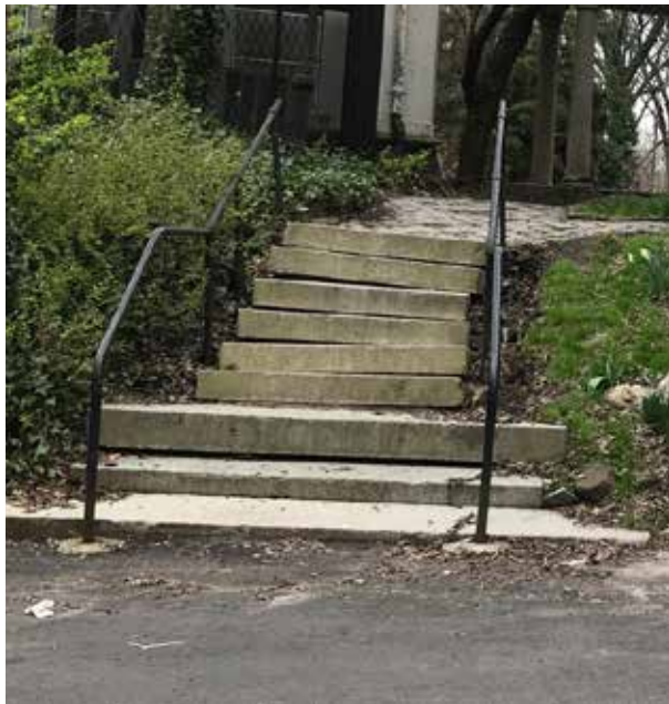
Painted pipe rail in rear of building.
