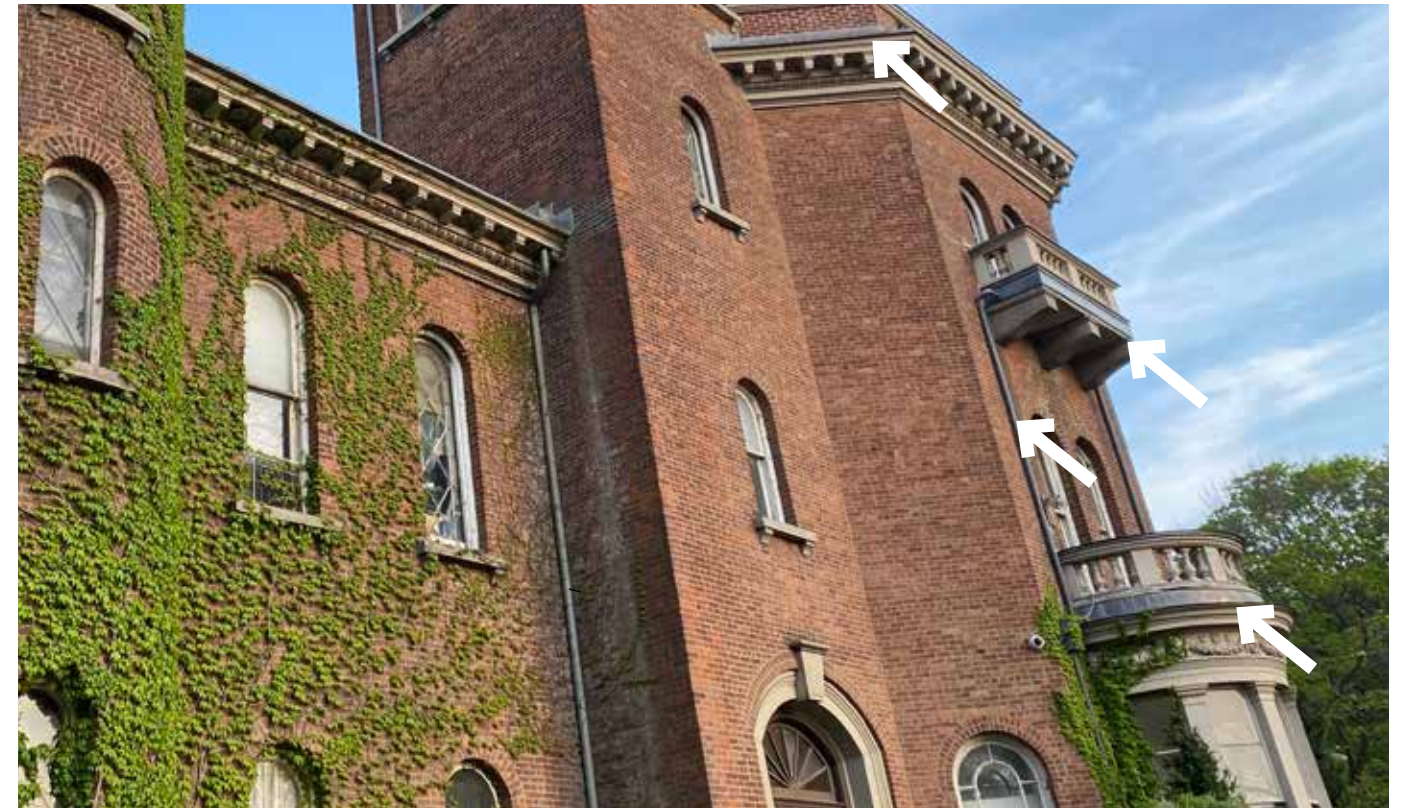
Only lead coated copper elements on front of building.
