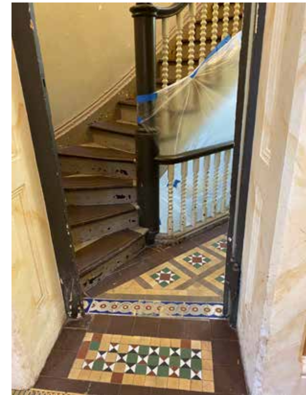
STAIRS AT FROM LOBBY
