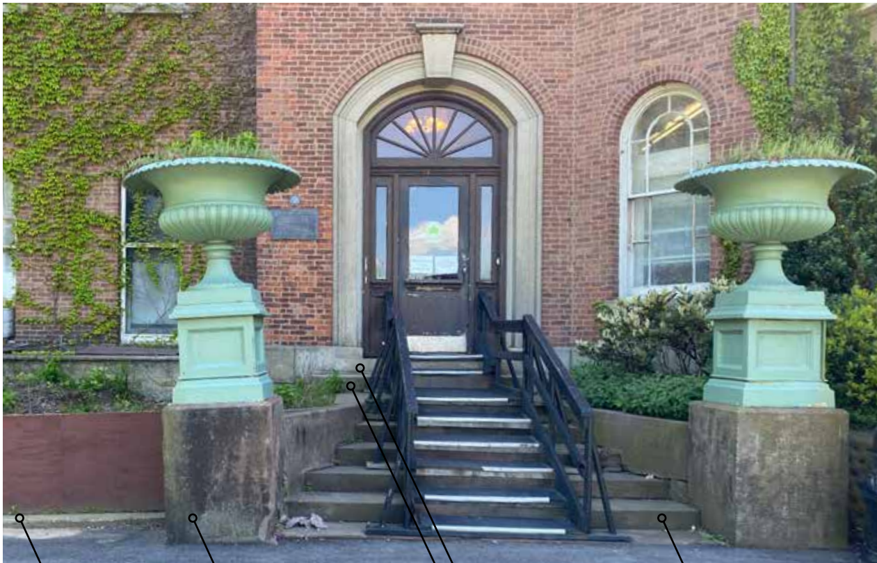
3 First brownstone step is buried, landing is also brownstone
