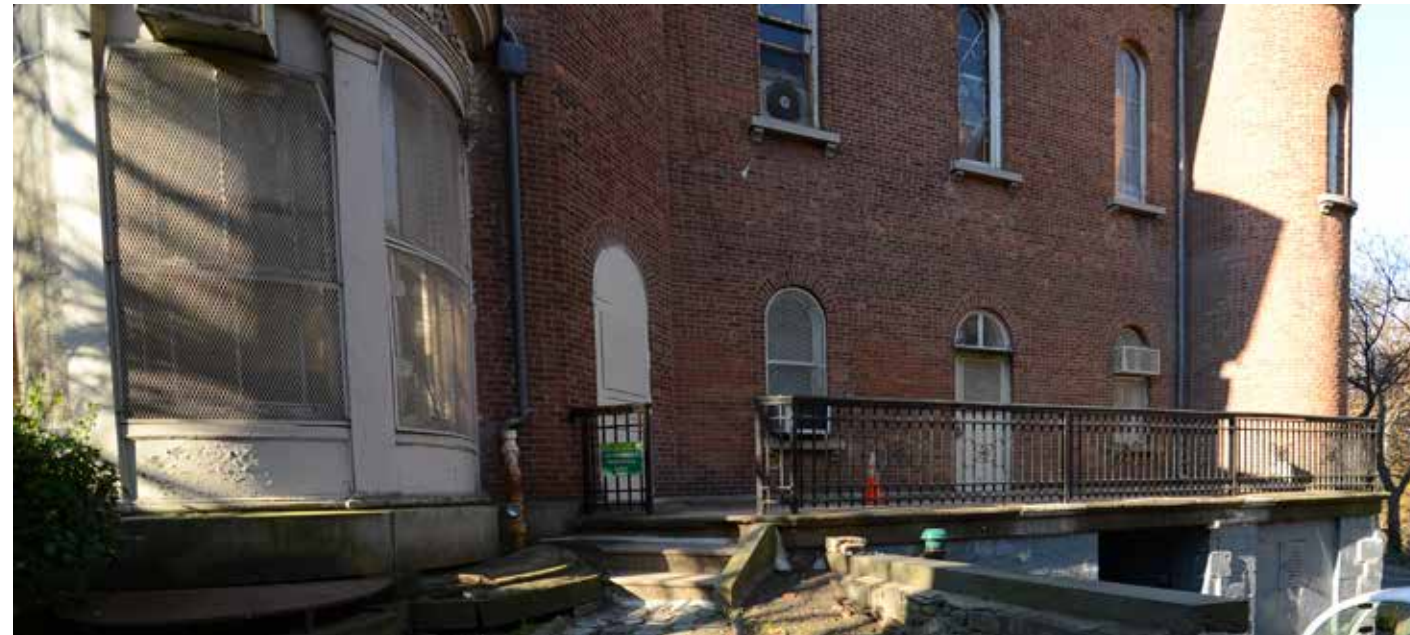
Cream metal mesh on windows. Painted black steel fence on terrace.
