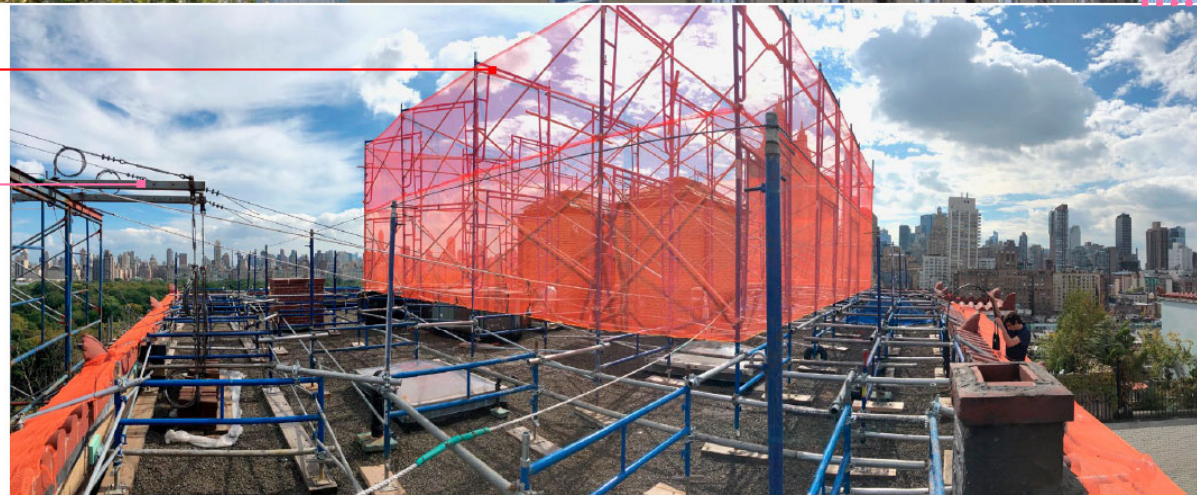
Facade Maintenance Rigging
