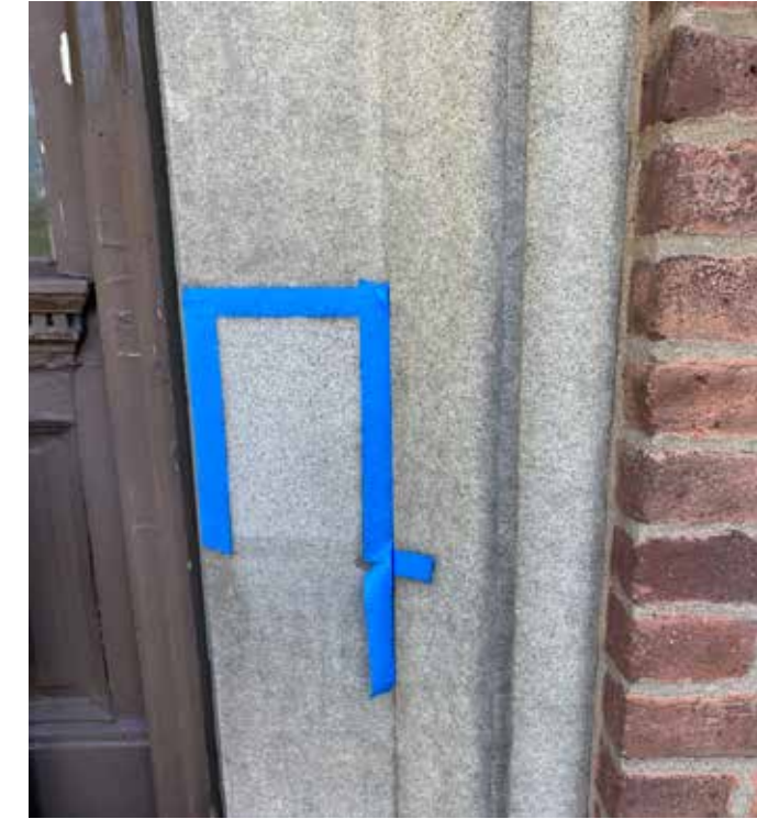
Cleaning test at granite door surround using detergent cleaner.
