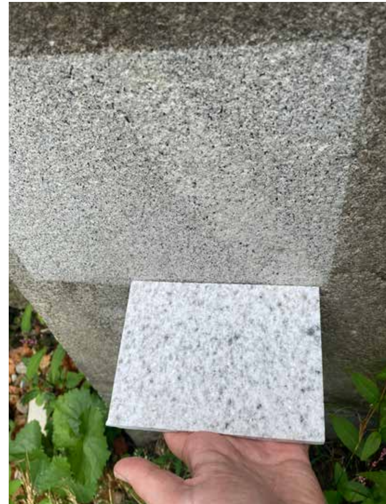
Bethel White granite for ramp surface and landing, as pictured in front of cleaned door surround
