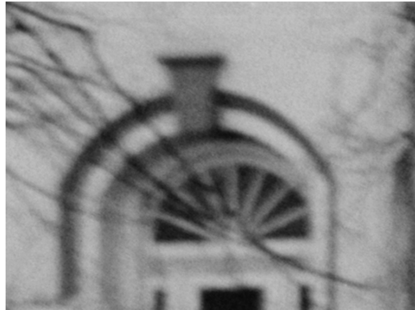
Historic 1934 photo of entrance shows paint at door surround matching the color found at the earliest extant finish layer.
