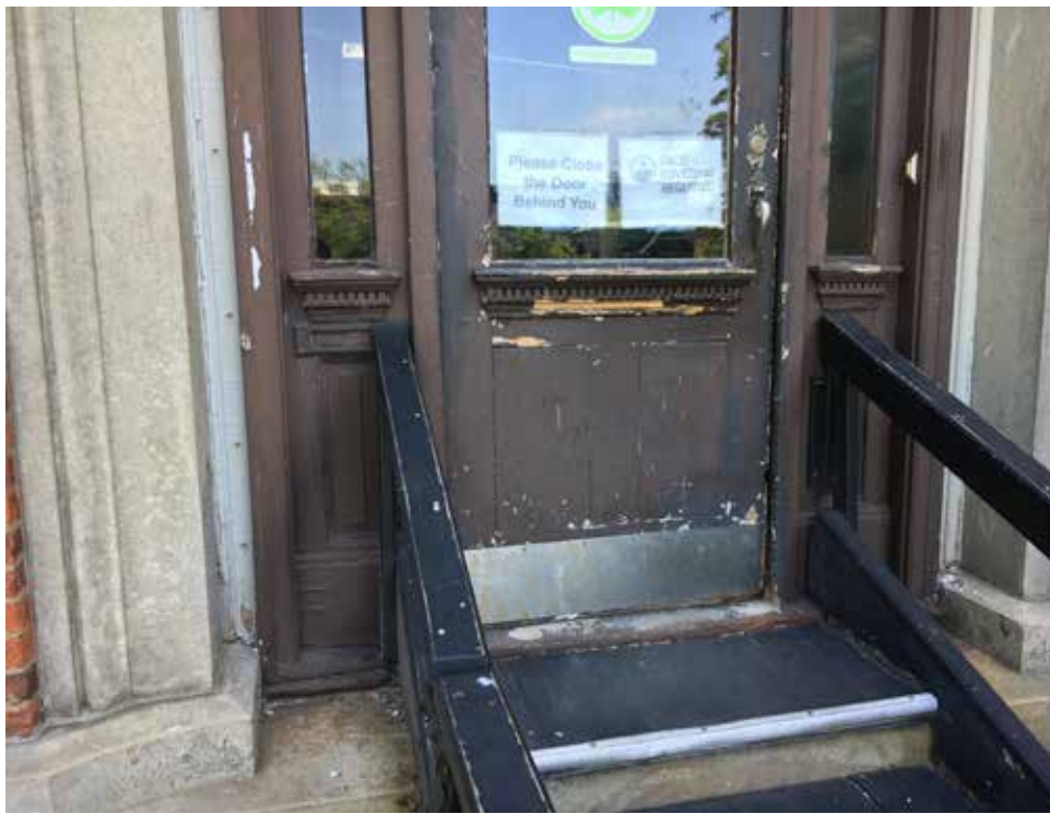
Granite door surround and base exhibiting general soiling.
