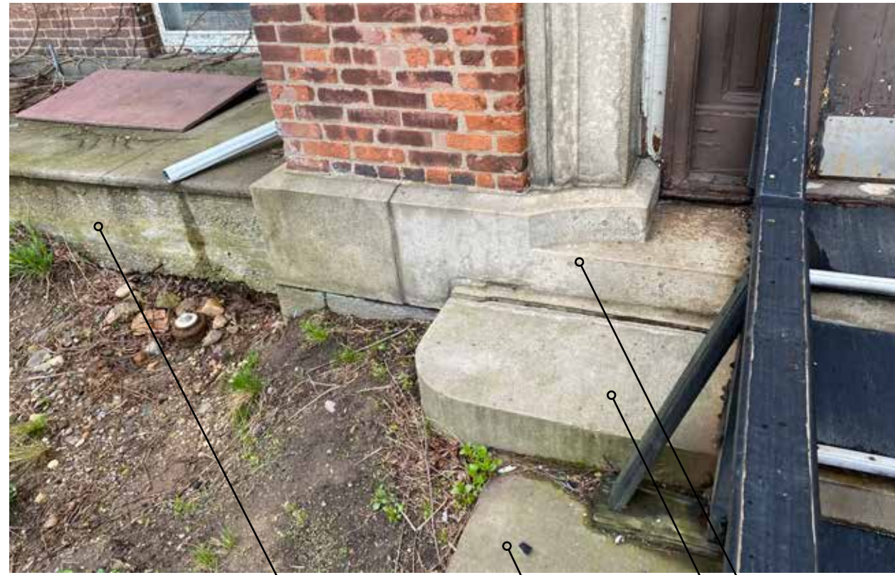
4 Top two steps are granite and match the building granite
