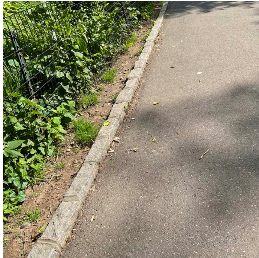
Granite Block Edging & Asphalt
