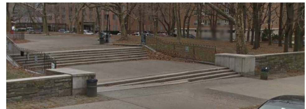
Existing Stair Entrance on Myrtle Avenue
