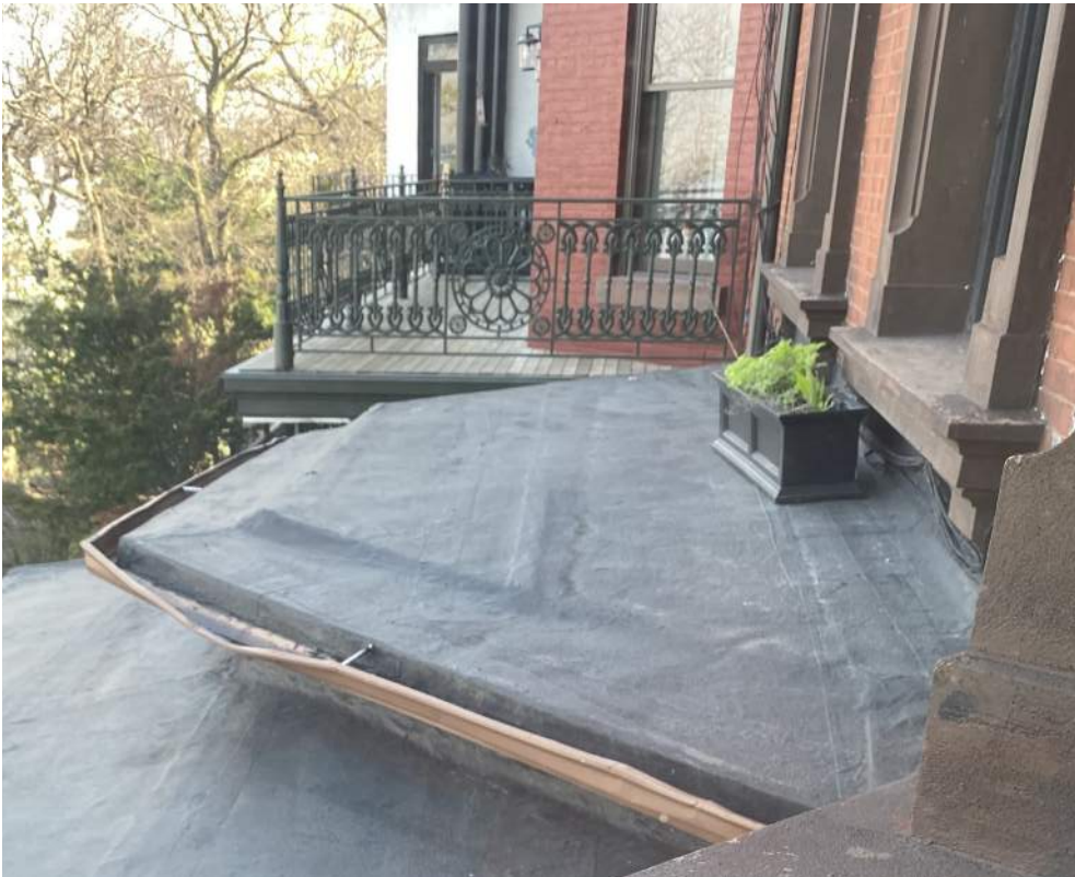
7 DETAIL VIEW OF 2ND FLOOR BAY WINDOW ROOF(AT 3RD FLOOR)
