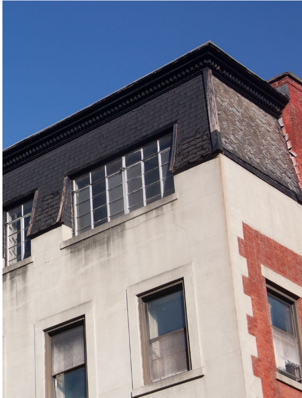
B. EXISTING MANSARD ROOF
