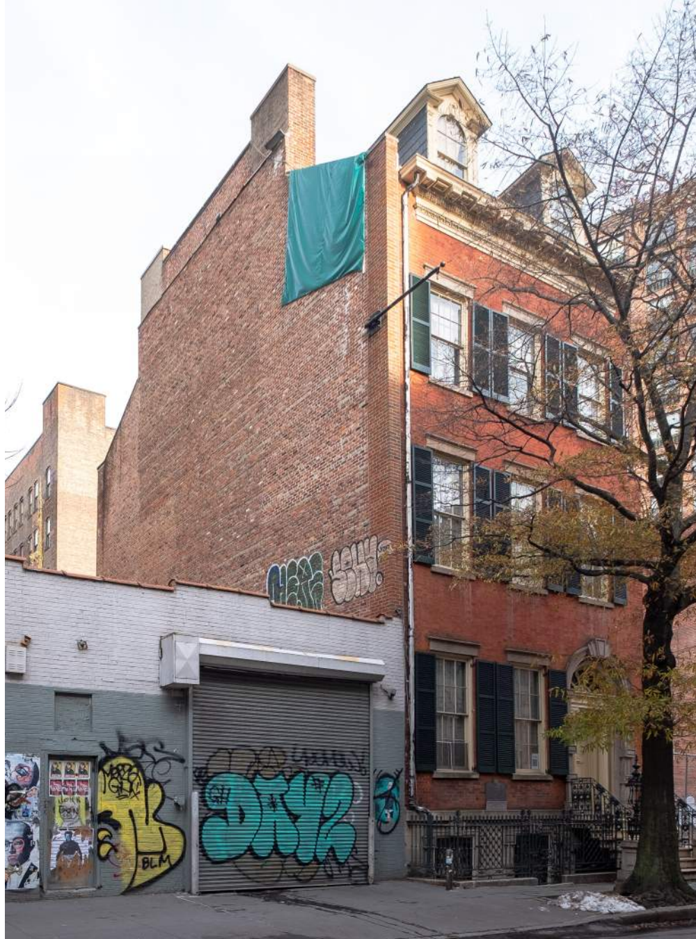
CURRENT LOT LINE WALL CONDITION
