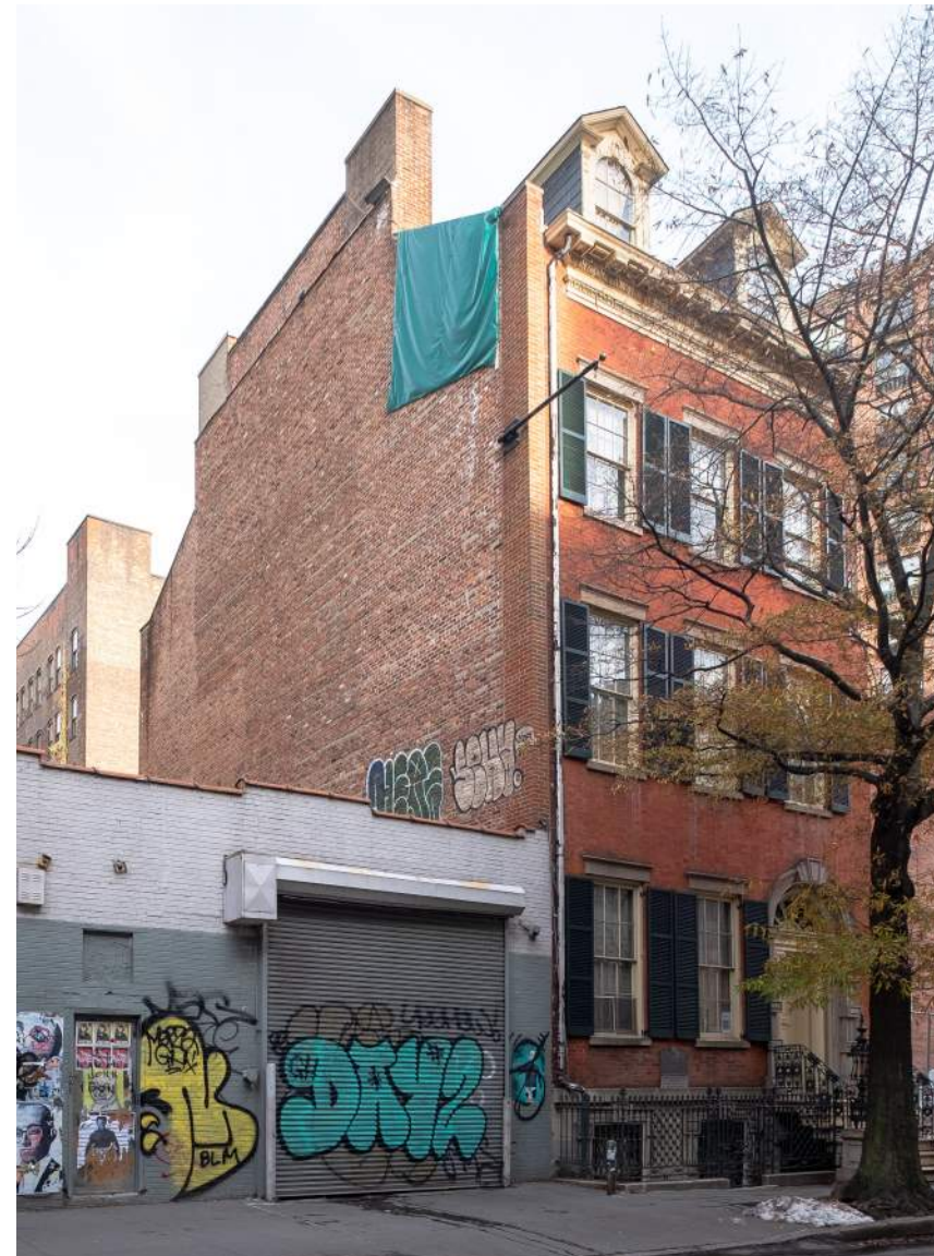
CURRENT LOT LINE WALL CONDITION
