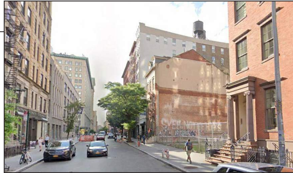
A - EAST STREET VIEW - FROM E 4TH ST & BOWERY
