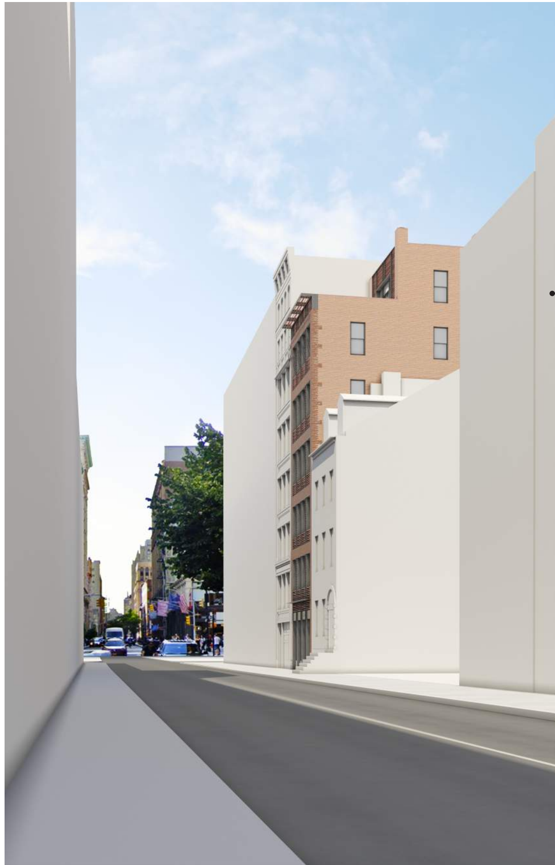
EAST STREET VIEW - FROM E 4TH ST & BOWERY
