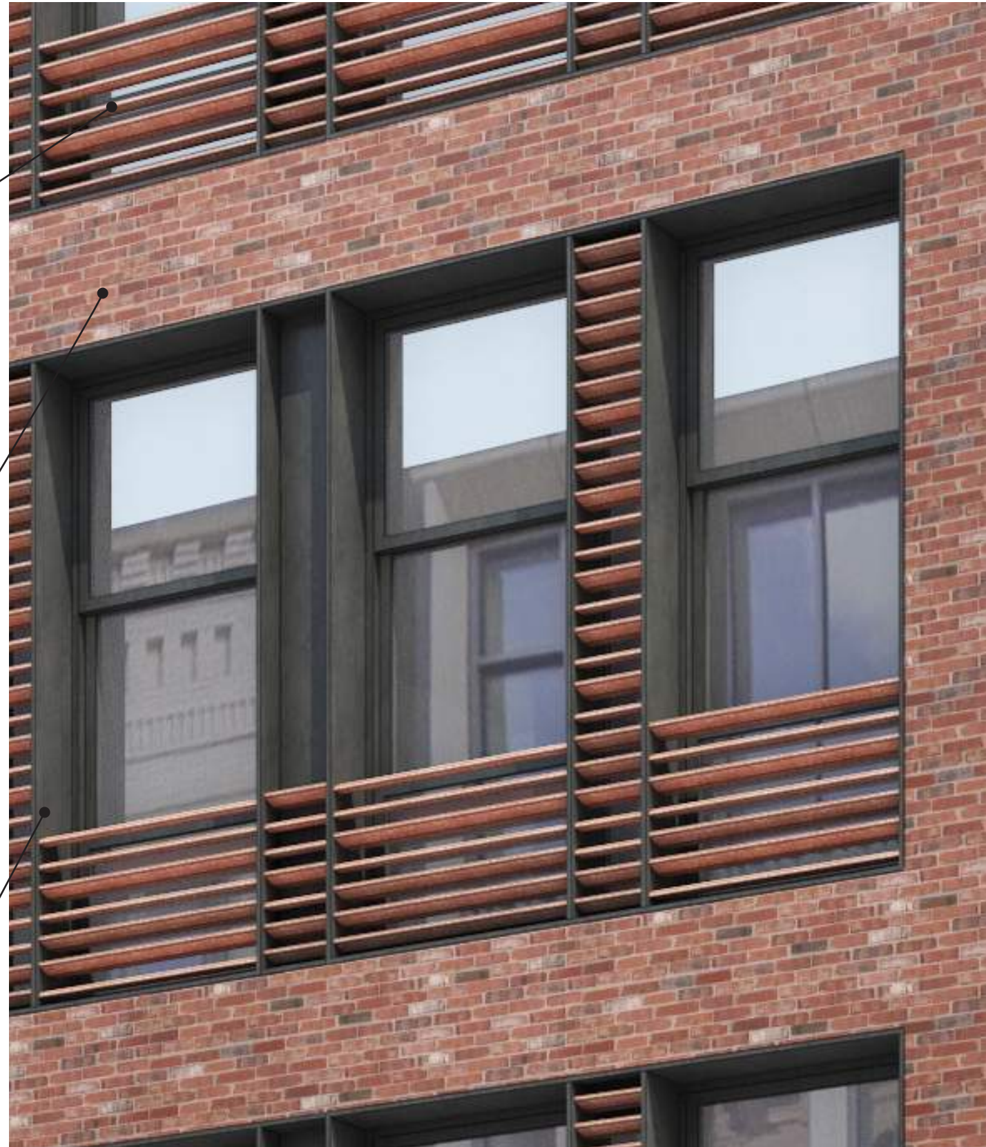
CLOSE UP OF TERRA COTTA SCREENS IN METAL FRAMES OVER CONTINUOUS WINDOWS
