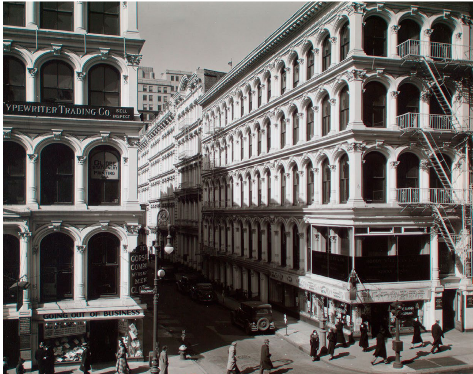
BROADWAY @ THOMAS ST. LOOKING WEST
