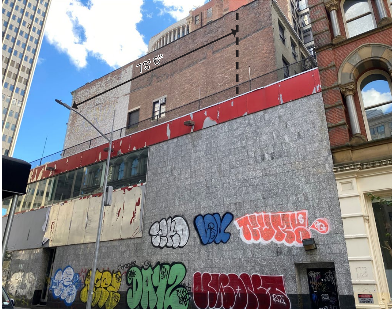
JUNE 2020, REAR OF 315 BROADWAY FROM THOMAS STREET
