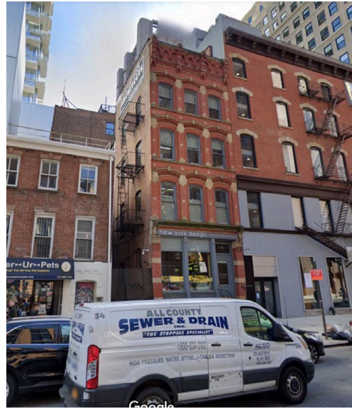
175 WEST BROADWAY DATE: 1877; ARCHITECT: SCOTT & UMBACH
