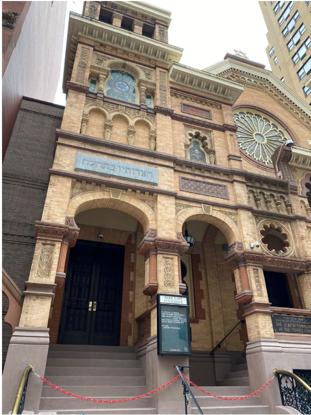
1 ST FLOOR ENTRANCE
