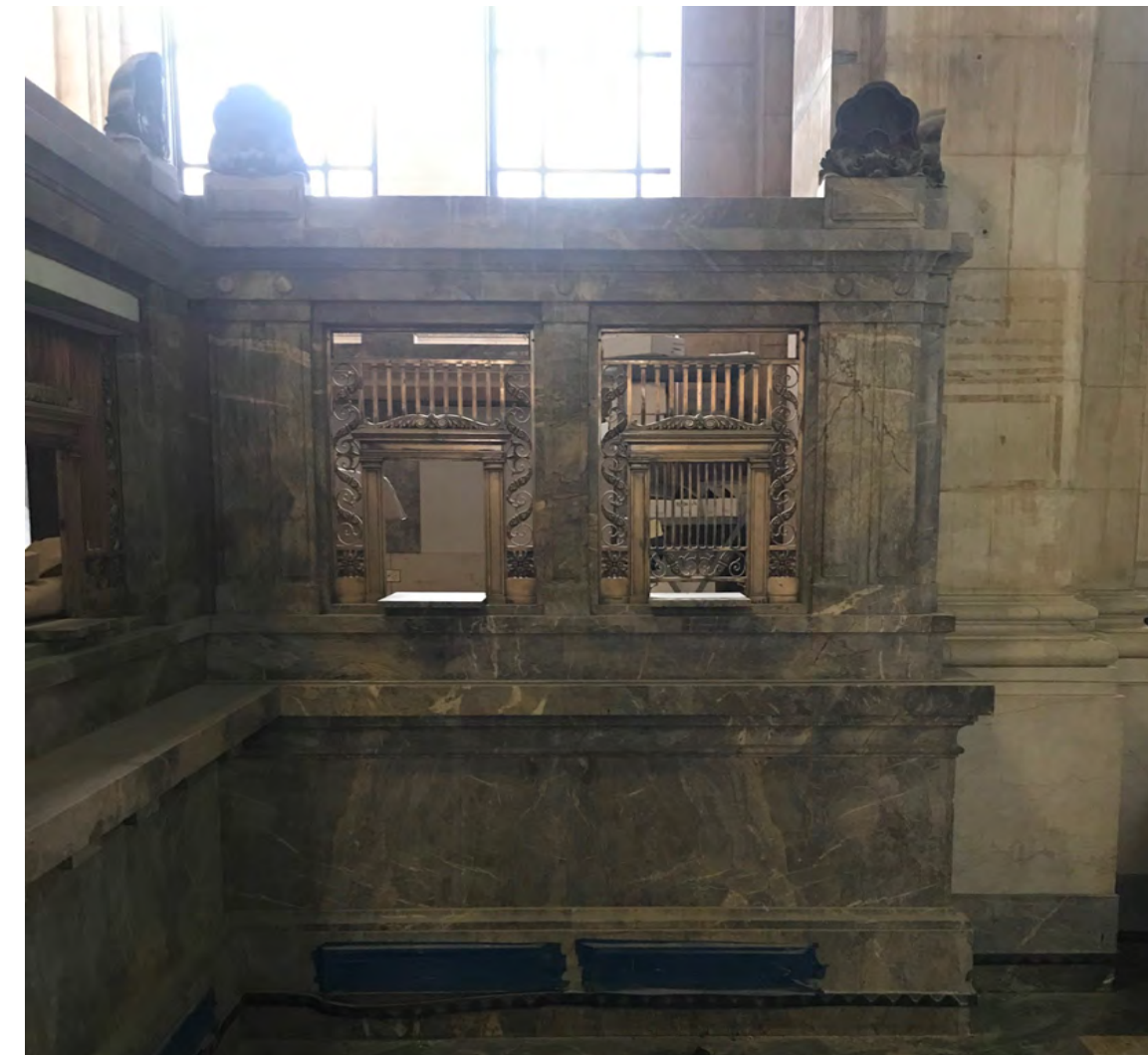
2 EXISTING PHOTO @ NORTH TELLERS
