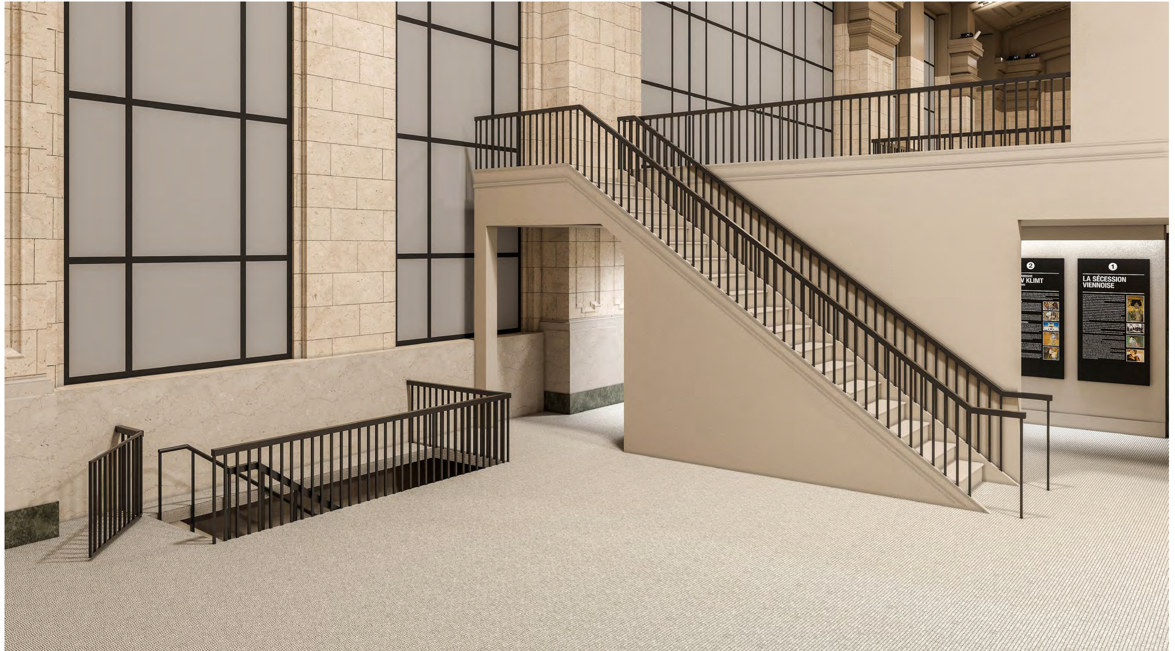
EXISTING VIEW OF STAIRS
