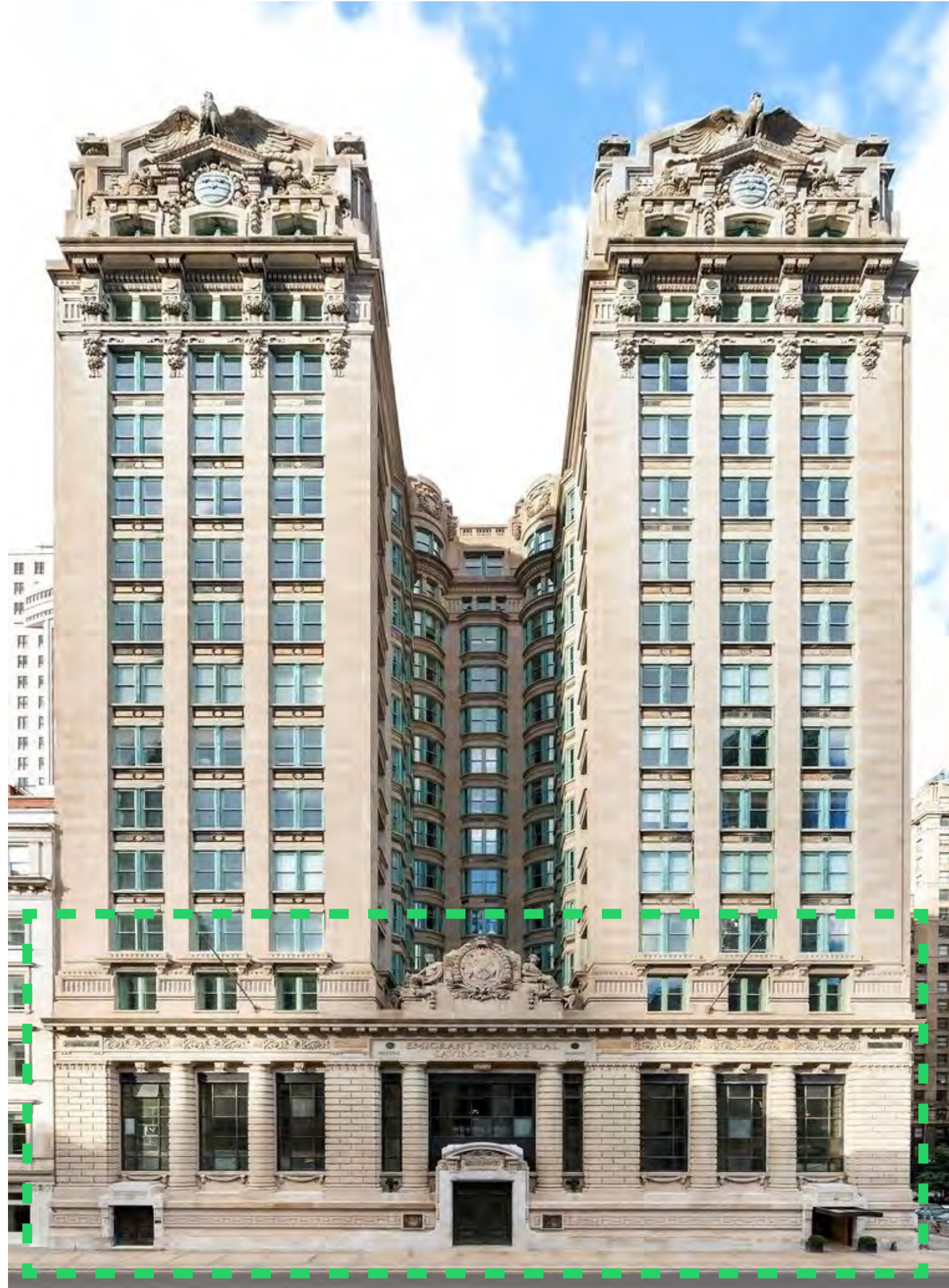
EXISTING CHAMBERS STREET FACADE
