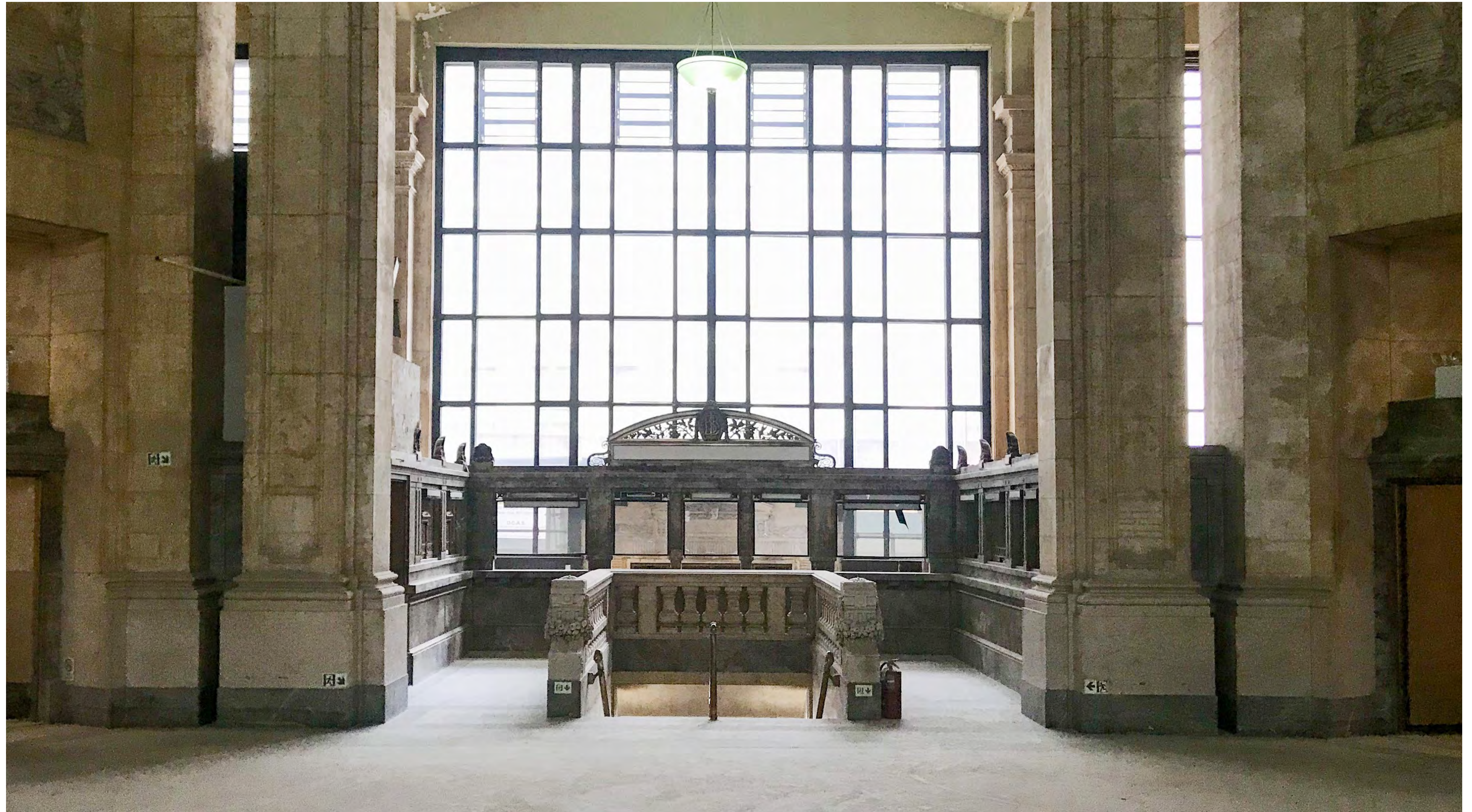
CURRENT INTERIOR CONDITIONS
