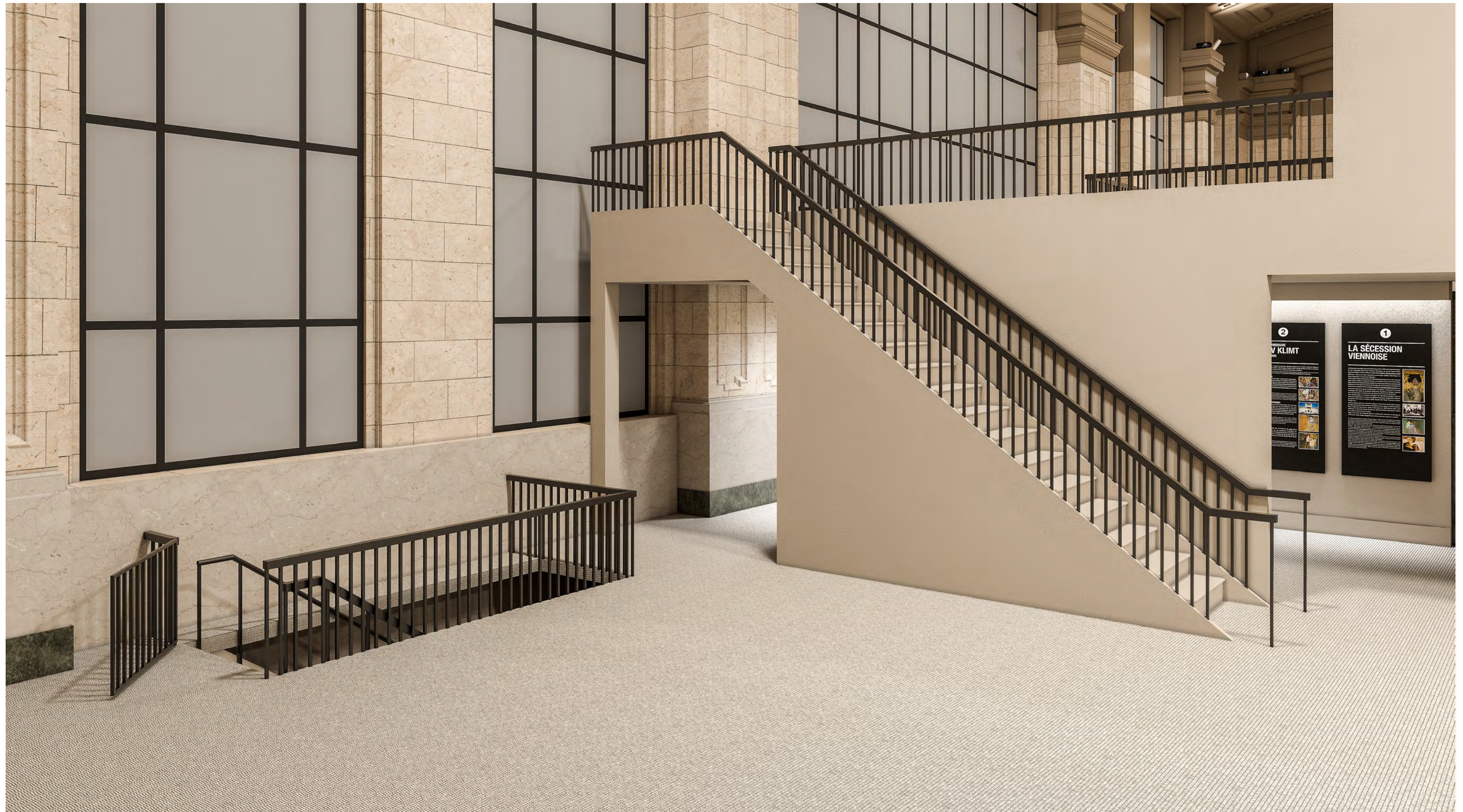
EXISTING VIEW OF STAIRS
