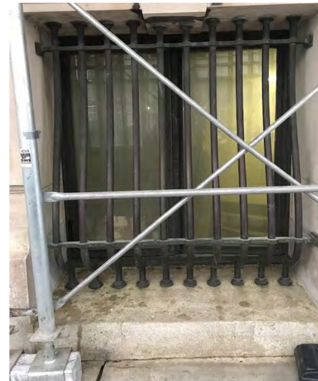
2 TYPICAL EXISTING WINDOW
