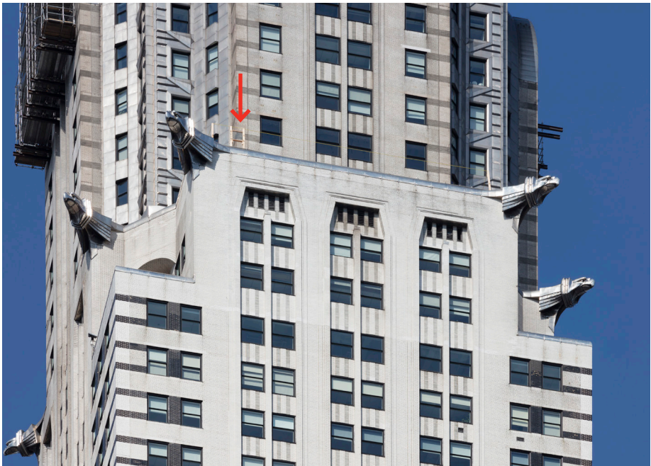
ZOOMED IN VIEW OF TERRACE RED ARROW POINTS TO GLASS SAMPLE MOCK-UP. CABLE AND WOODEN POSTS REPRESENT EXTENT OF GLASS SCREEN.
