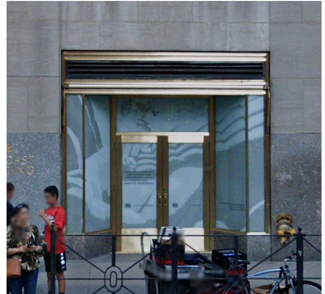
3 EXISTING CONDITIONS 1250 AVENUE OF THE AMERICAS - WEST ELEVATION
