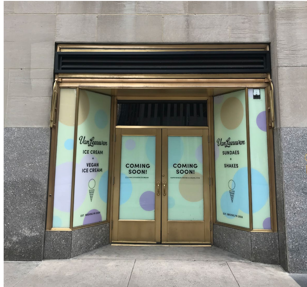
2 EXISTING CONDITIONS 1250 AVENUE OF THE AMERICAS - WEST ELEVATION
