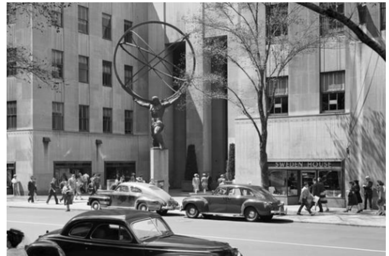
3. 45 Rockefeller Plaza (630 Fifth Avenue), view of Fifth Avenue storefronts, 1950. (MCNY)
