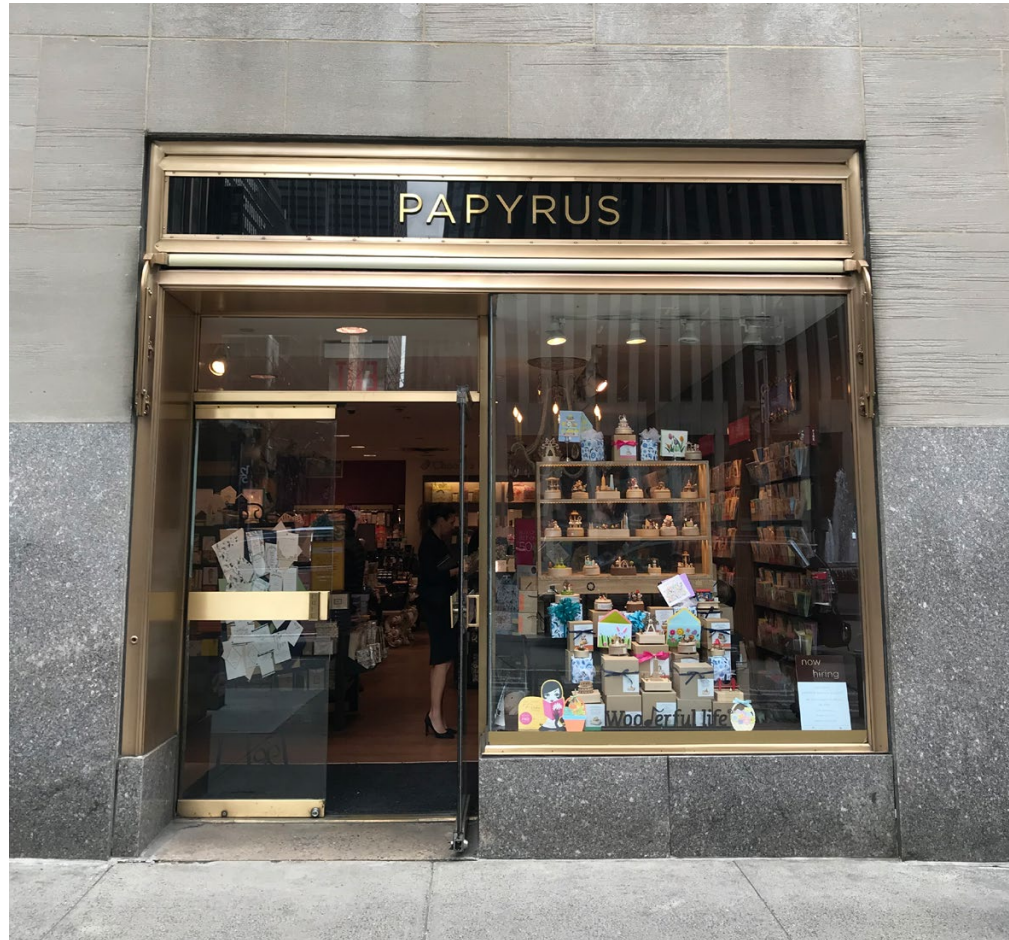
1 EXISTING CONDITIONS 1250 AVENUE OF THE AMERICAS - WEST ELEVATION
