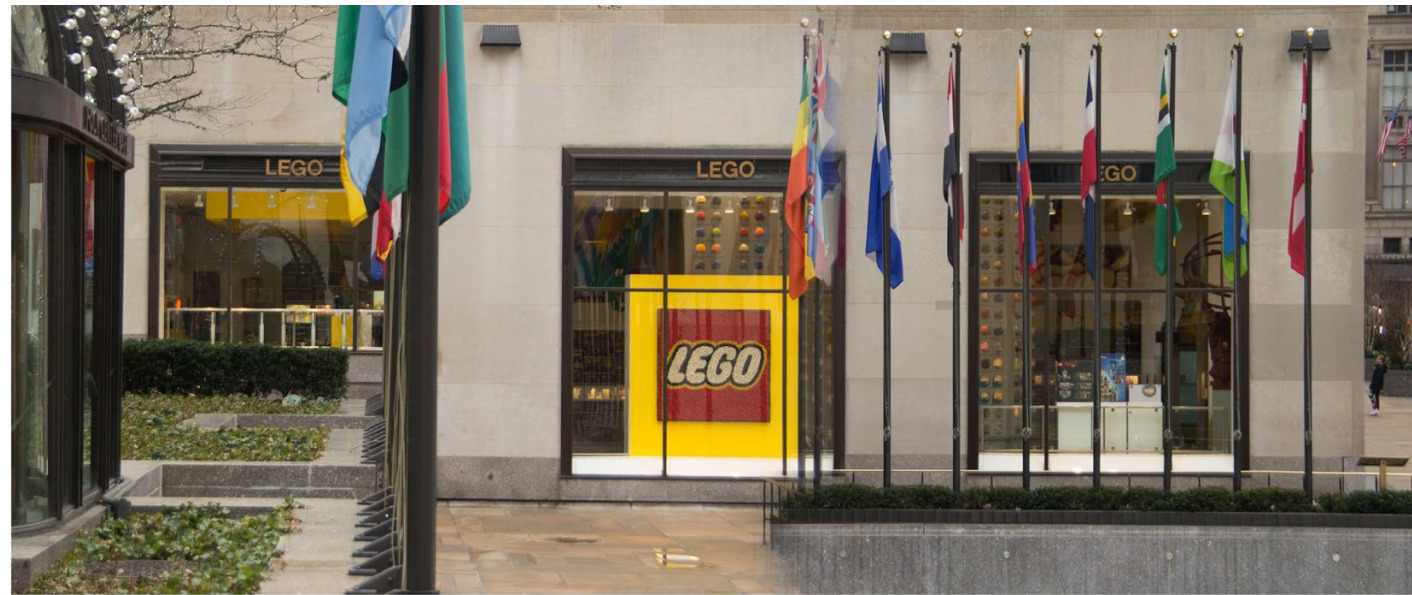
620 FIFTH AVE - WEST FACADE
