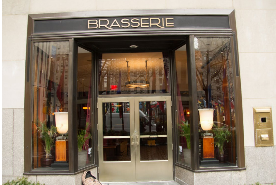
12 EXISTING CONDITIONS 45 ROCKEFELLER PLAZA - W50TH STREET ELEVATION
