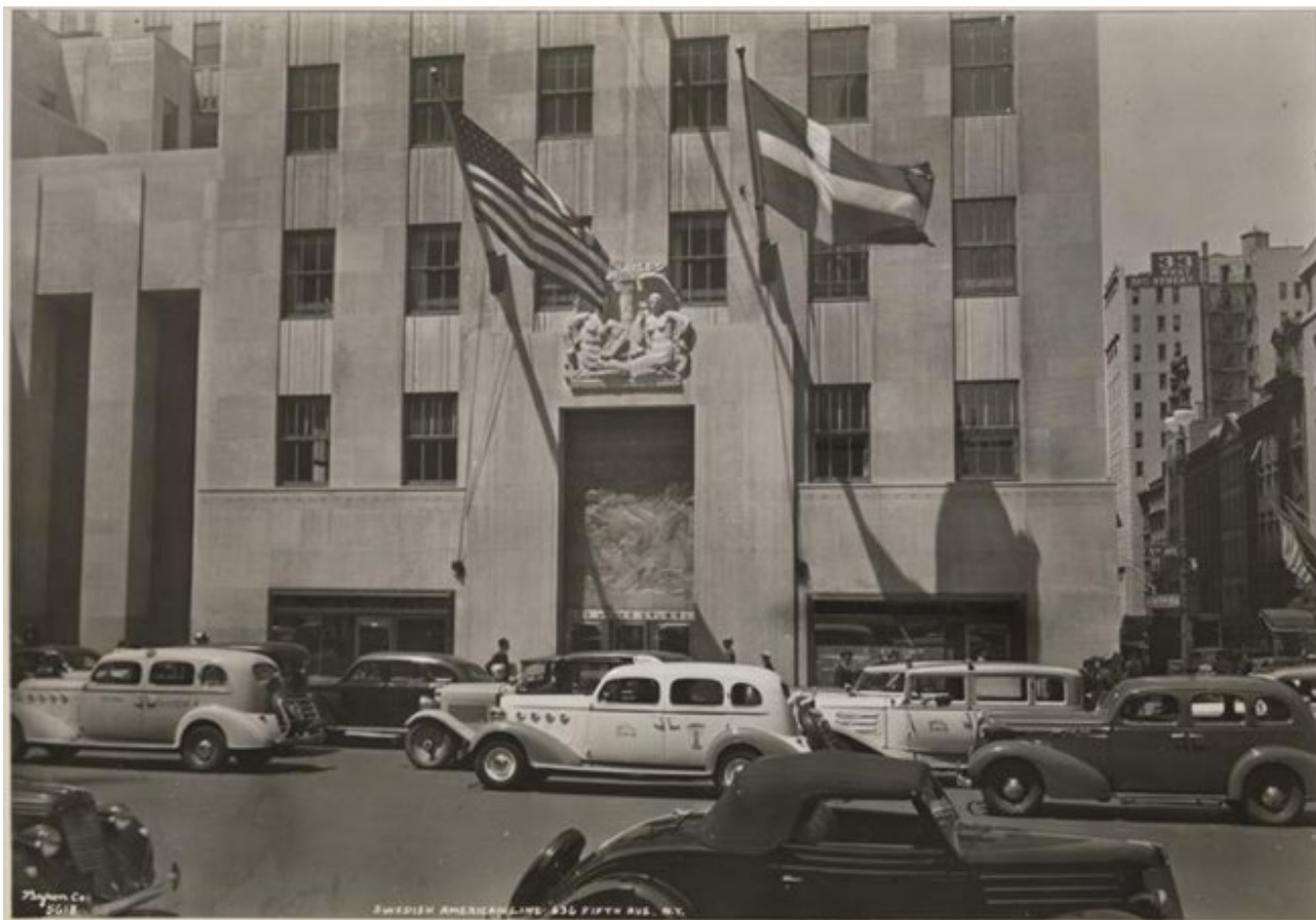
2. 45 Rockefeller Plaza (630 Fifth Avenue), view of Fifth Avenue storefronts, 1936. (MCNY)
