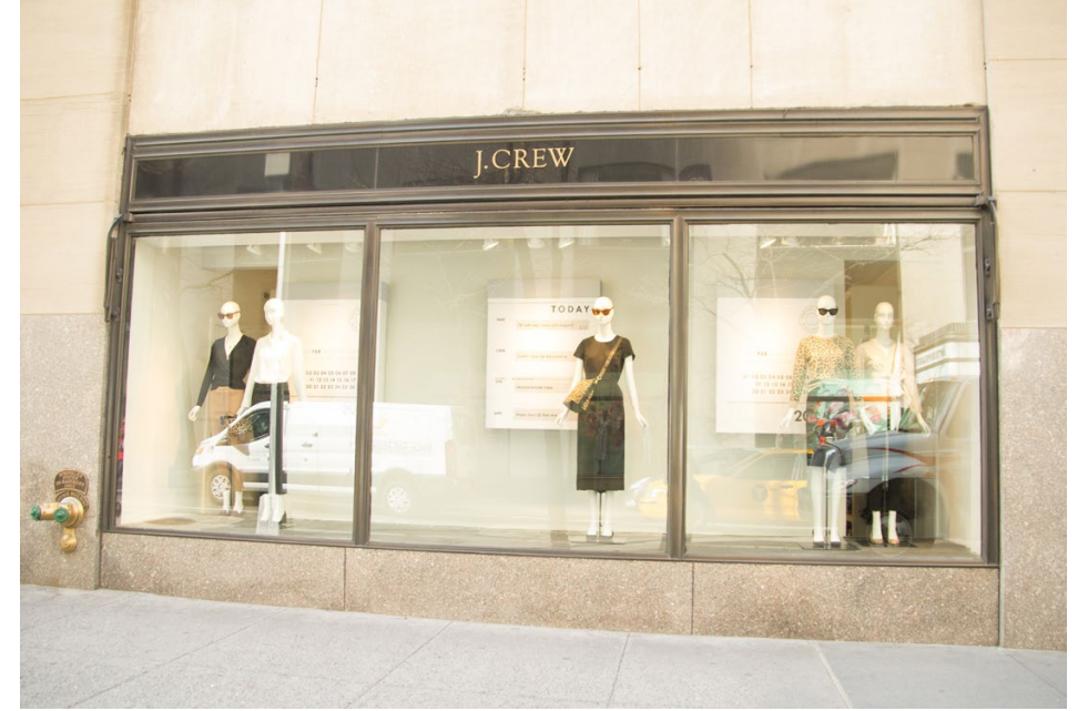
18 EXISTING CONDITIONS 30 ROCKEFELLER PLAZA - W50TH STREET ELEVATION
