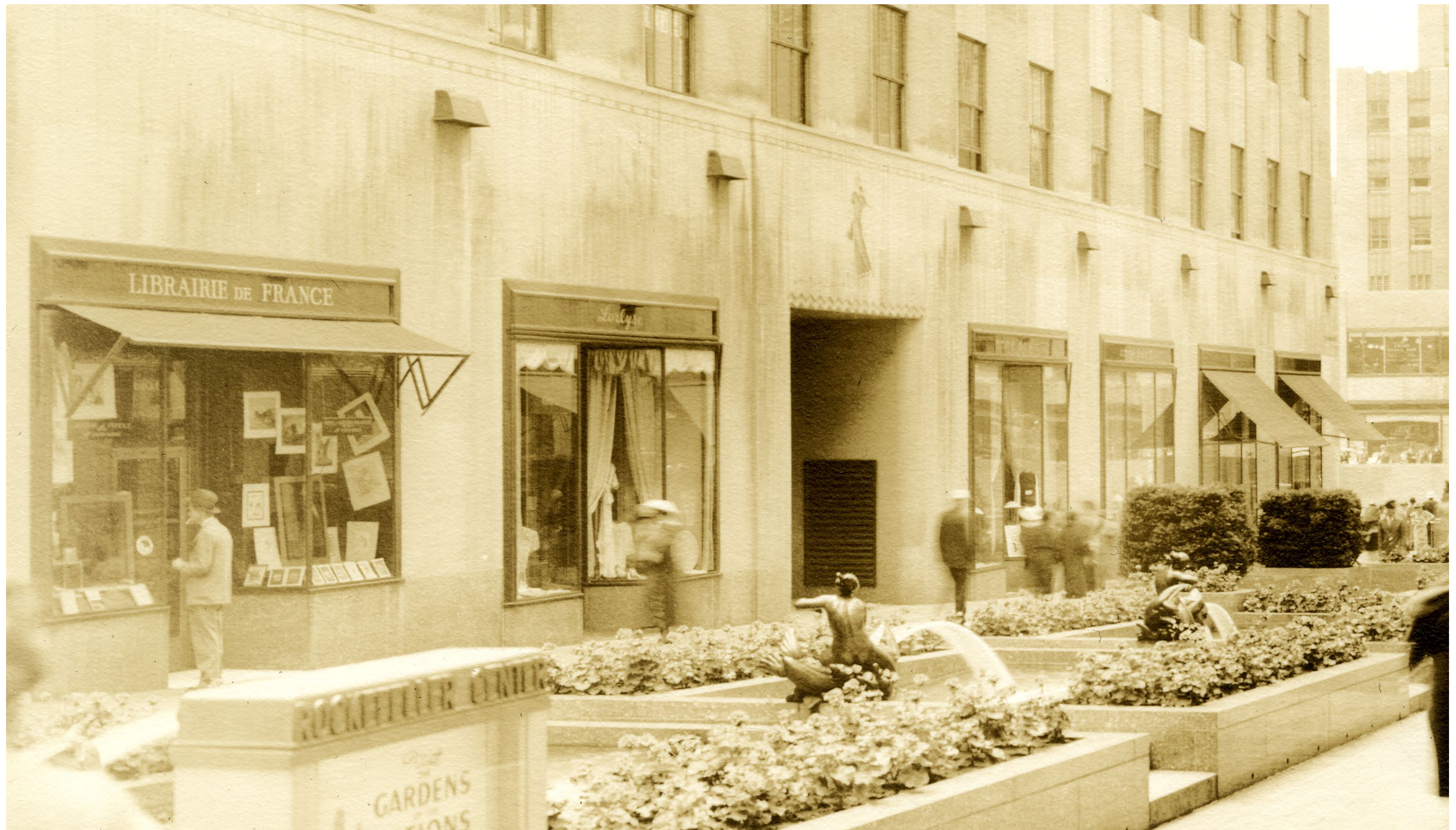
610 Fifth Avenue, view of north facade storefronts, 1935. (NYHS)
