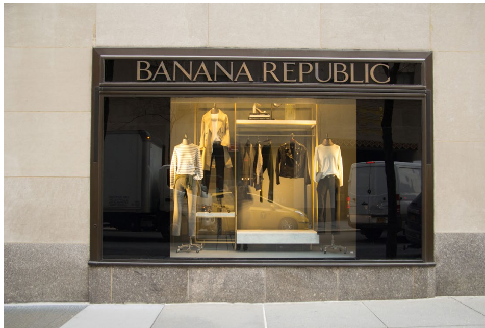
5 EXISTING CONDITIONS 45 ROCKEFELLER PLAZA - W50TH STREET ELEVATION
