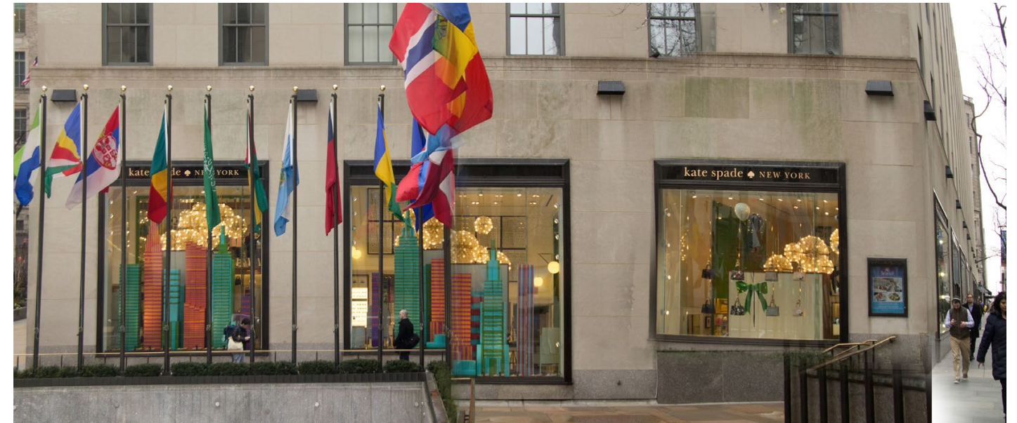
610 FIFTH AVE - WEST FACADE
