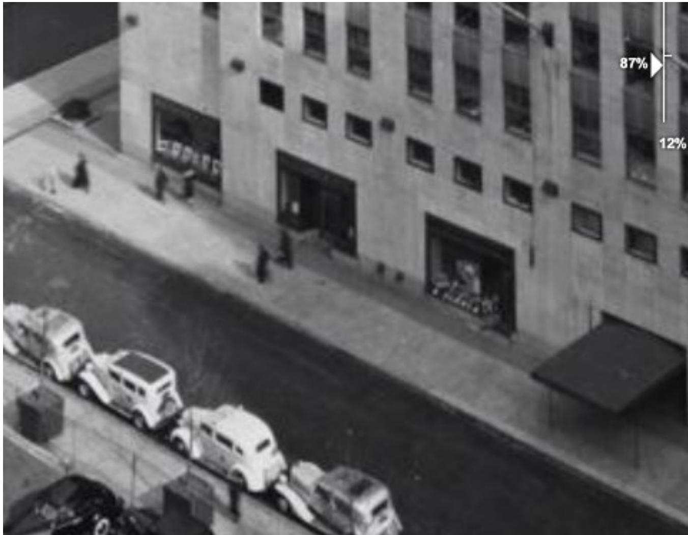
1. View of northern storefronts, ca. 1950. (MCNY)
