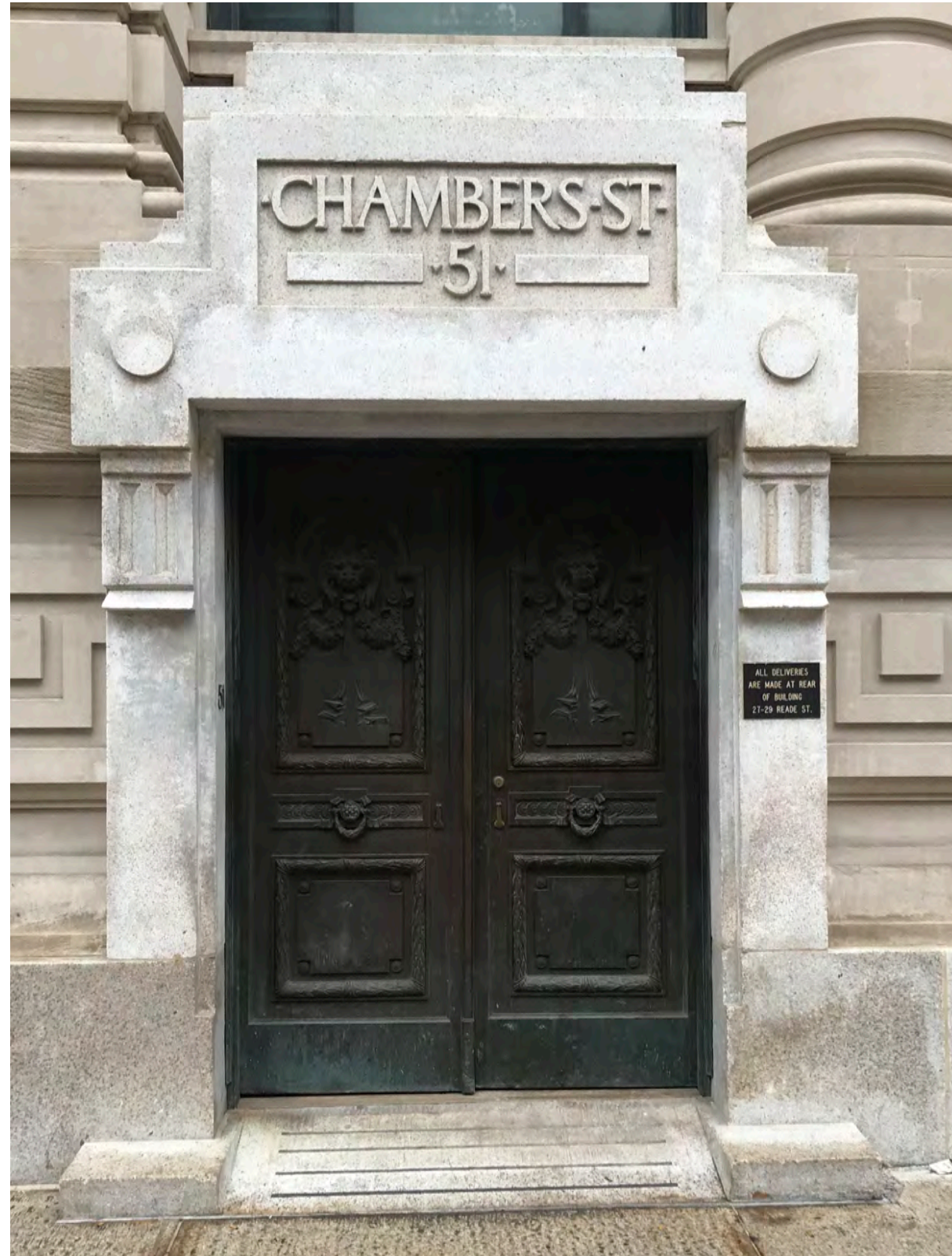
1 EXISTING 51 CHAMBERS ST. ENTRANCE
