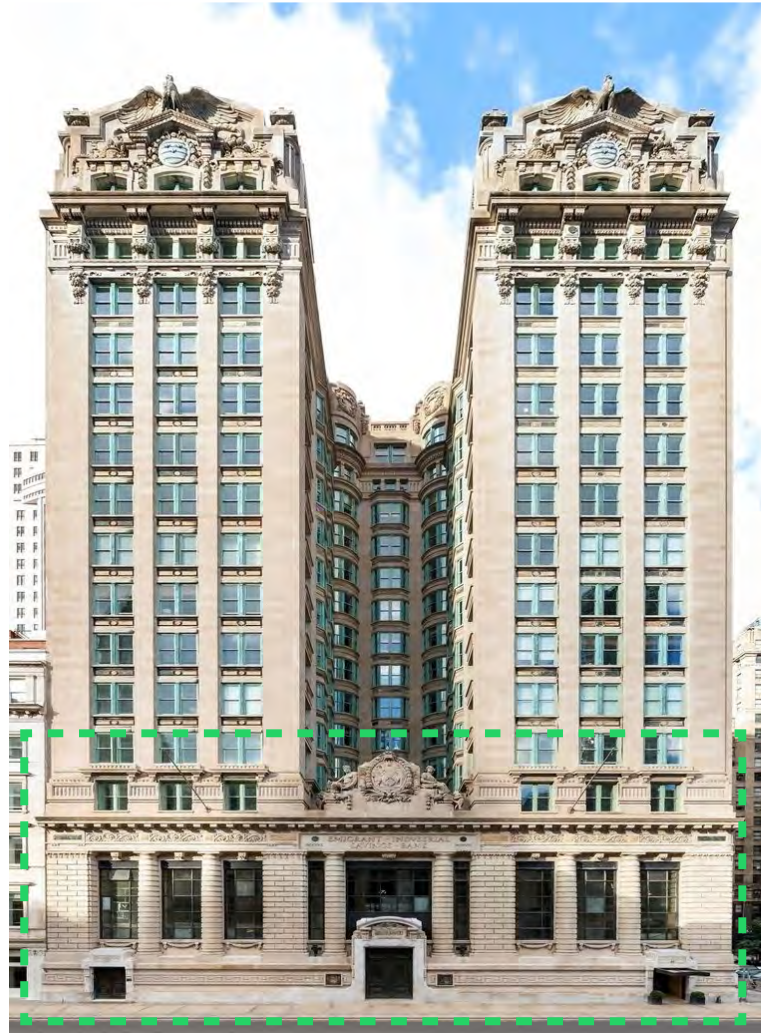
EXISTING CHAMBERS STREET FACADE
