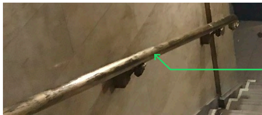
FIXTURE AT EXISTING HANDRAIL
