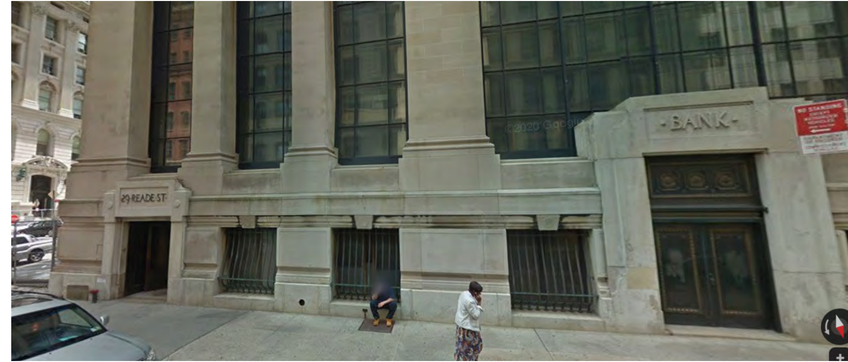
1 EXISTING READE STREET FACADE
