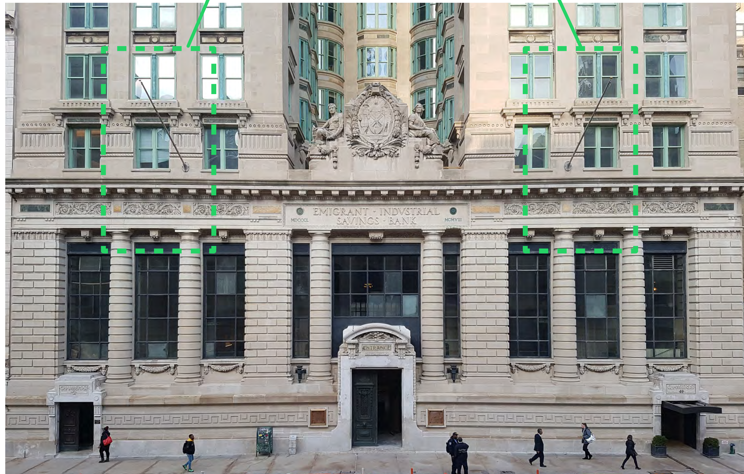
EXISTING CHAMBERS STREET FACADE
