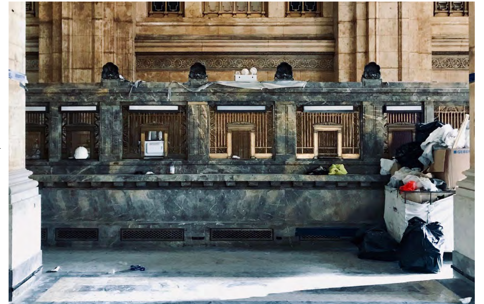
2 EXISTING PHOTO @ WEST TELLERS
