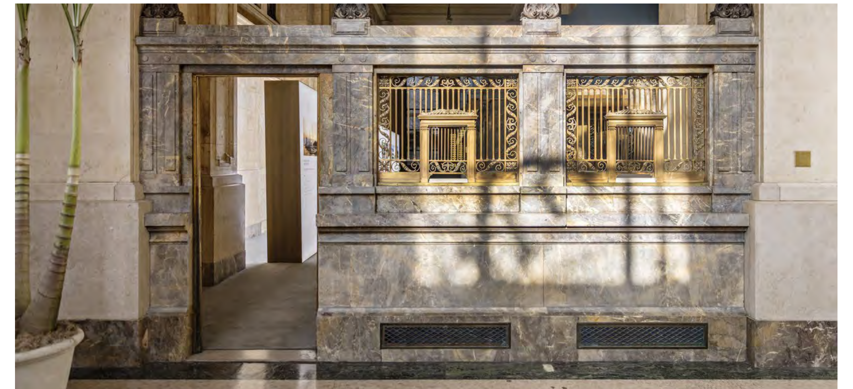
2 EXISTING PHOTO @ FRONT TELLERS
