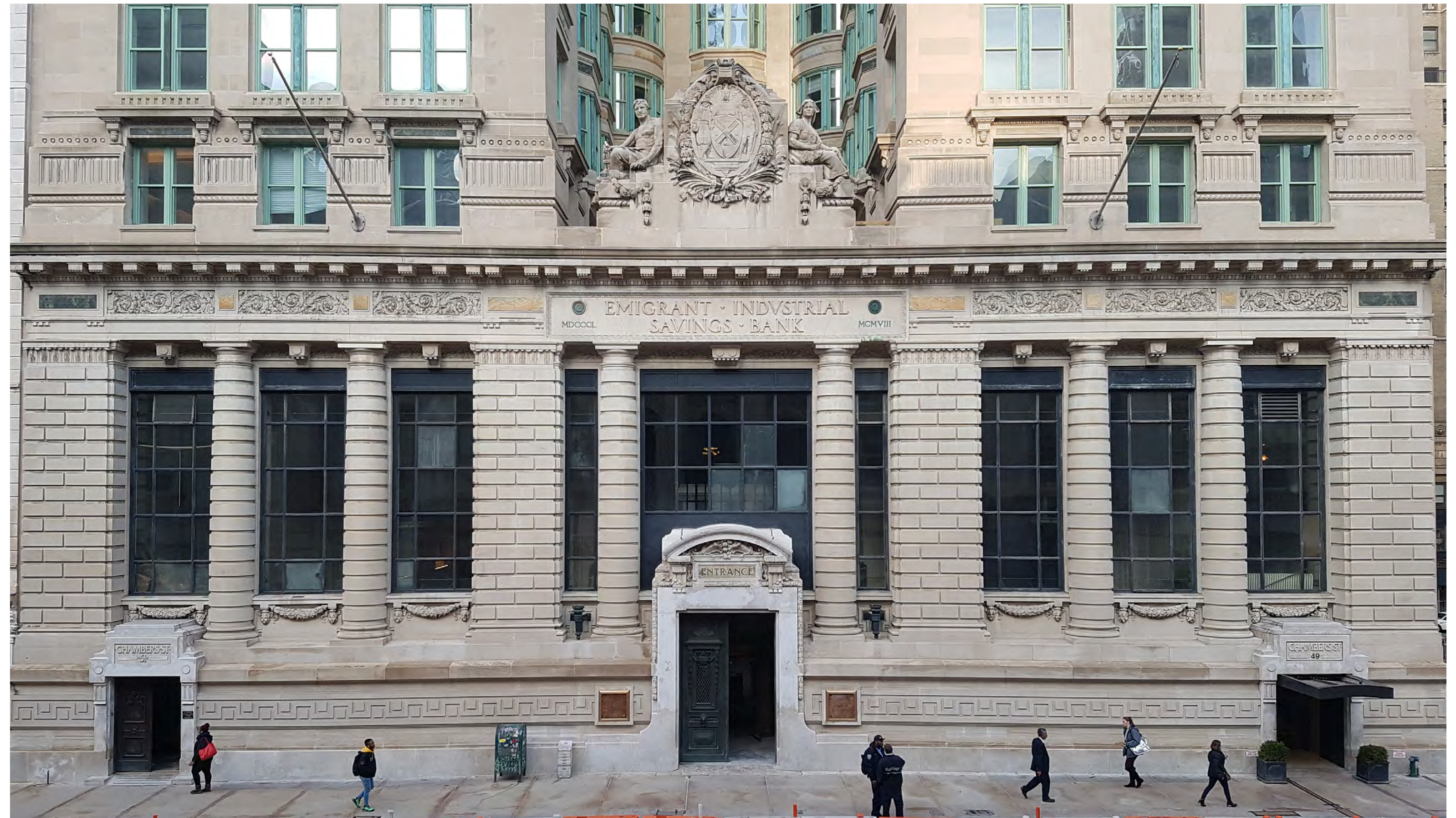
EXISTING CHAMBERS STREET FACADE
