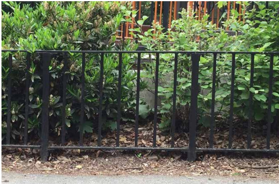
2'-6" Ht Steel Fence to replace Chain Link Fence
