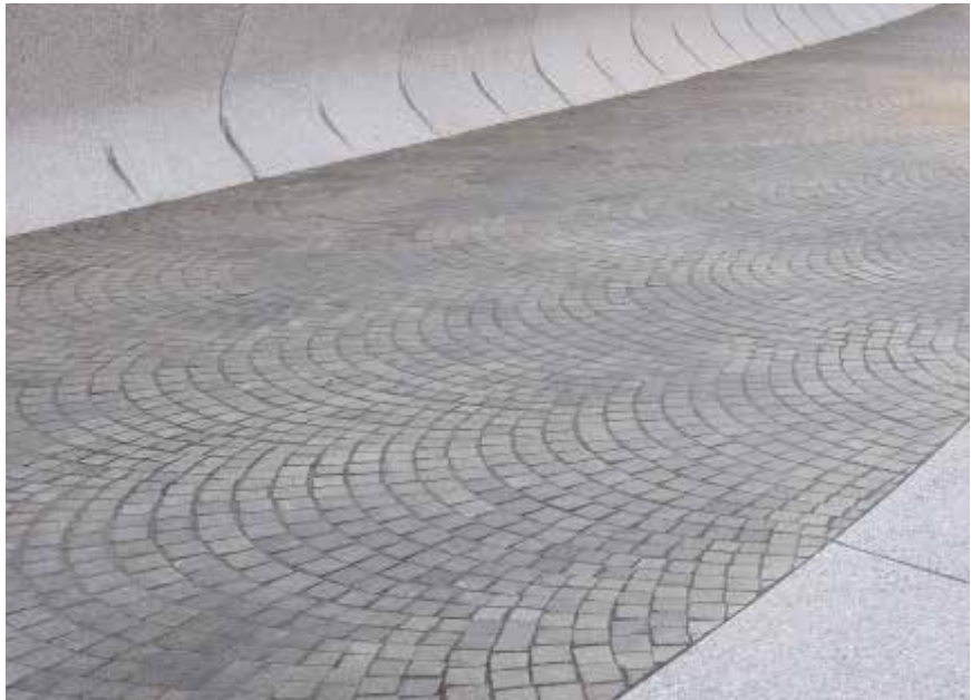
Granite Sett, fan pattern, sawn and sanded finish, on concrete
