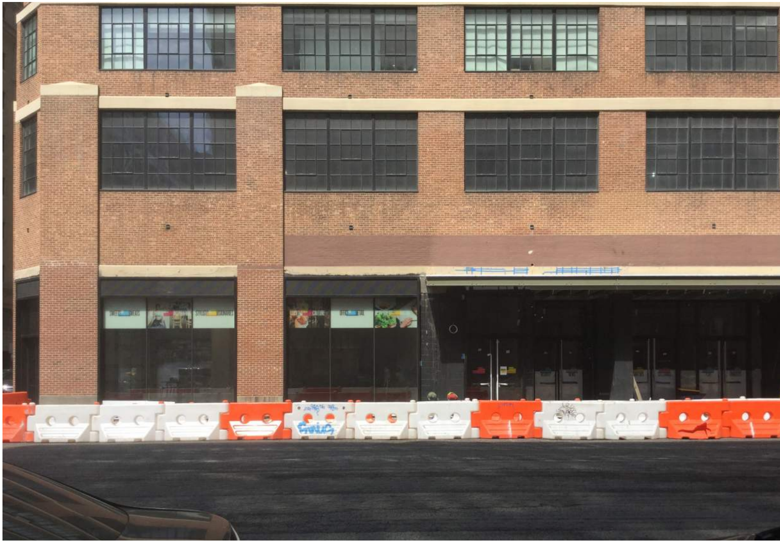
11th Avenue facade, frontal view of proposed work location
