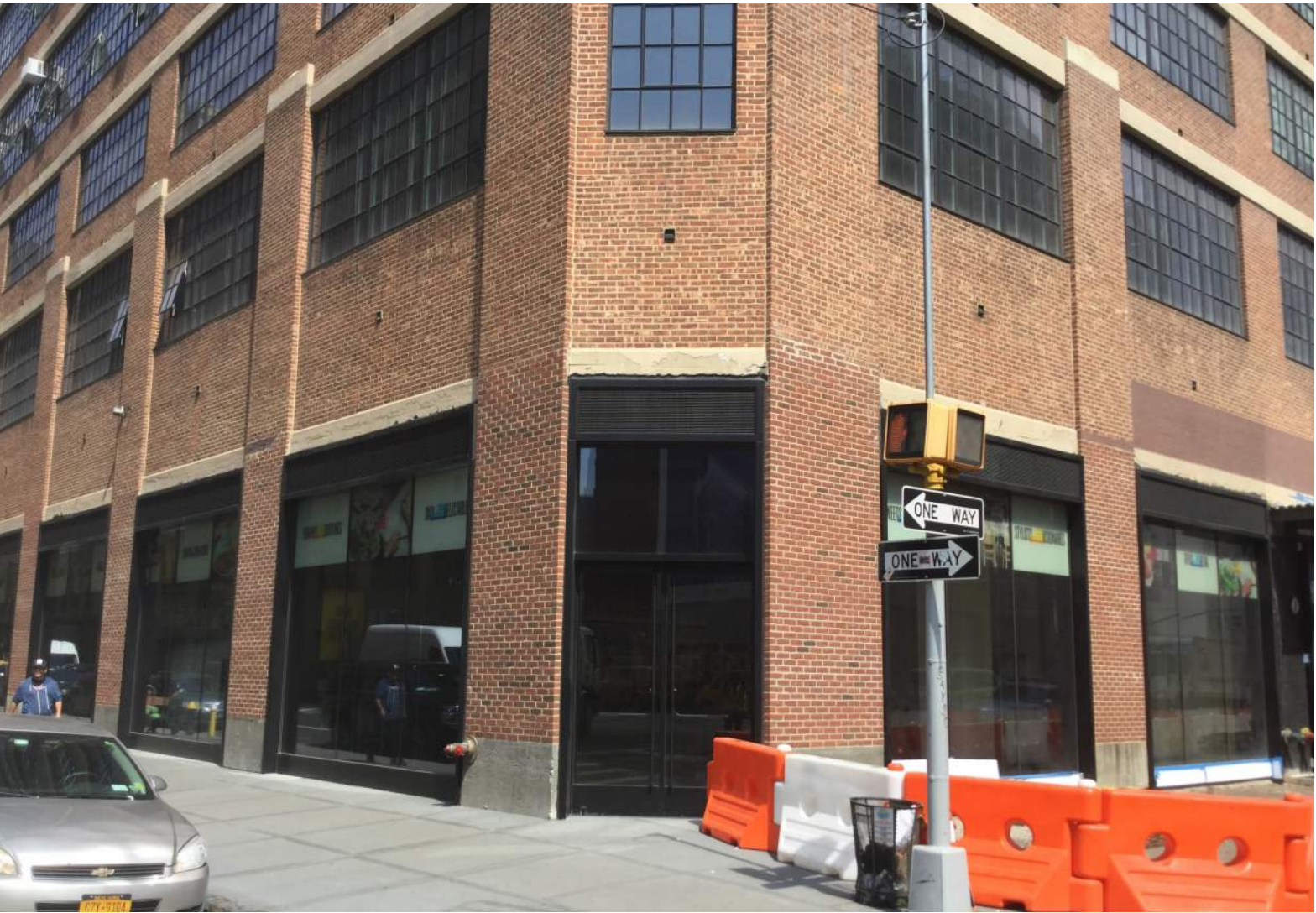
11th Avenue and 26th Street corner
