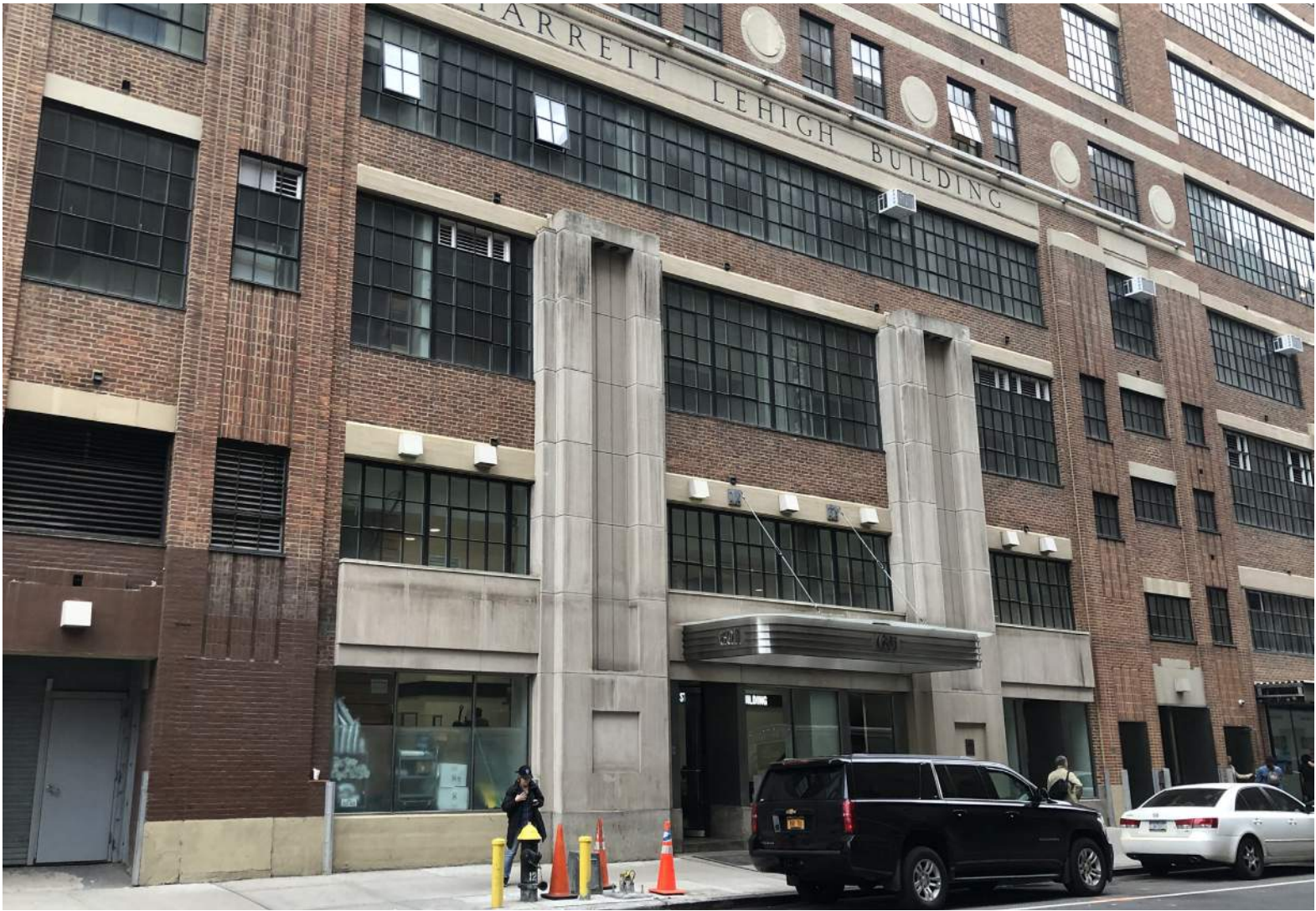
26th Street facade, view looking east at main building entrance
