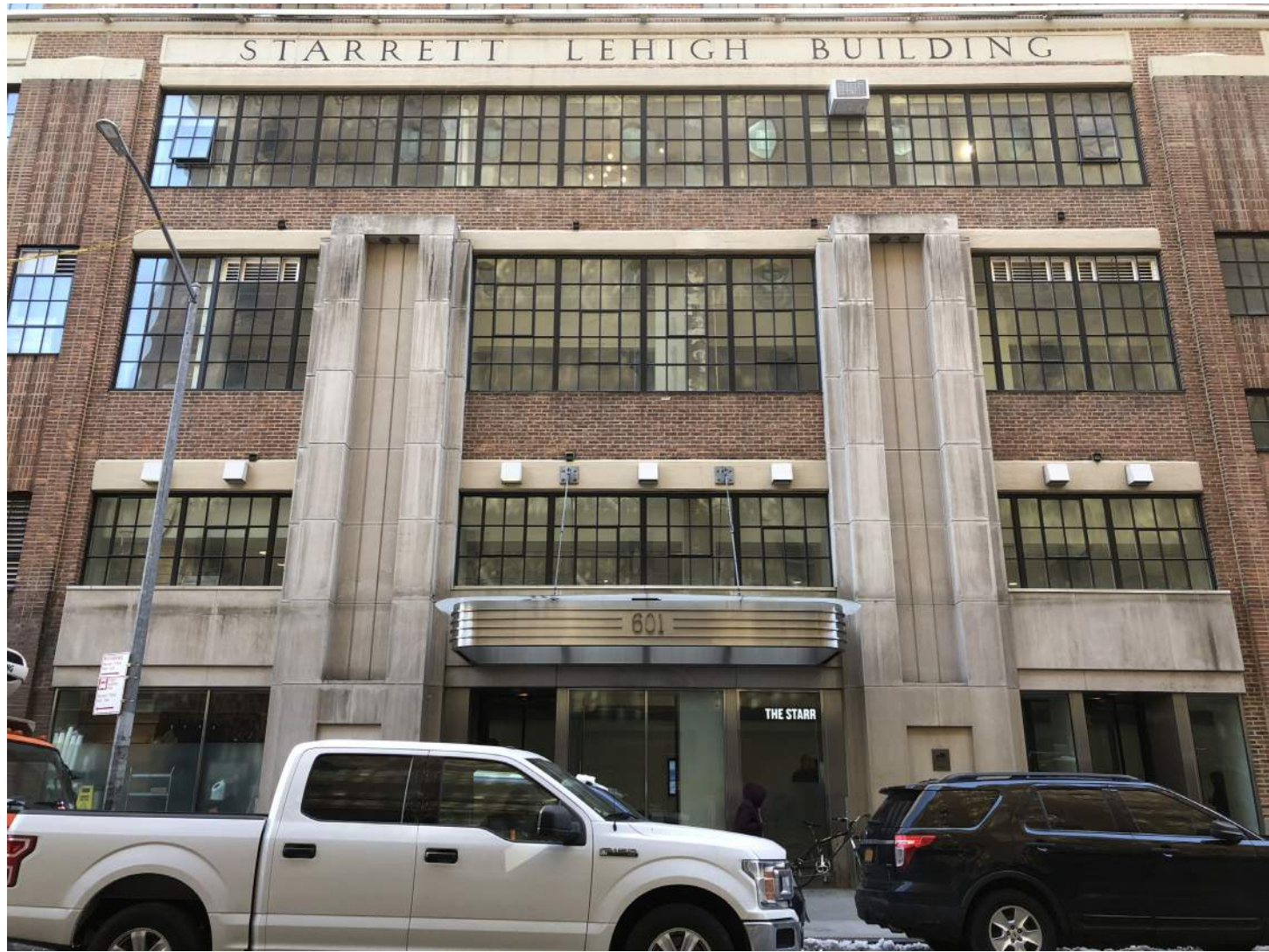
26th Street facade, frontal view of proposed work location
