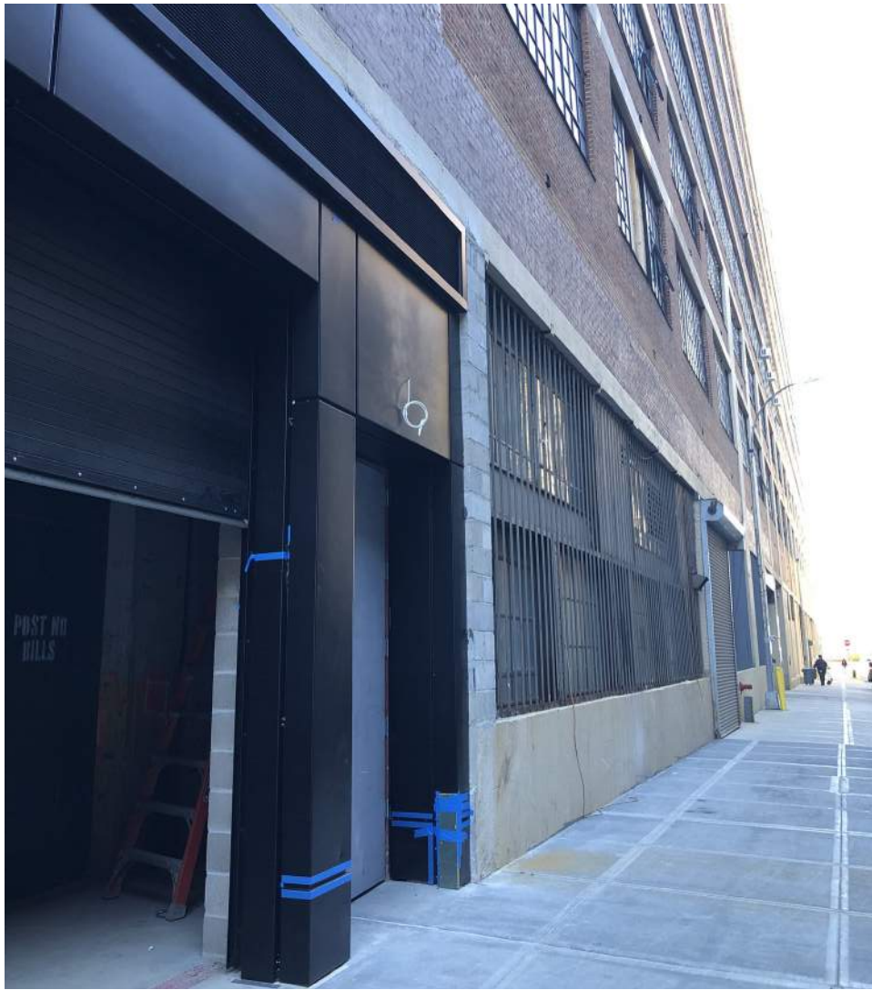
27th Street facade, view looking west of proposed work location
