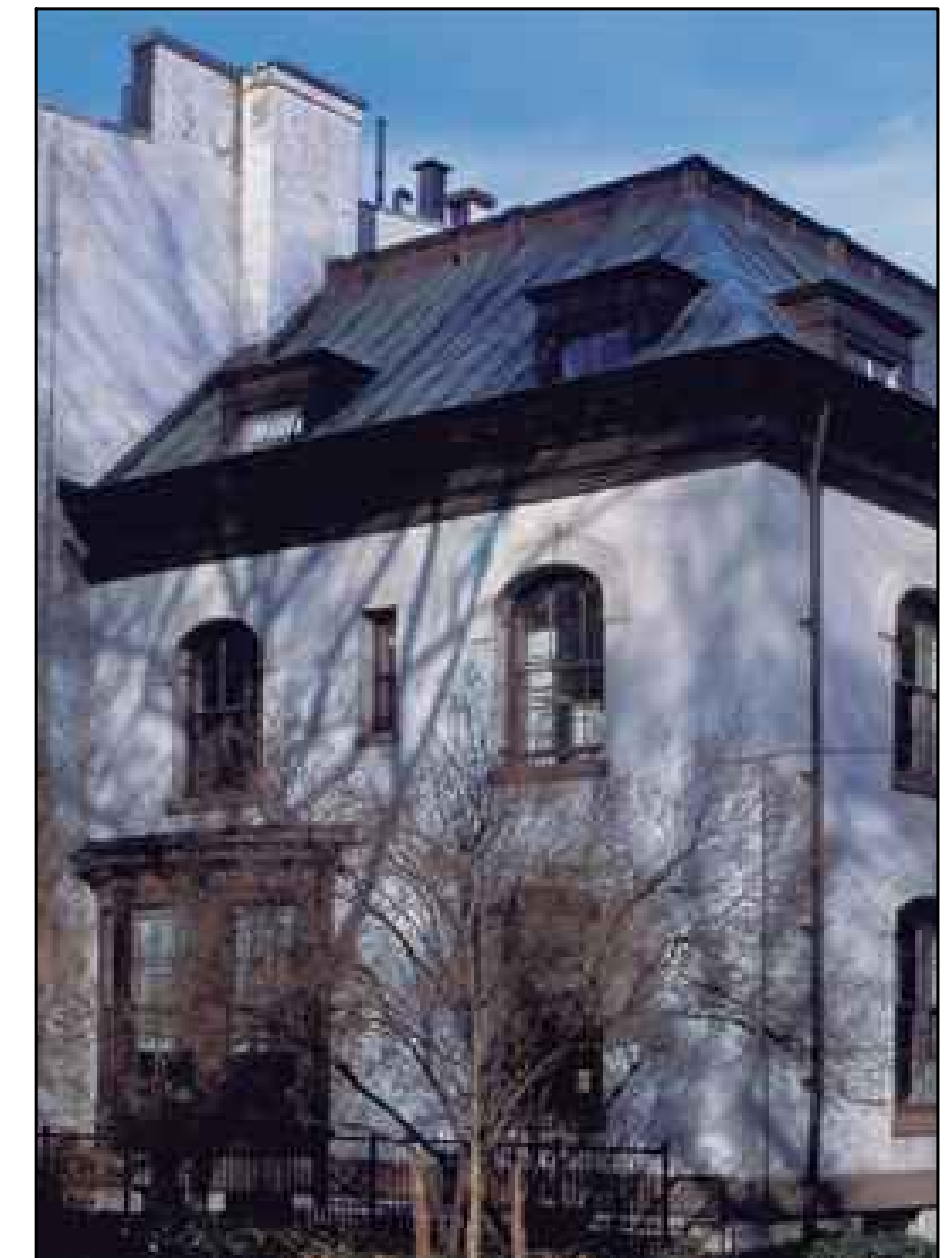
Standing Seam Roofing at Flagg's St. Marks Rectory
