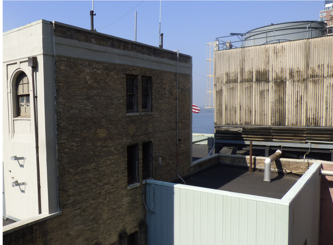
OVERALL VIEW OF ROOF, LOOKING SOUTHWEST
