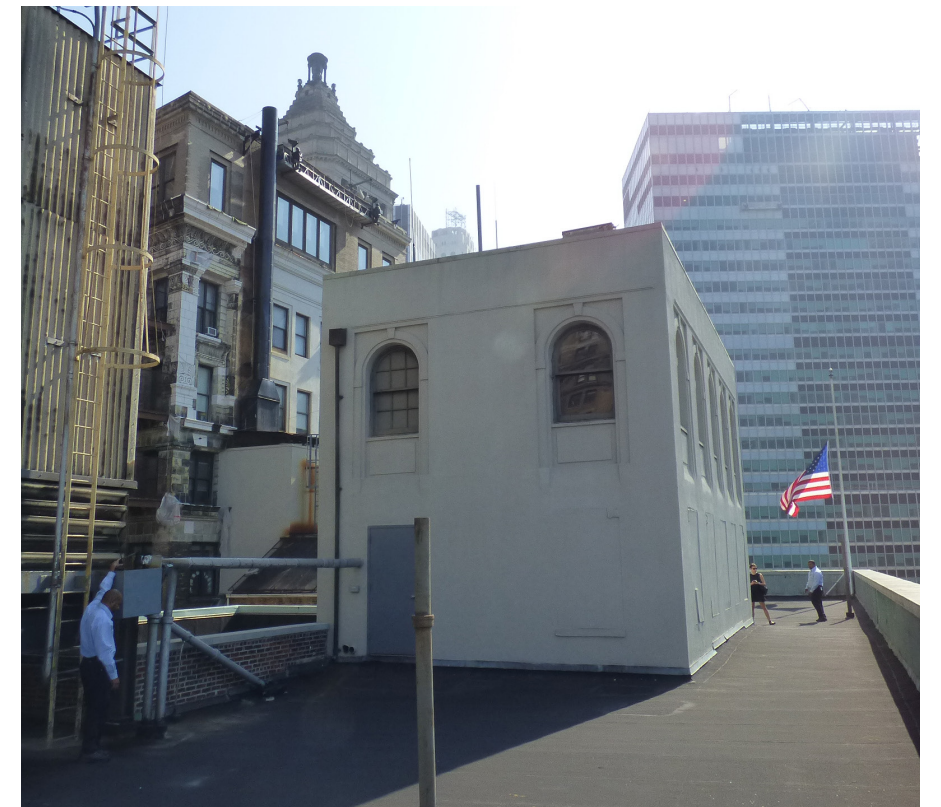
VIEW OF CENTRAL SERVICE PENTHOUSE, LOOKING EAST
