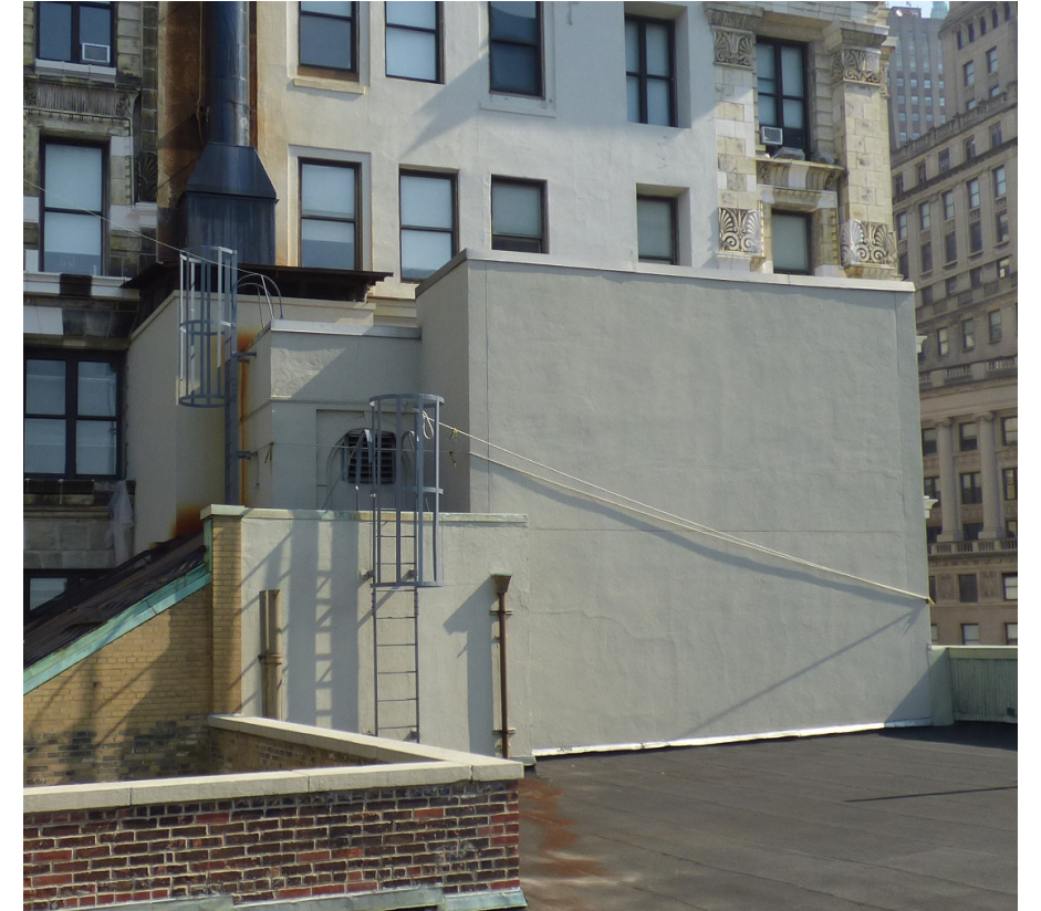
SOUTH ELEVATION OF EASTERN MACHINE ROOM BULKHEAD
