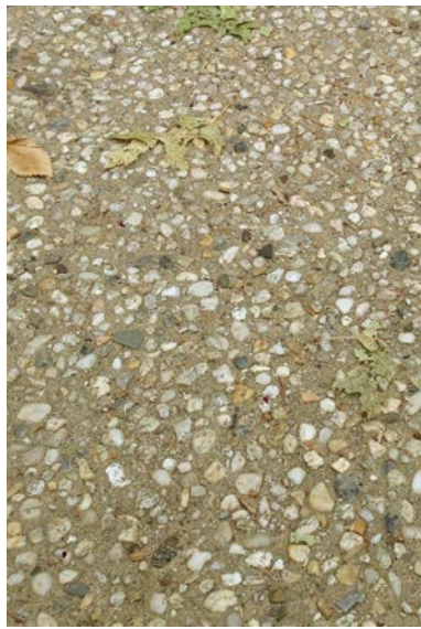
Exposed Aggregate Concrete Pavement
