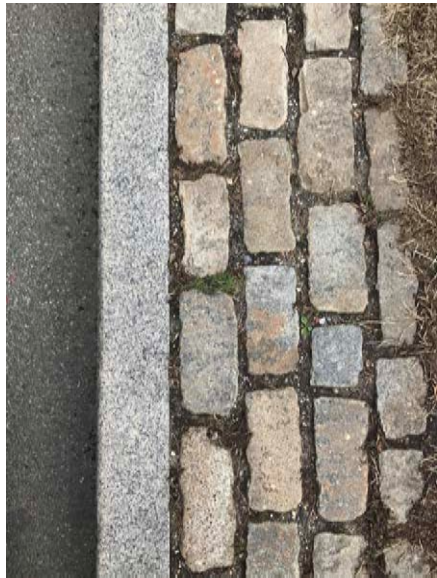
Granite Curb with Cobble left: Eastern Parkway, right: Ocean Parkway
