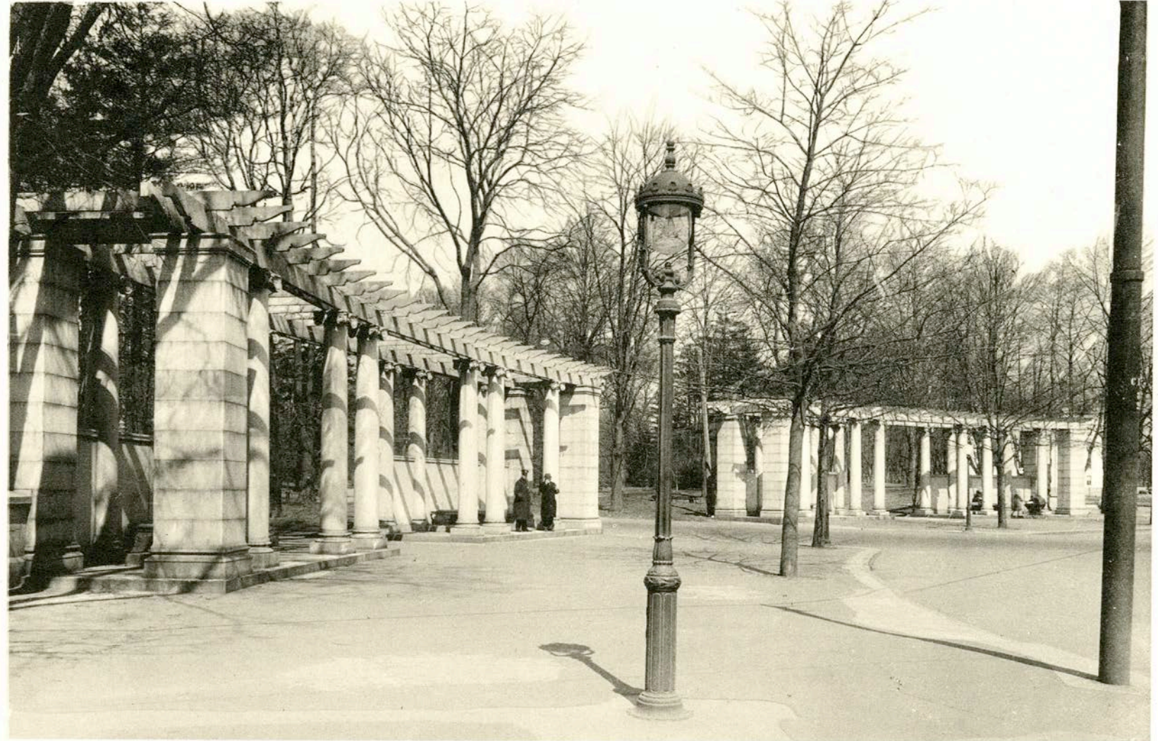
PERGOLA AT 15 TH ST. ENTRANCE.
