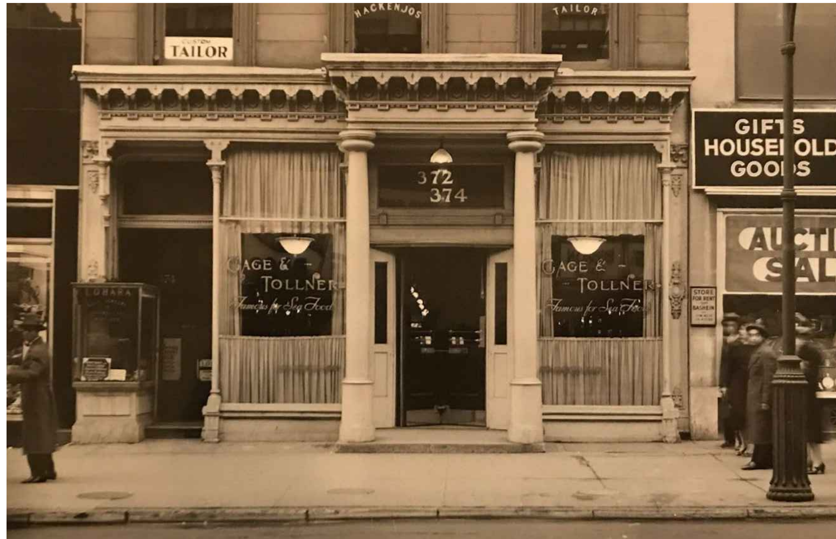
VIEW OF FRONT FACADE - 1950s
