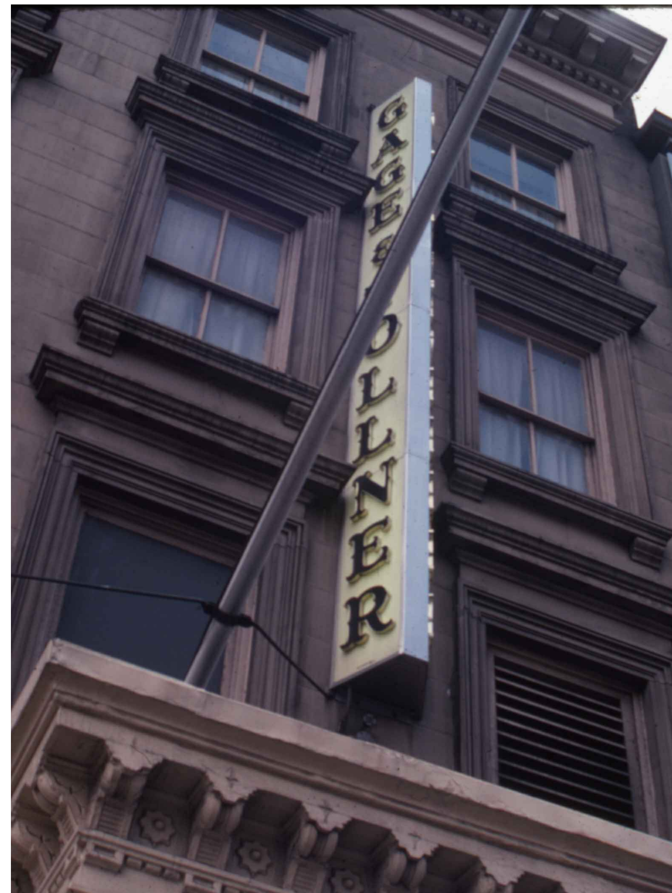
VIEW OF ILLUMINATED SIGN
