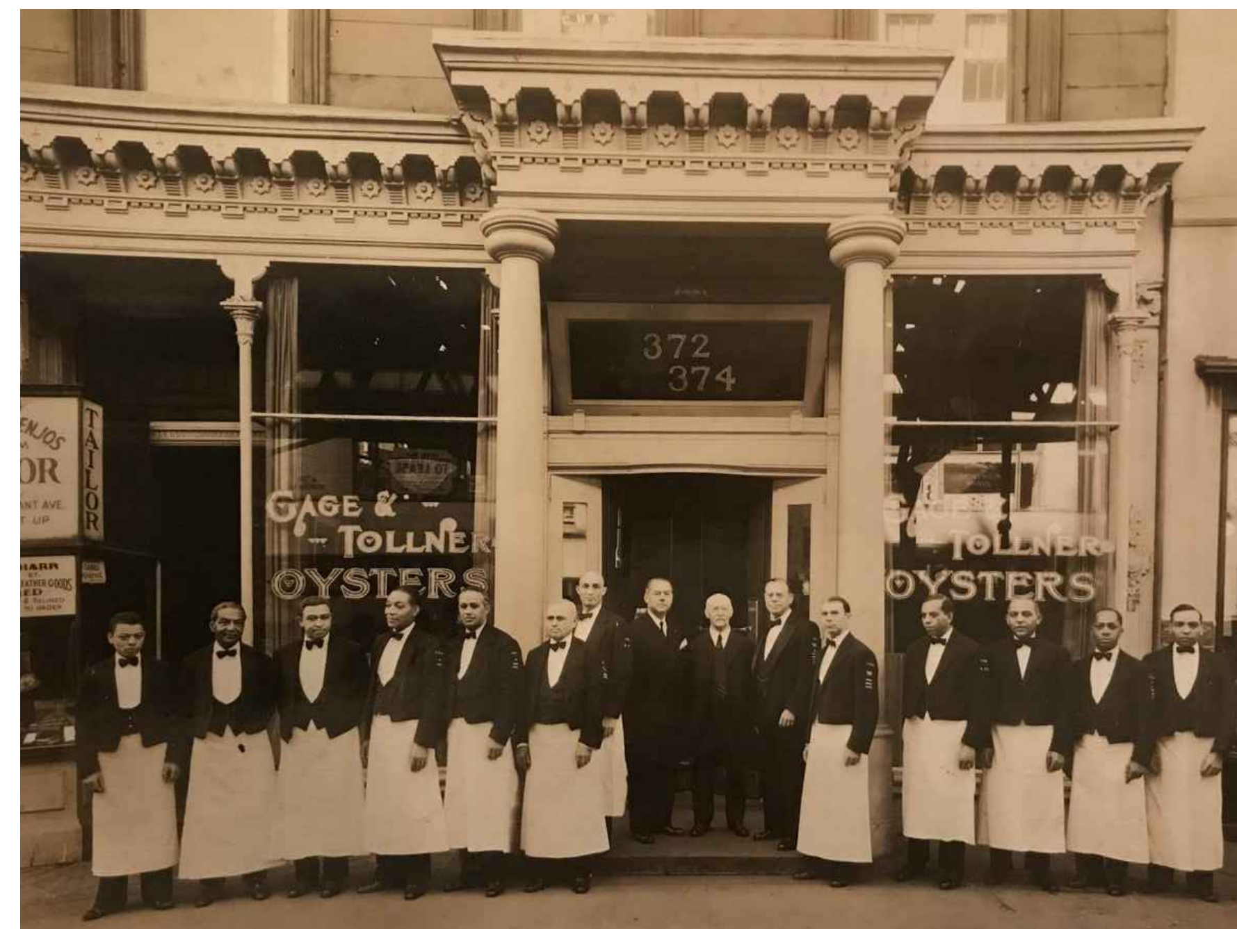
VIEW OF STAFF AT EXTERIOR - 1920s
