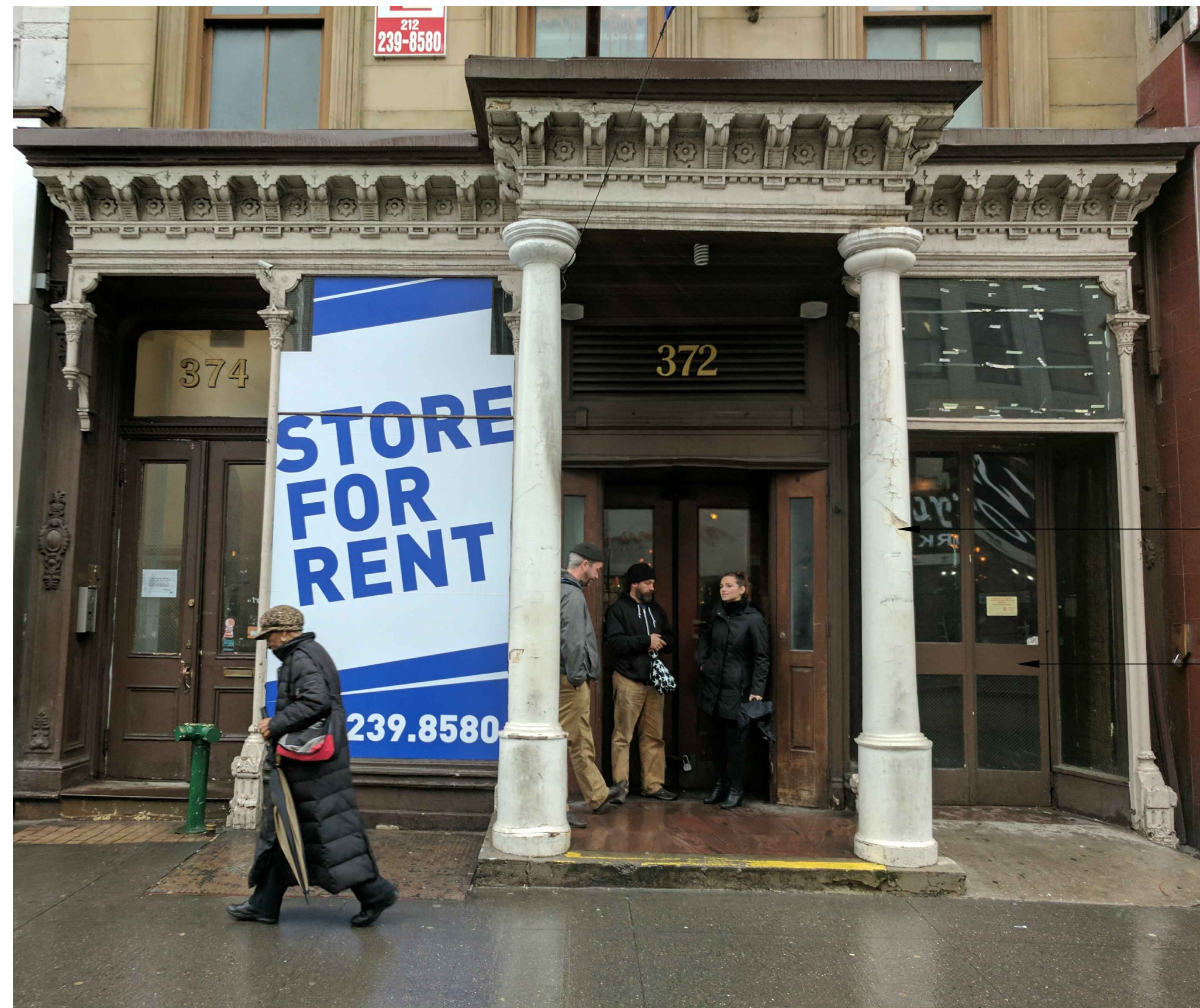
EXIST. VIEW OF LOWER FRONT FACADE
