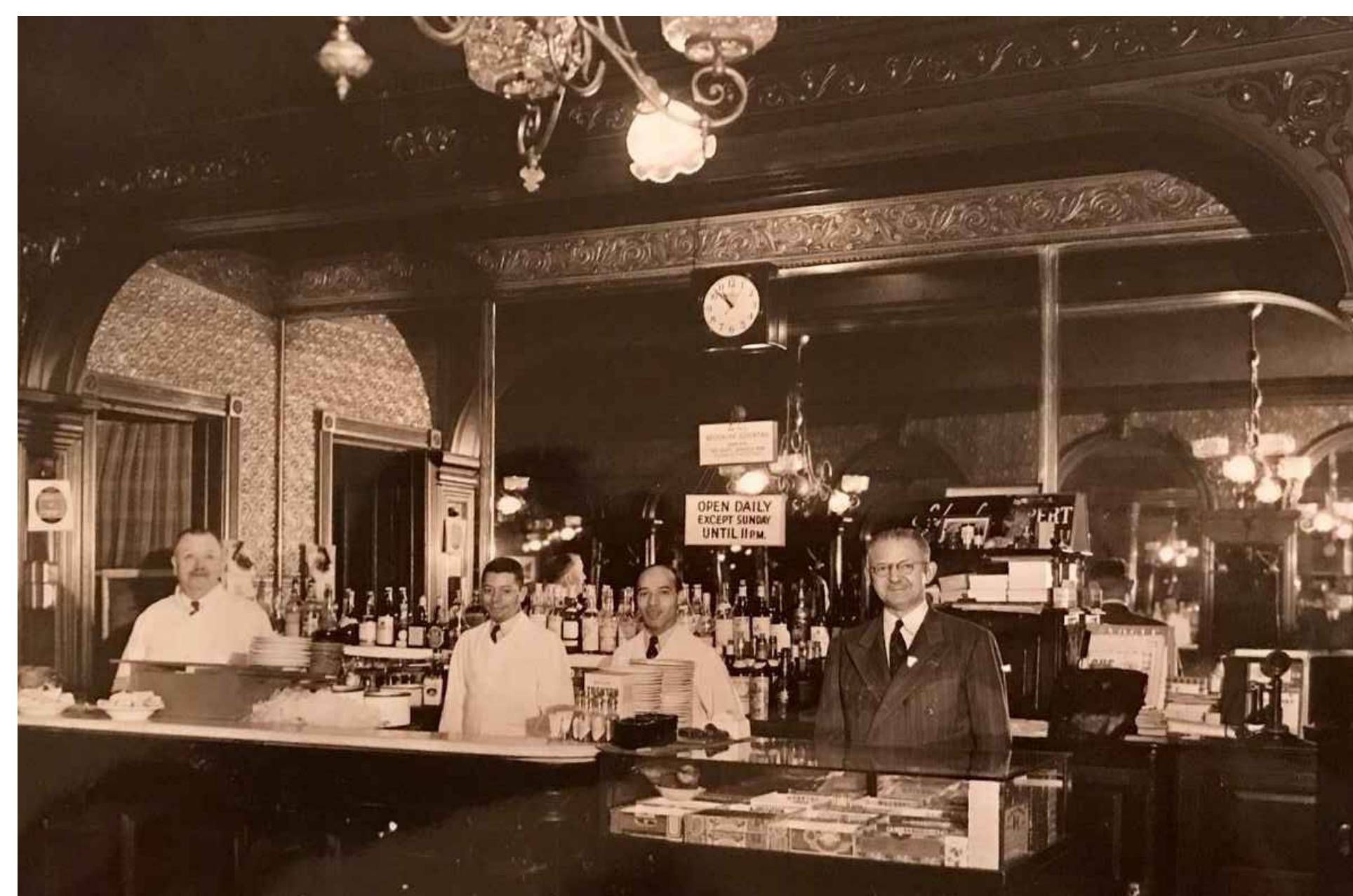
VIEW OF SERVICE BAR - 1939
