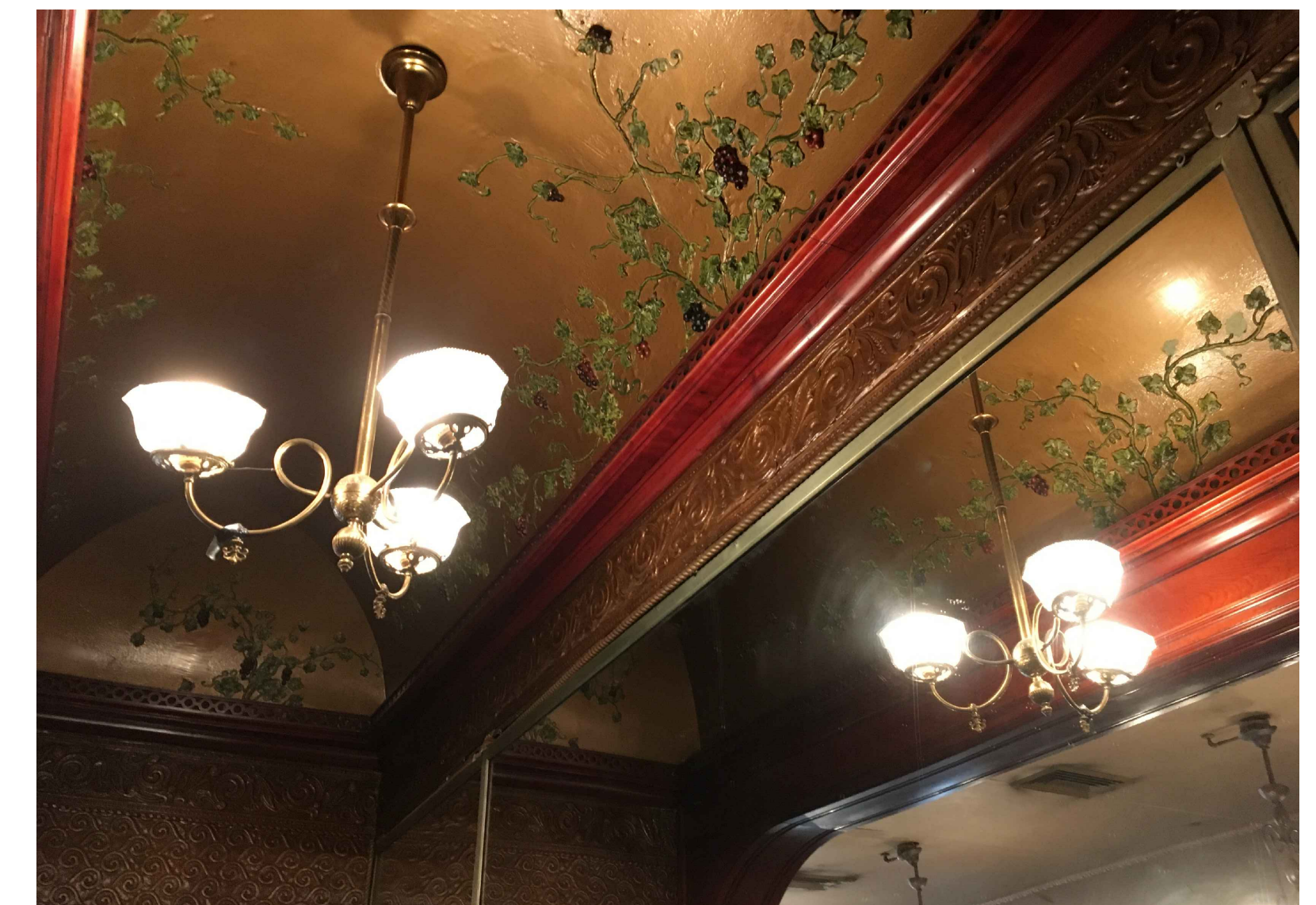
EXIST. VIEW OF CEILING AT SERVICE BAR
