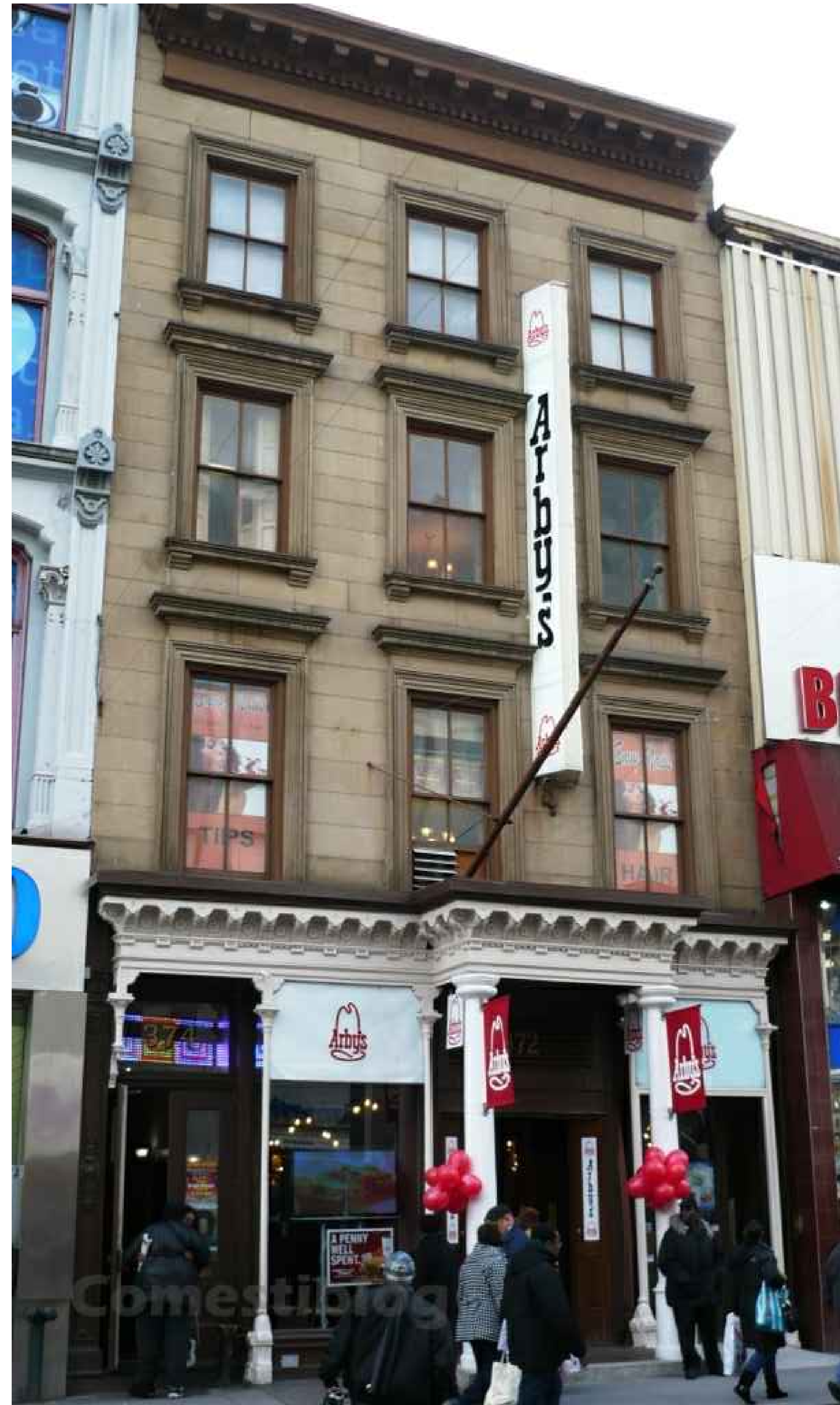
VIEW OF FRONT FACADE - "ARBY'S" ILLUMINATED SIGN", 2010
