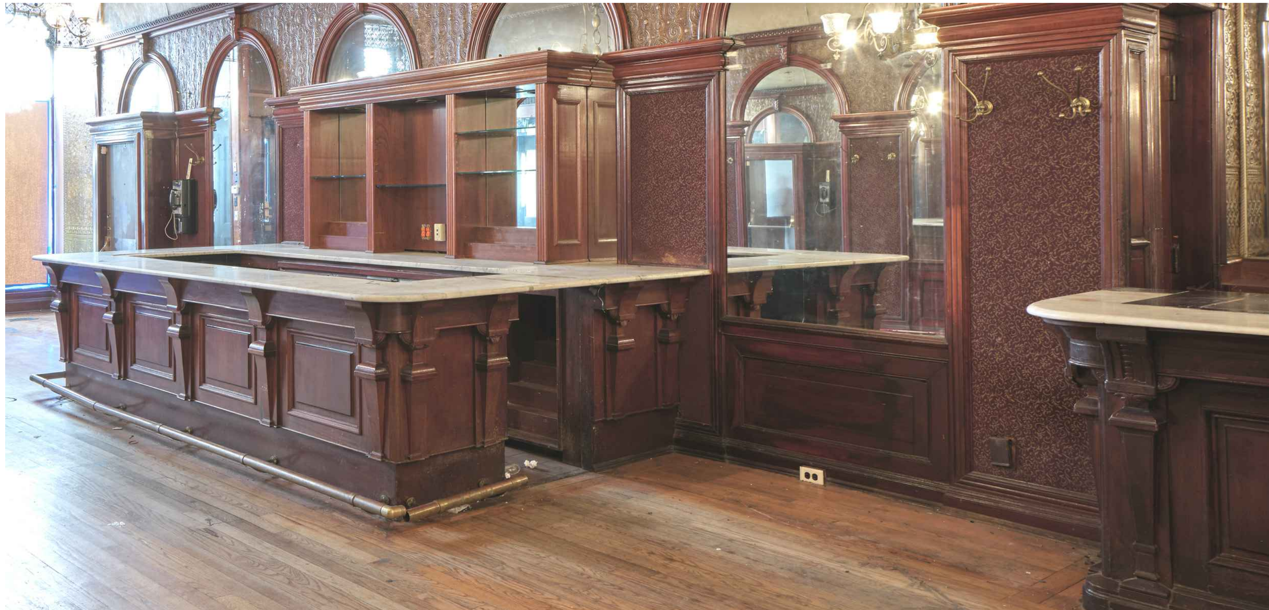
VIEW OF EXISTING BAR - INSTALLED IN 1999 UNDER CNE 96-0843
